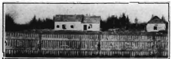
Trading Store and Warehouse, Cedar Lake
