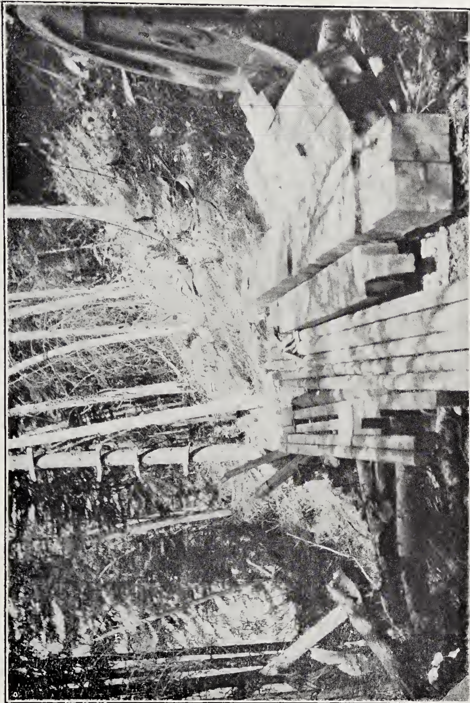
Oil boring machine in place, beyond Fort McKay. Latitude 56°3', longitude 111°3'. Timber cut in locality, spruce, 18 feet by 18 inches.
