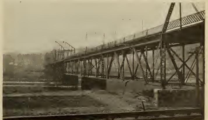
Figure No. 5.—Reno Traction Bridge Put Back Without Damage on to its Piers with the Removal of the Ice by the Thermit Treatment.
