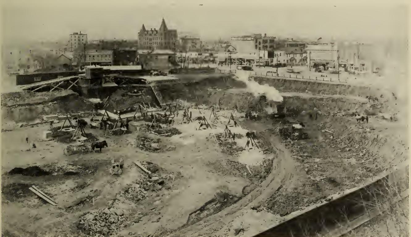
Figure No. 1.—Taking out General Excavation and Sinking Caissons on Hudson's Bay Building, Winnipeg, Man.
