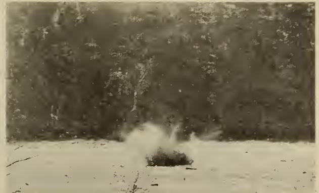
Figure No. 10.—Lowering Water Level. Shot No. 2.—Black Powder, 25 lbs., Thermit, 160 lbs.
