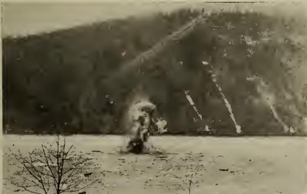
Figure No. 9.—Lowering Water Level. Shot No. 1.—Black Powder, 25 lbs., Thermit, 160 lbs.
