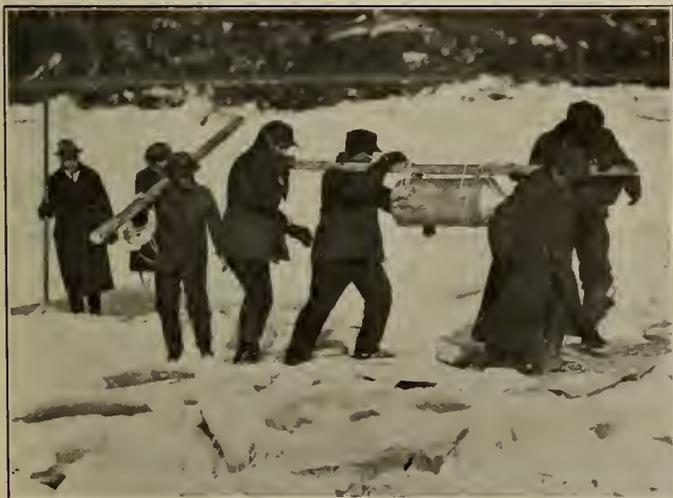
Figure No. 13.—Carrying Large Heat Unit out on the Ice.
