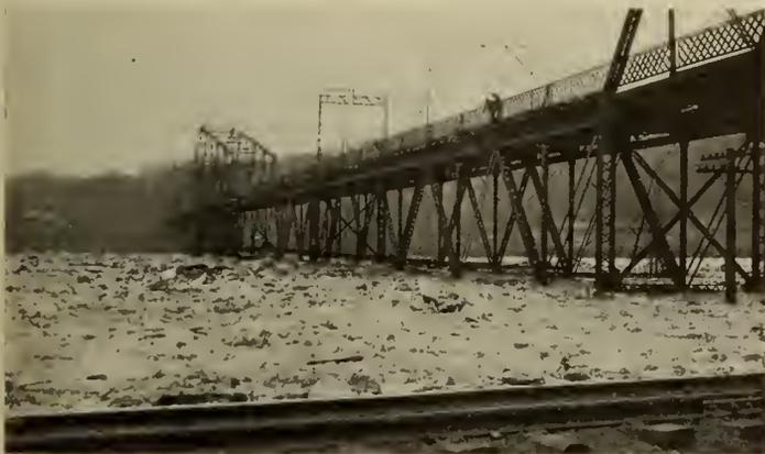
Figure No. 3.—Reno Traction Bridge at Oil City Lifted 18 inches above its Piers by the Ice.
