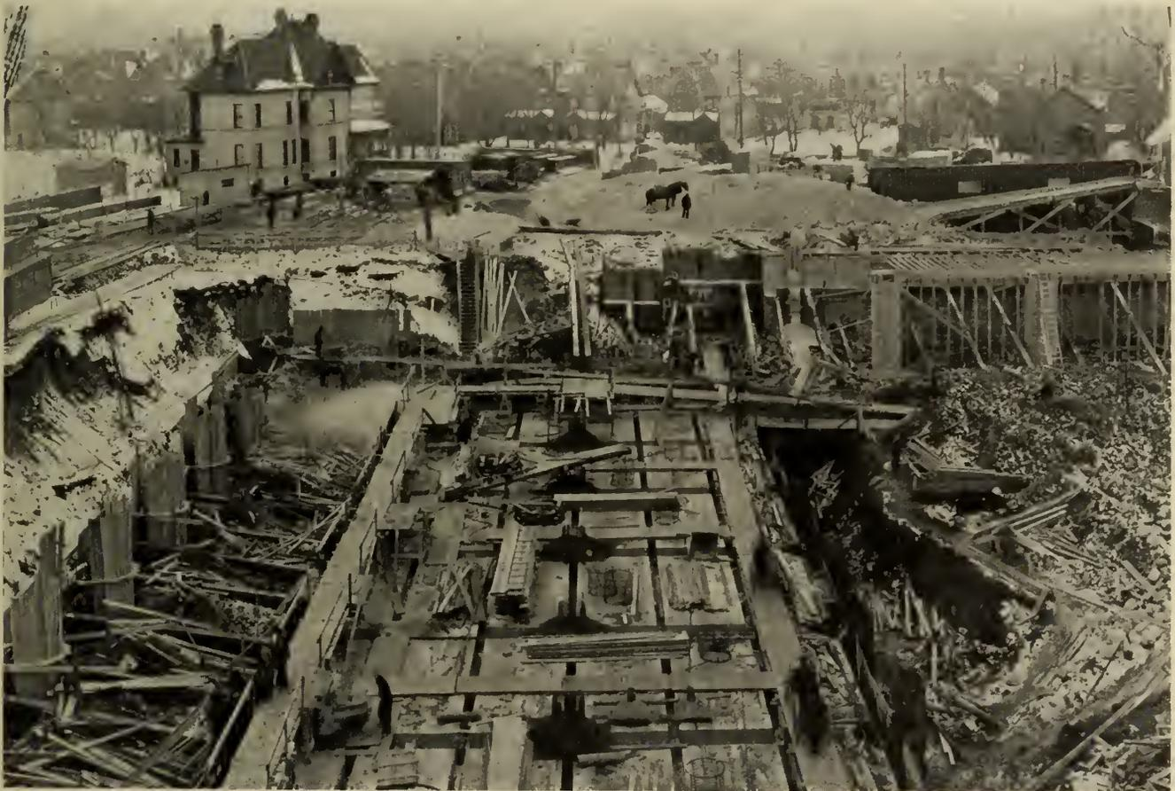
Figure No. 2.—Forming for Basement Floor over Sub-basement on Hudson's Bay Building, Winnipeg, Man.
