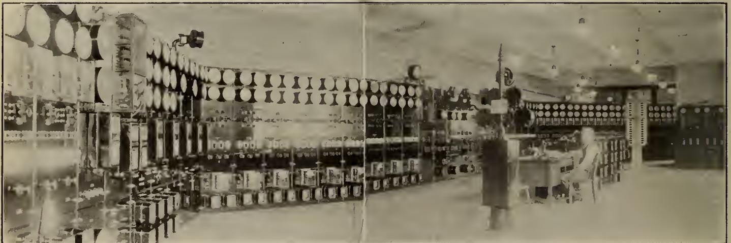
Figure No. 19.—Main Switchboard in Control Room.
