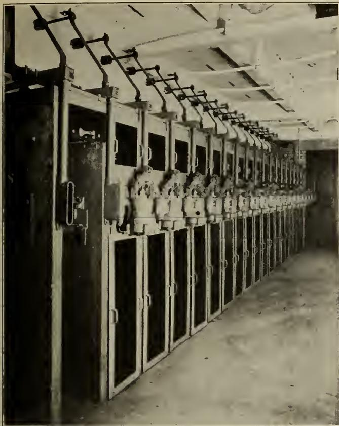
Figure No. 3.—Oil Circuit Breaker Cells.
