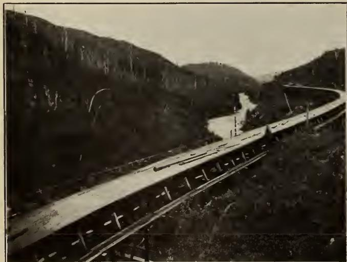
Figure No. 9.—Typical Scene on a Flume, Showing Guardian and Logs Going Down.
