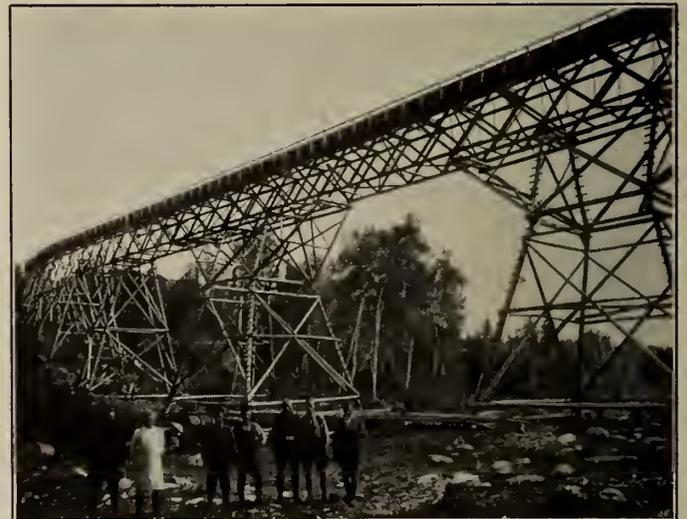
Figure No. 10.—A High Trestle Flume—Subgrade 80 feet above Sills.
