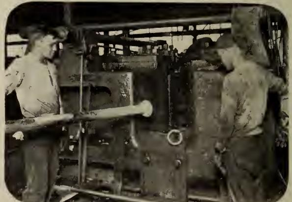
Figure No. 13.—Forging Machine Used in Forming Bearing Rings.
