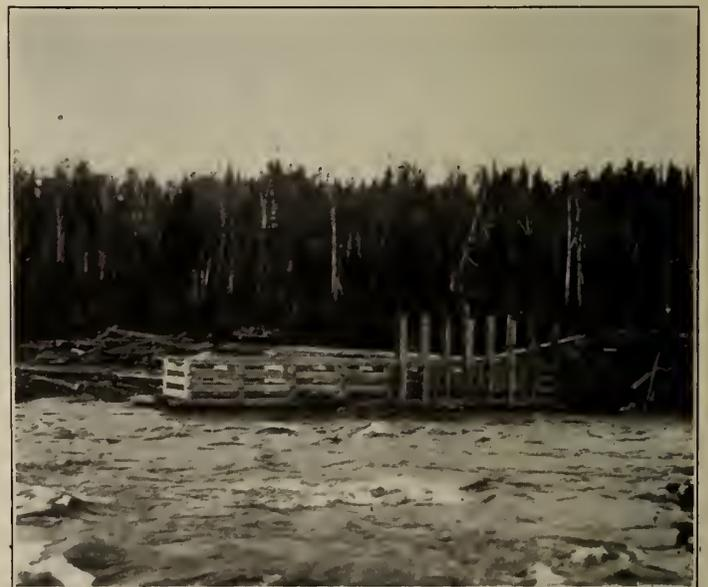
Figure No. 3.—A Wing Dam with Skeleton Made of Precast Reinforced Concrete Timbers.
