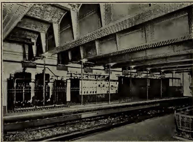
Figure No. 7.—Rectifier Installation, Mounted on Platform of Subway Station.
