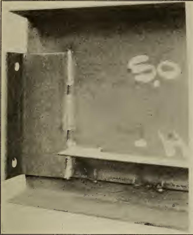
Figure No. 3—Method of Welding Flanges and Window Supports to Floor Beams.
