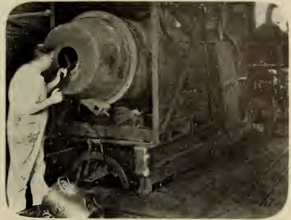
Figure No. 8.—Type of Furnace for Hardening Balls.
