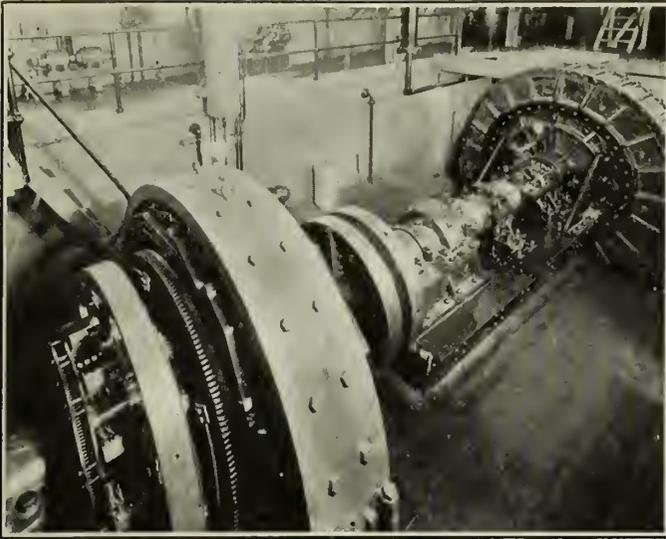
Fig. 3—Main Pump and Drive Motor.
