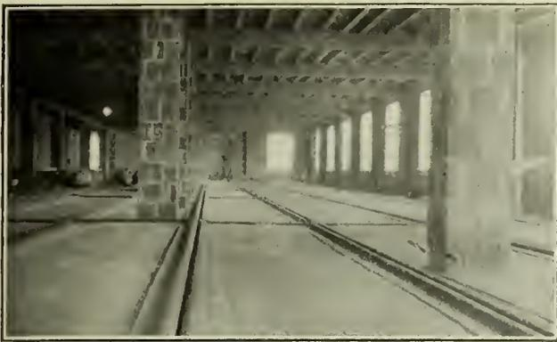
Fig. 5—Typical Under-floor Duct Layout.
