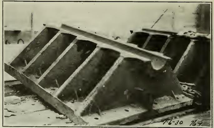
Fig. 10—Steel Castings for Hinges.
