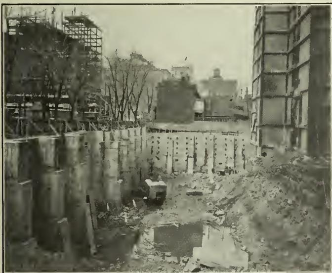
Fig. 3—West Side—Basement Walls designed as Retaining Walls.
