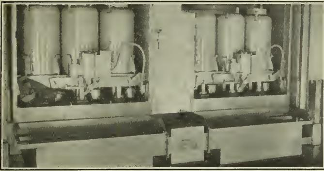
Fig. 15—Metal-clad Circuit Breakers.
