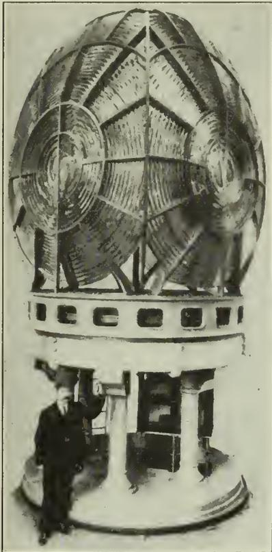
Fig. 7—Optical Apparatus of Lighthouse, Outside View.
