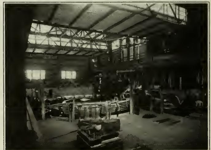
Fig. 7—Wire Bar Casting Wheel.
