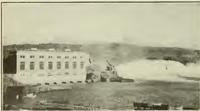
Fig. 12—View of Power House from Downstream Side. All River flow Passing over Spillwall.
