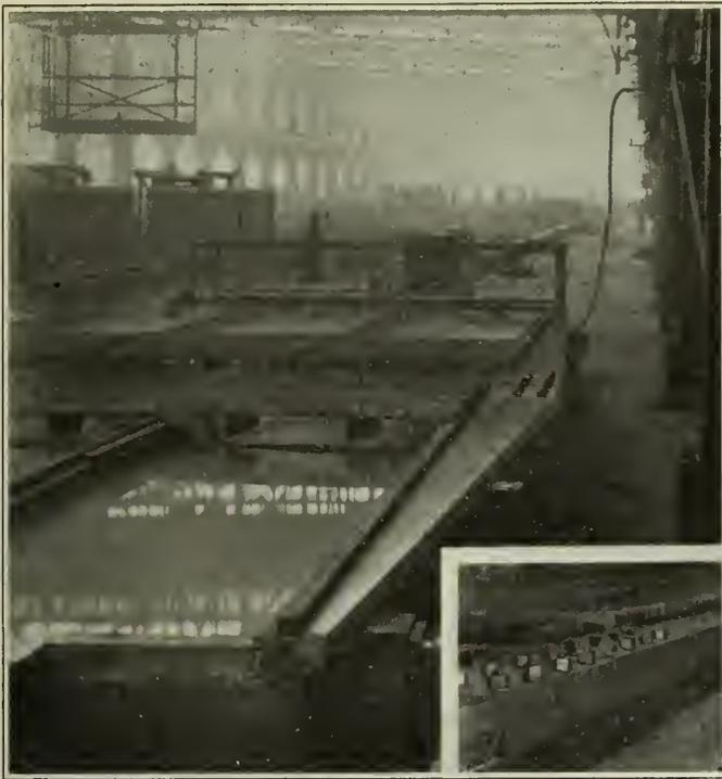
Fig. 8—General View of Tank House Showing Method of Splicing Bus Bar.
