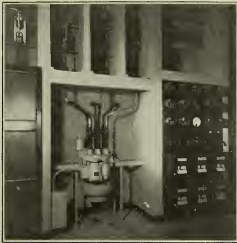
Fig. 1—Control Panel and B-16 Oil Circuit Breaker.
