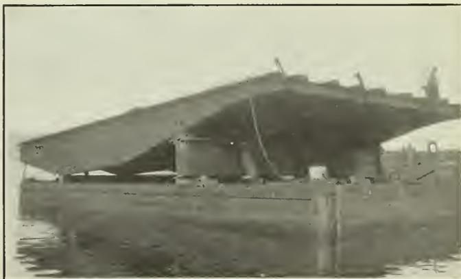
Fig. 22—Old Apron with Girder *B* being floated out.
