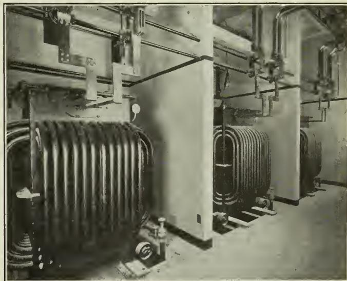
Fig. 2—Three 500 Kv.a. Power Transformer Banks 13,000 to 220 volts.
