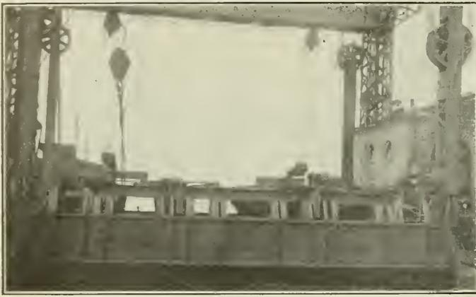
Fig. 23—Apron connected to Girder E. Note Shoes for connection of Intermediate Span Girders and Springers.
