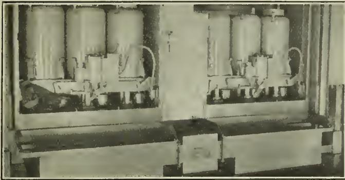
Fig. 15—Metal-clad Circuit Breakers.
