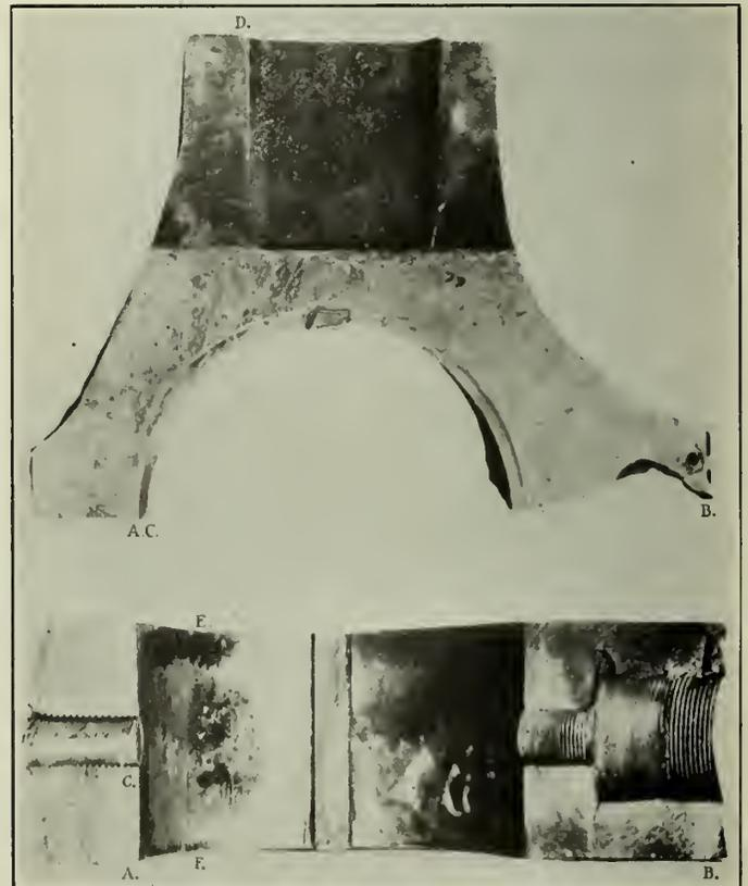
Fig. 12—Side and End View of Broken Leading Locomotive Side Rod.
