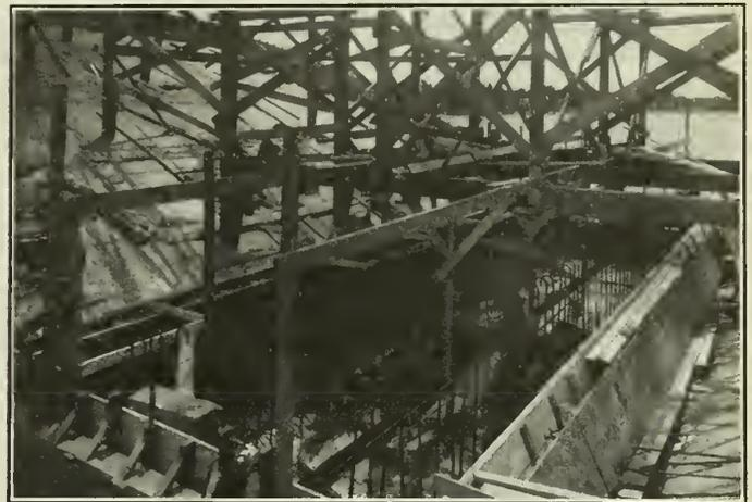
Fig. 8—Forms and Reinforcing, Pier No. 3.
