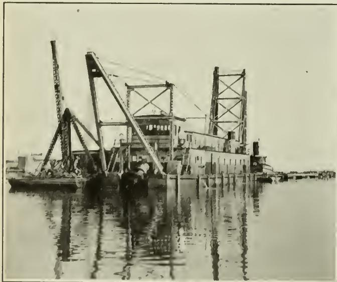
Fig. 7—Diesel Electric Suction Dredge "General Brock."
