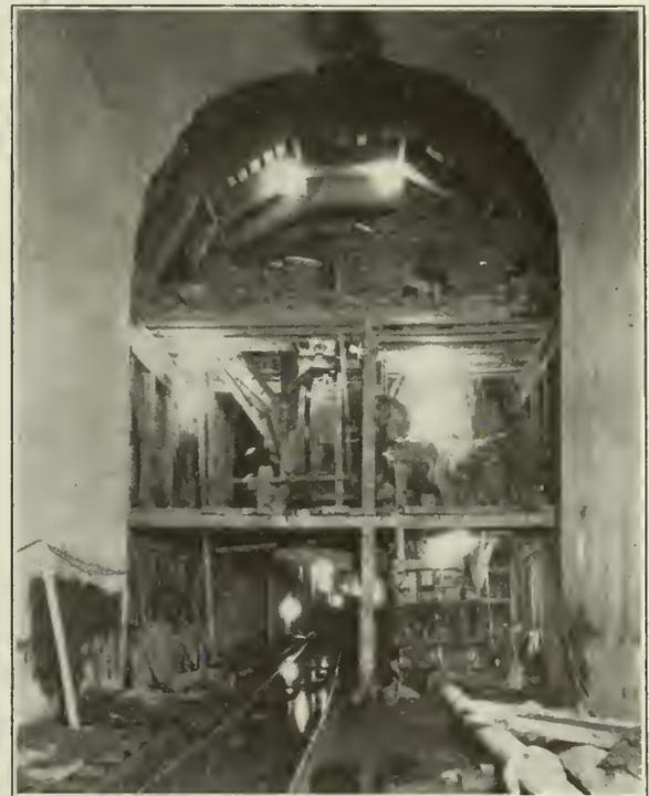
Fig. 9—Concrete Plant in Tunnel.
