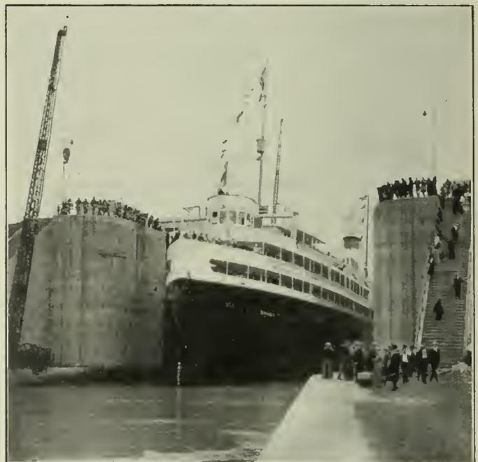
The S.S. Noronic of the Canadian Steamship Lines leaving lock No. 7 in the Welland Ship canal. The Noronic has a keel length of 362 feet, 52-foot beam and a gross tonnage of 6,905 tons. It will be noticed that the roof of the upper cabin is level with the top of the walls showing that the ship has a freeboard of about 51 feet.
