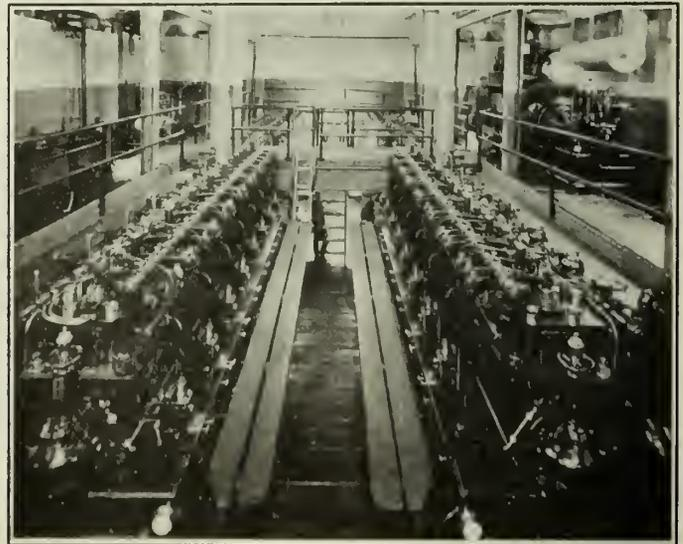
Fig. 2—Four 700 h.p., eight-cylinder Diesel Engines.
