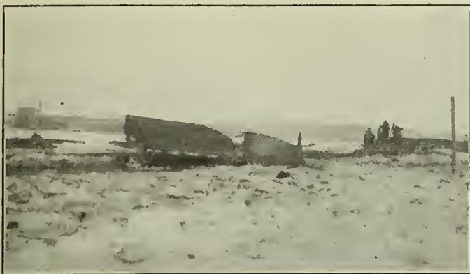
Fig. 5—Settlement—Rubble Mound Breakwater.
