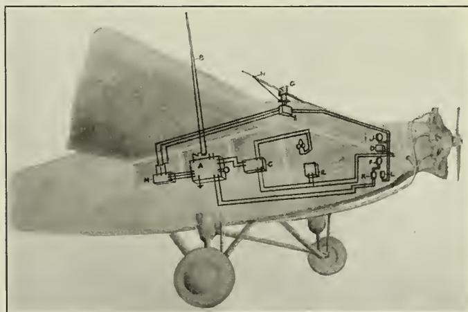
Fig. 4—Complete Aeroplane Radio Equipment for Blind Landing System.
