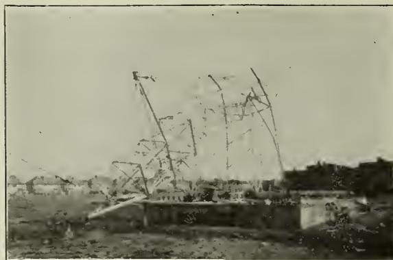
Fig. 12—Tower Test to Destruction.
