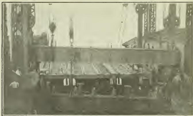
Fig. 21—Removing old Girder *E*. New 26-ton Girder suspended from Overhead Gantry.
