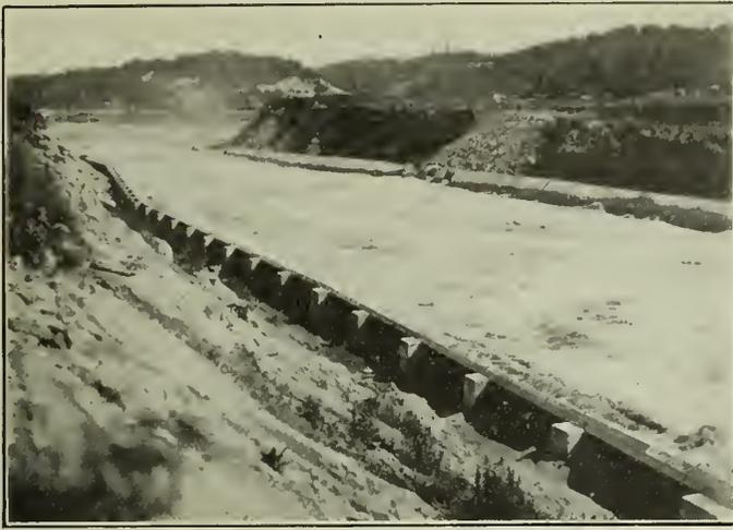
Fig. 2—Slab Displacement in Tailrace due to Gravel Slide.
