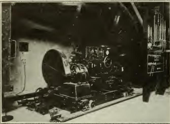
Fig. 9—Dynamometer and Air Duct as Arranged for Test of Tractor Type Air-Cooled Engine.
