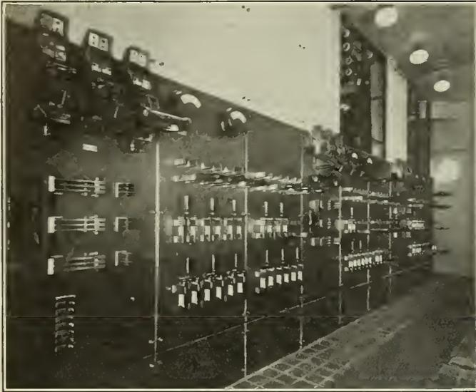
Fig. 3—Main Lighting Switchboard.
