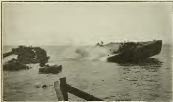
Fig. 7—Deck Dumping Scow, unloading.
