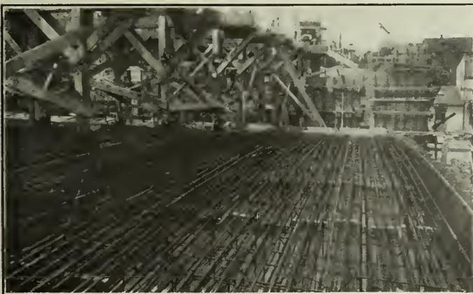
Fig. 7—Arch Reinforcing in Place.
