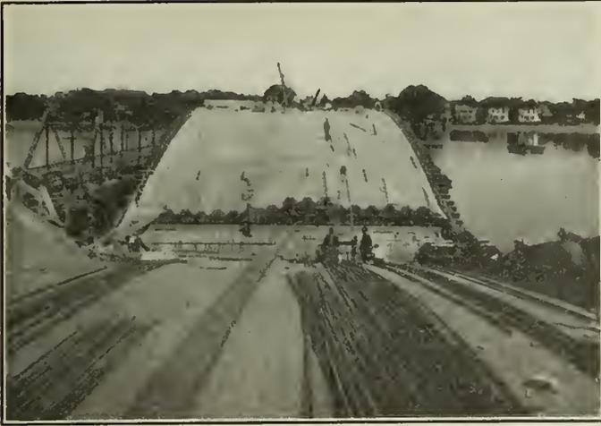
Fig. 6—Forms for Concrete Arches.
