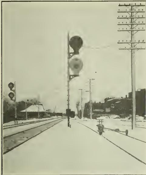
Fig. 3.—Disc Type Signal.
