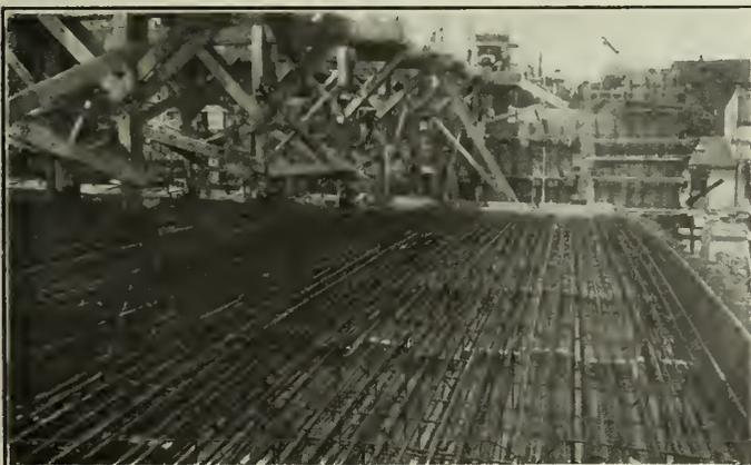
Fig. 7—Arch Reinforcing in Place.
