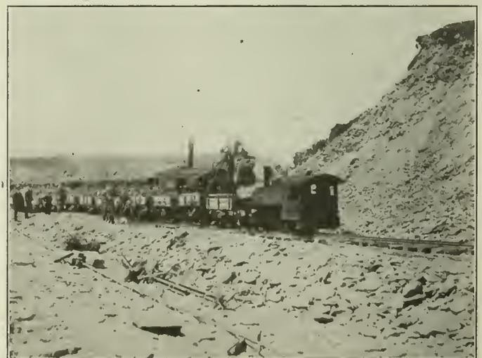
Fig. 13—Train loading old Beach Deposit for Core.
