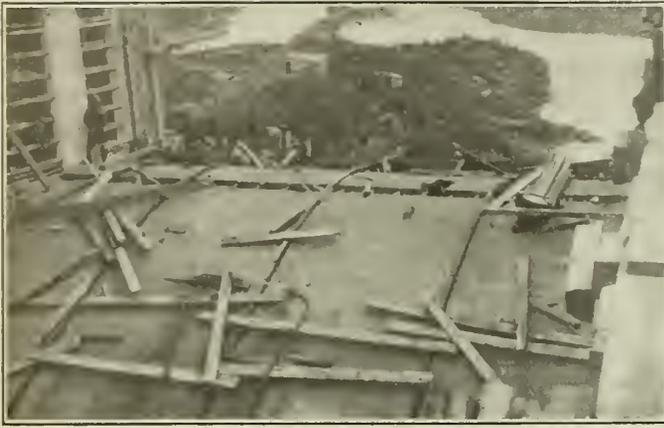
Fig. 6—Rollway Crest finished by Screeding.
