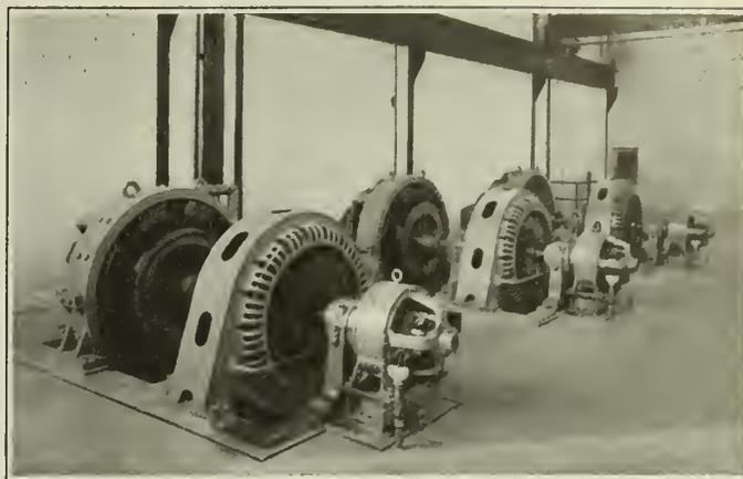
Fig. 13—Motor Generator Sets Supplying Current to Refining Circuit.
