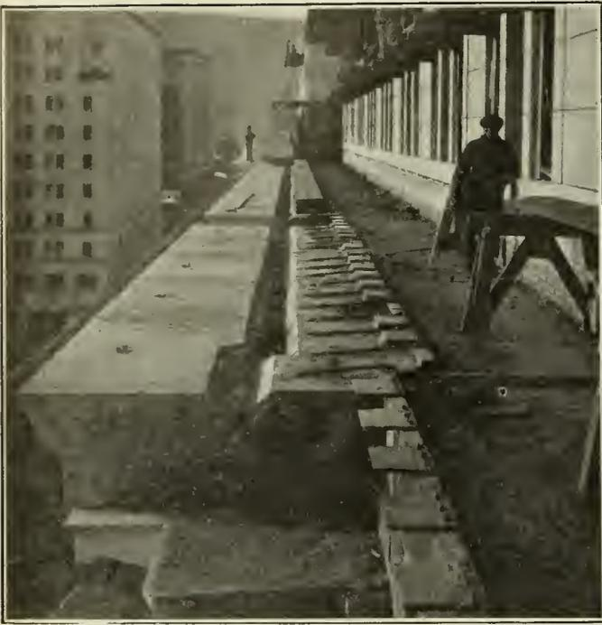
Fig. 14—Method of Anchoring Top Cornice.
