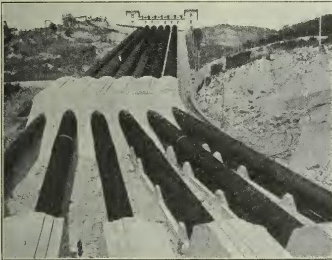
is collected by means of a large dam and forebay, whence it passes through a tunnel to a surge tank, thence through the penstocks to the power house.
