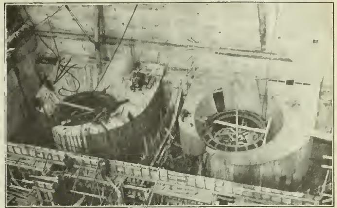
Fig. 11—Power House Substructure showing Forms for Concrete Spiral Scroll Case.
