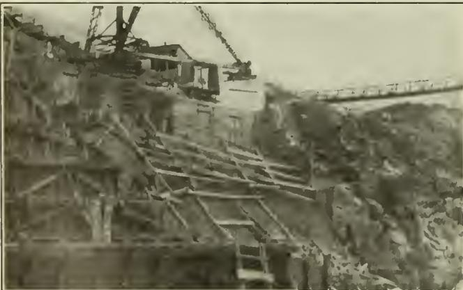
Fig. 7—Method of Setting Screeds on Warped Surface of Bucket.
