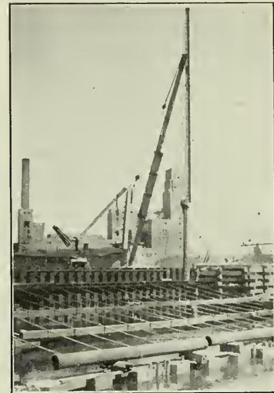
Fig. 5—Interlocking Last Sheet Pile. Length of Pile 60 feet.
