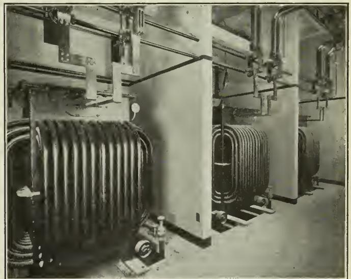
Fig. 2—Three 500 Kv.a. Power Transformer Banks 13,000 to 220 volts.
