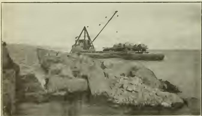
Fig. 8—Rubble Mound Breakwater as Constructed.
