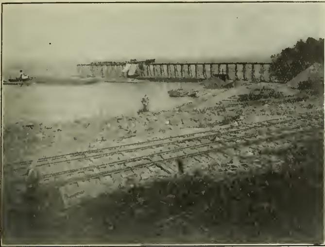
Fig. 14—Loading Scows from train by chute.
