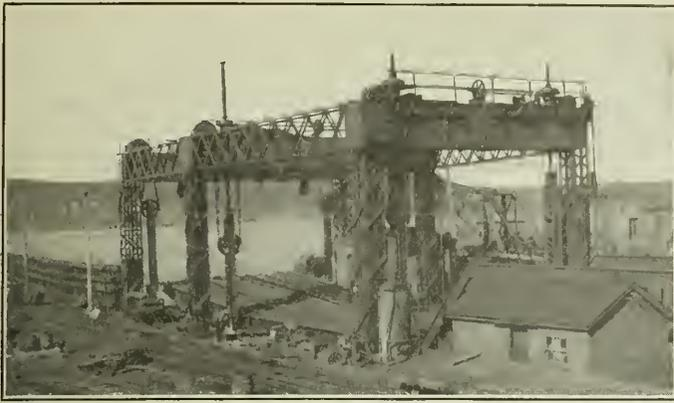
Fig. 11—Point Tupper Landing—Showing Apron and Intermediate Span.
