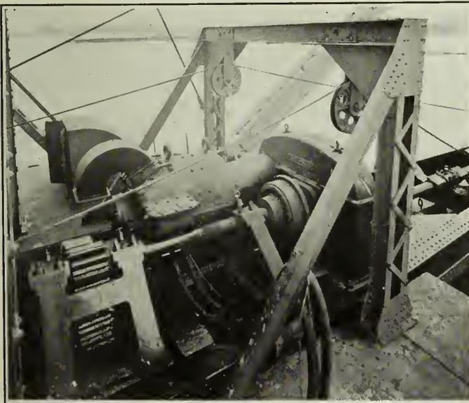
Fig. 4—Cutter Shaft Drive.
