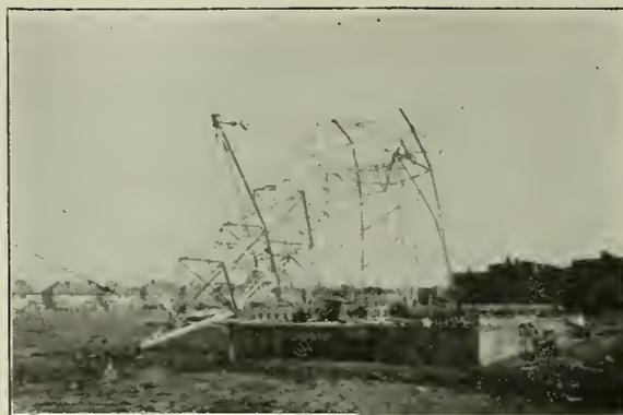
Fig. 12—Tower Test to Destruction.
