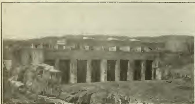
Fig. 11—General View of Forebay and Power House Headworks. Diversion Channel in left Foreground.
