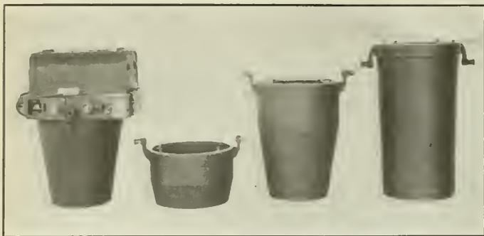
Fig. 5—K.3 Camera with 8-inch, 12-inch and 20-inch Cones.
