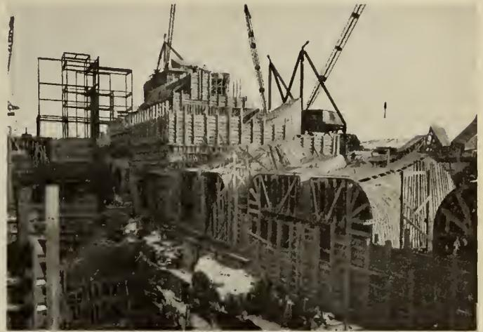
Fig. 5—Building Concrete Forms on Section of Power House.
