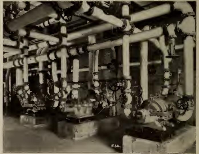
Fig. 5—Boiler Feed Water Pumps and Piping.
