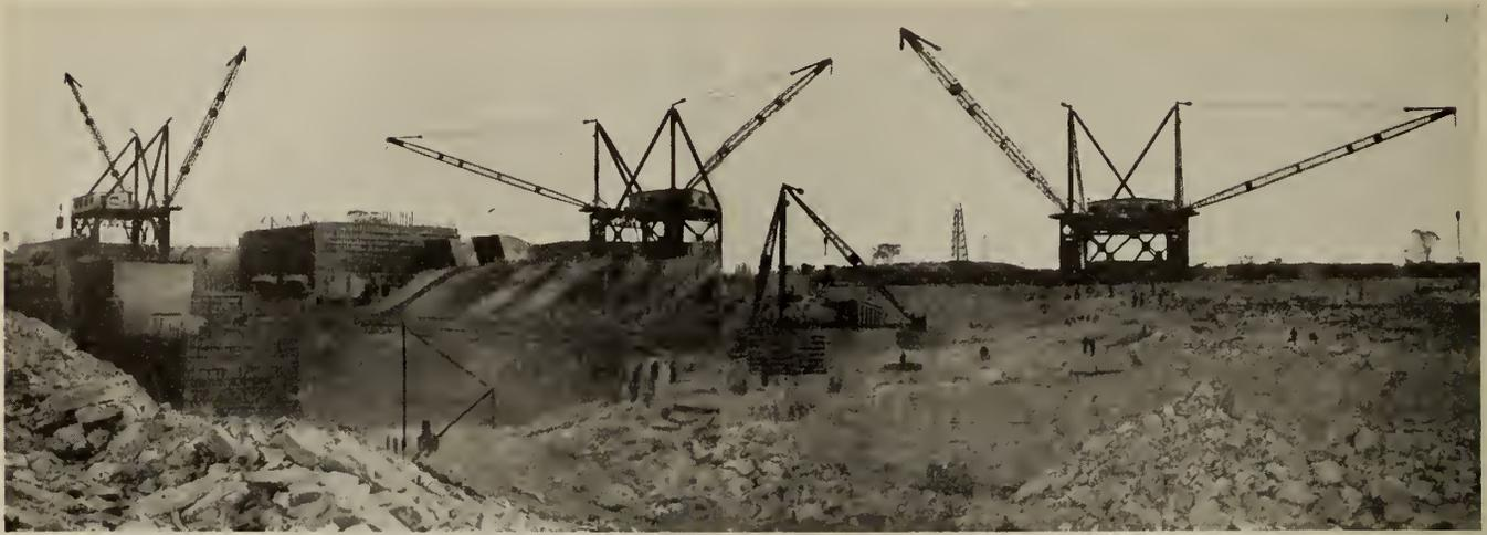
Fig. 3—Excavating for Power House, November 10th, 1930.
