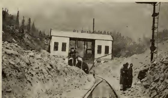
Fig. 3—Fan House West Portal—One Track Cleared for Traffic.
