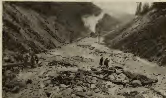
Fig. 2—View from West Portal—Debris 17 to 18 feet Above Top of Rail.
