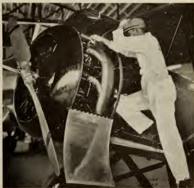
Fig. 3—Accessibility Obtained with Hinged Sections in N.A.C.A. Cowl.
