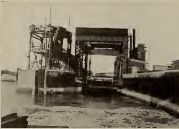
Fig. 6—Cape Tormentine Ferry Terminal Showing Inclined Bridge for Automobiles.
