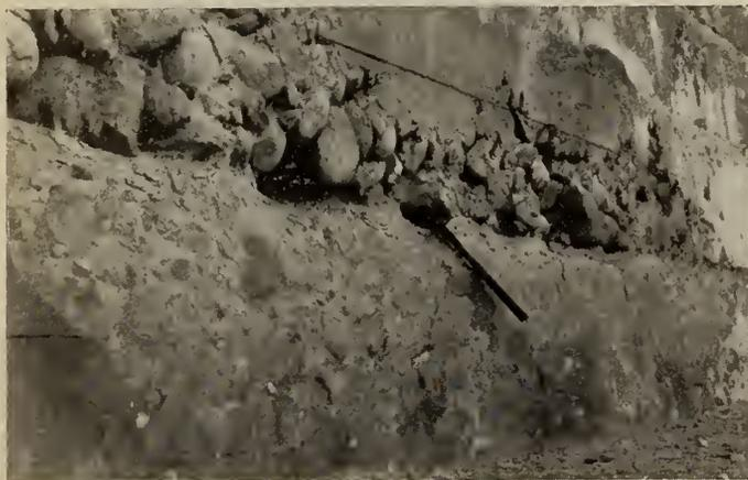
Fig. 7—Portion of Dam Showing Segregation of Constituents and Consequent Disintegration.
