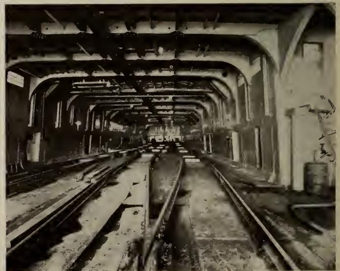
Fig. 9—Charlottetown—View of Car Deck showing Three Tracks.
