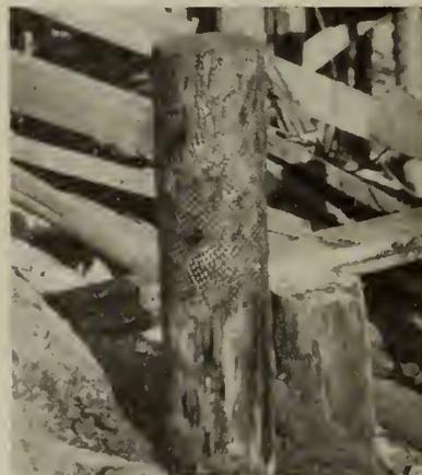
Fig. 4—Pile Incised before Field Treatment.
