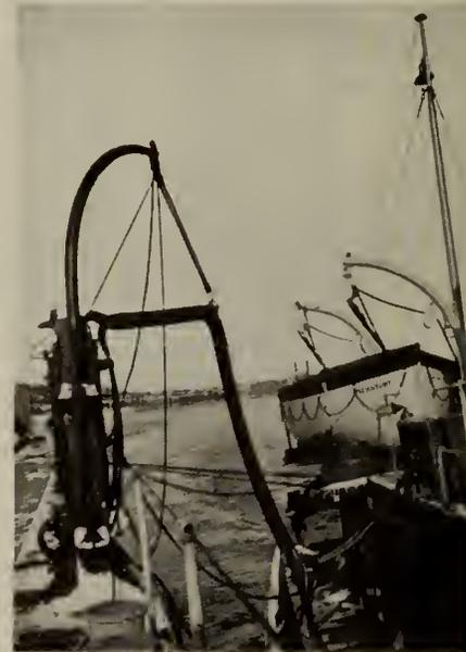
Fig. 8—Electric Connections Between Tug and Float.
