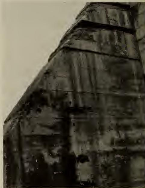
Fig. 8—Disintegration of Concrete in Buttress of Dam Due to Wet Consistency and Segregation.
