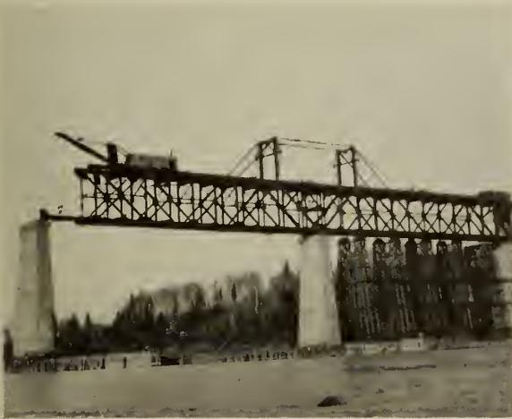
Fig. 10—Superstructure Under Erection, October, 1929.
