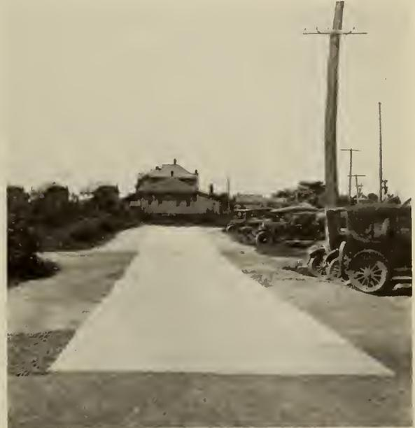
Fig. 1—Experimental Road Opened to Heavy Traffic in Twenty-four Hours, Pointe Anne, September, 1925.
