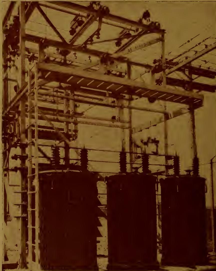
The above photograph shows three Moloney transformers installed in substation for operating bridges 13 and 14, Welland Ship Canal.
