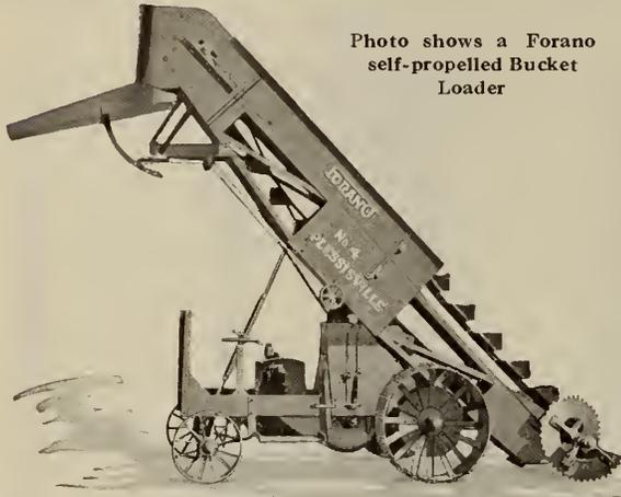
Photo shows a Forano self-propelled Bucket Loader
