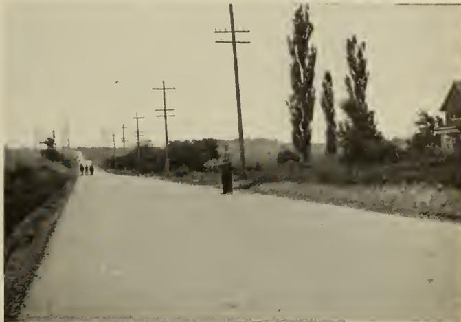
Fig. 2—A Tar Penetration Road, Constructed 1932.
