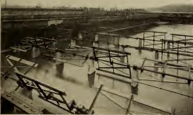
Fig. 2—Mechanical Conditioning Unit Located at one End of Settling Basin.
