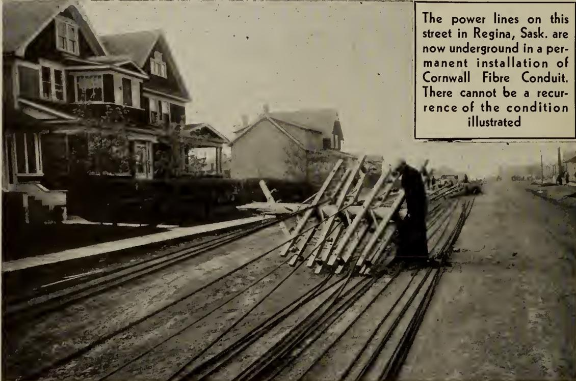
The power lines on this street in Regina, Sask. are now underground in a permanent installation of Cornwall Fibre Conduit. There cannot be a recurrence of the condition illustrated
