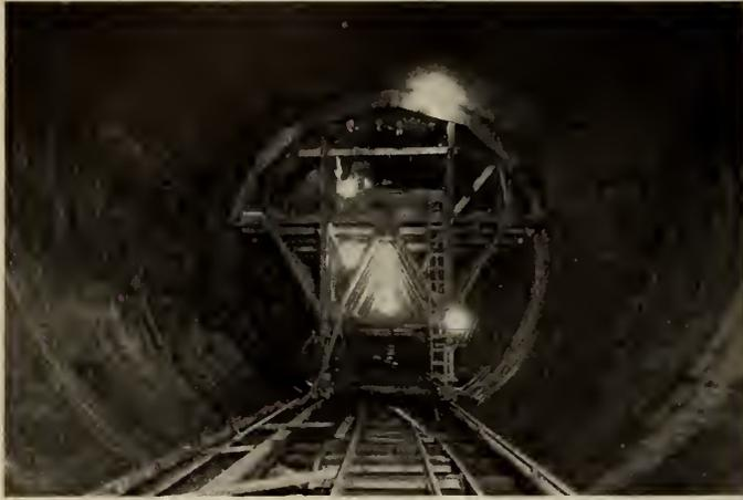
Fig. 7—Wall and Arch Forms Showing Arch Section.
