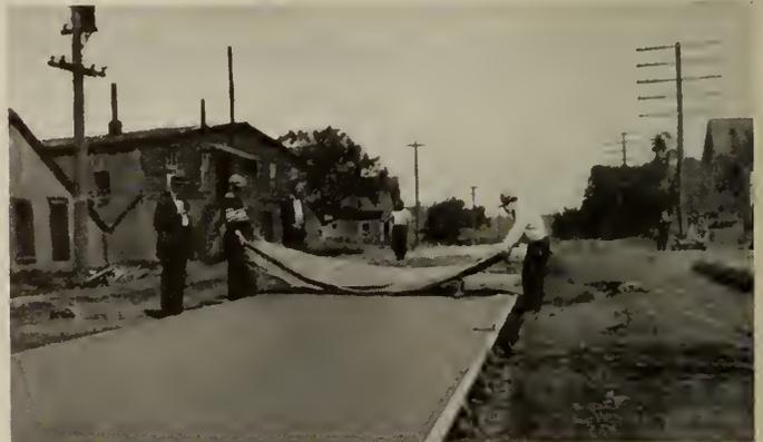
Fig. 3—Curing—covering with Burlap and Spraying.
