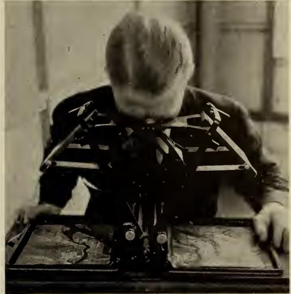
Fig. 9—Stereoscope with Grids for Accurate Contour Work.
