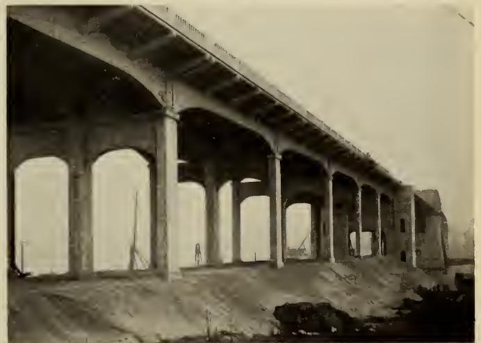
Fig. 4—Completed Railway Fill and Bents of South Viaduct.
