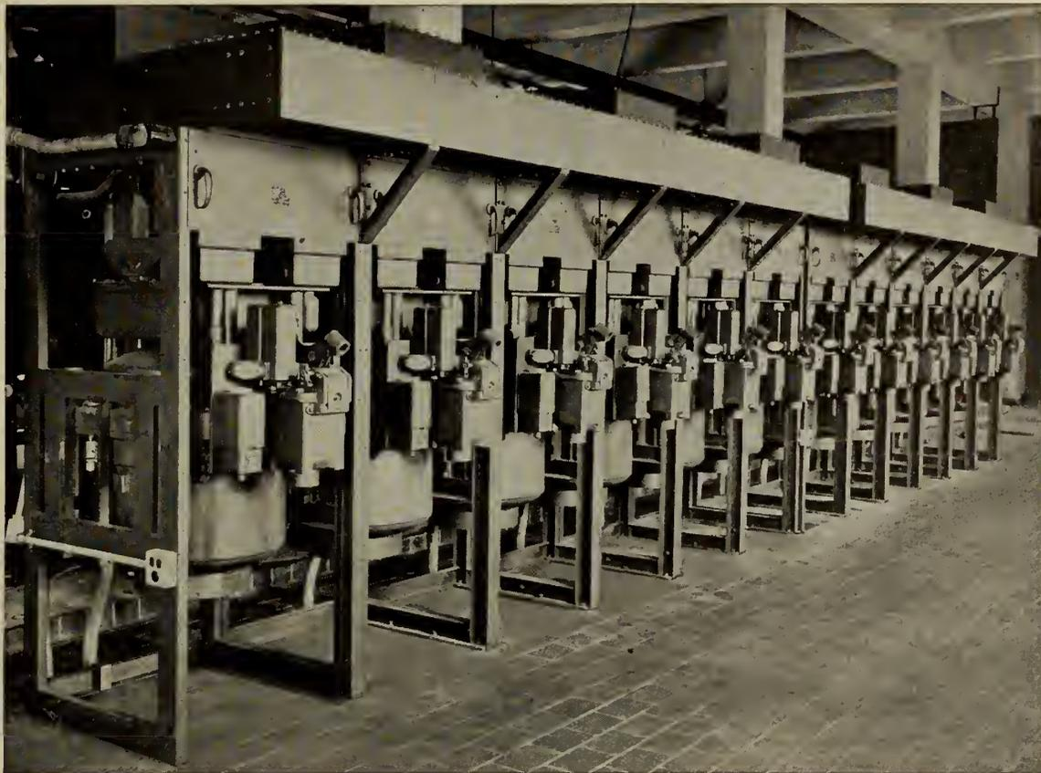
General Electric 4,150 volt metal-clad switchgear with solenoid operated oil circuit breakers installed at the Duke and George Streets Station of the Toronto Hydro Electric System.
