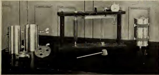
Fig. 2—Humboldt Apparatus for Concrete Durability Tests. Used in obtaining Results shown in Fig. 11.
