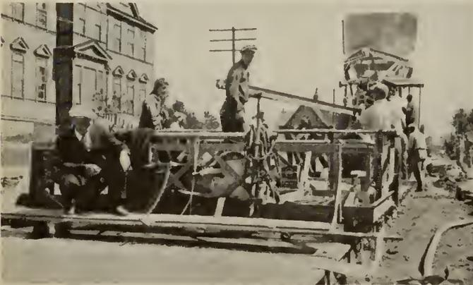
Fig. 2—Mechanical Finisher with Belt.
