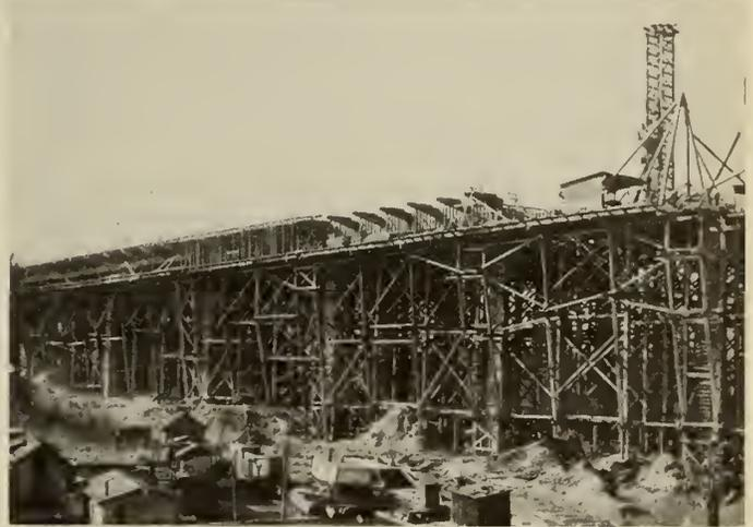
Fig. 9—Falsework for Viaduct—Bent 16 to Pier 1.
