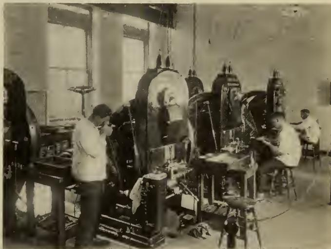
Fig. 5—The Coining Presses.
