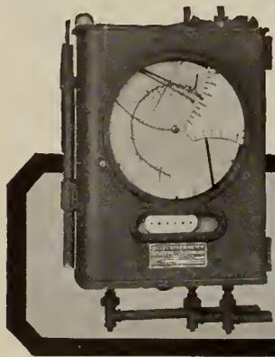
**INDICATE:** Steam Flow, Air Flow and Furnace Draft.
