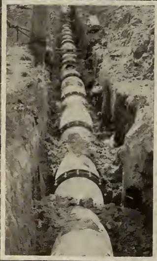
**W**ORKING under difficulties that otherwise would have slowed up even an expert construction crew, unskilled men laid 7,800 feet of this 24-inch cement-lined, cast-iron pipe in fast time—with Dresser Couplings. The pipe was easily coupled in a wet ditch. At 75 pounds pressure, it is now serving a new 7,000,000-gallon reservoir in Kalamazoo, Mich. Each and every joint is permanently and *absolutely* tight.
