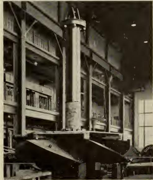
Fig. 10—Turbine Runner and Shaft Ready for Installation.
