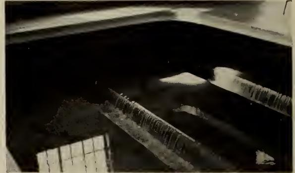
Fig. 5—Rapid Sand Filter During Wash.
