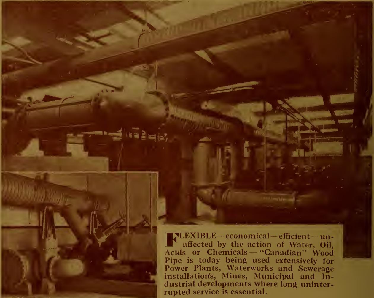
*Above is shown white water pumps and "Canadian" Wood Piping in the Powell River Company's new plant; and below, another view of "Canadian" Wood Pipe in use at a paper plant. Note how flexible and adaptable to any requirement this type of pipe is.*
