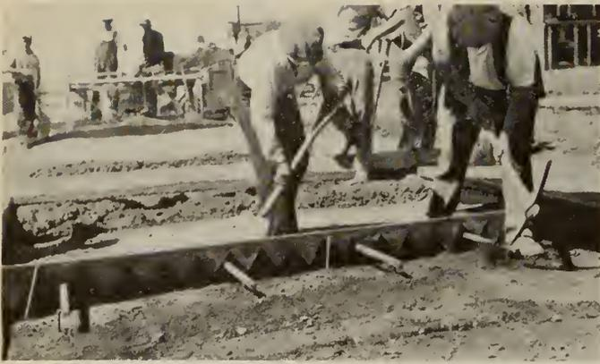
Fig. 1—Premoulded Expansion Joint—Dowels and Sleeves in Place.
