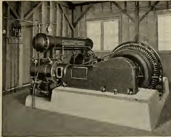
**A** modern "PRE-2" Compressor at Coniaurum Mines, Schumacher, Ont. . . . one of three installed since 1924.
