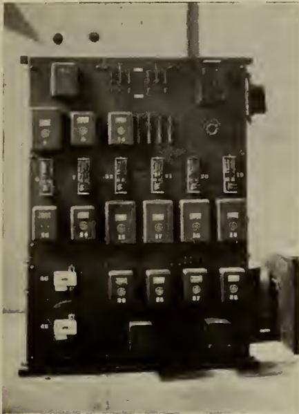
Fig. 11—Switchboard and Electrical Control Apparatus for Boiler, Fig. 10.
