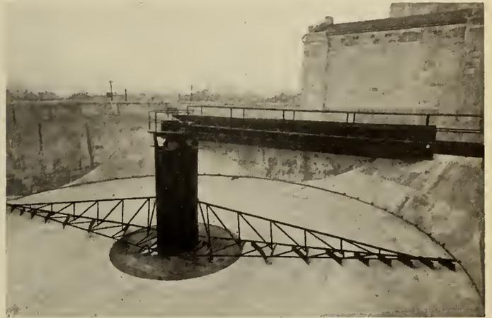
Fig. 3—Mechanical Collecting Unit in a Settling Basin.
