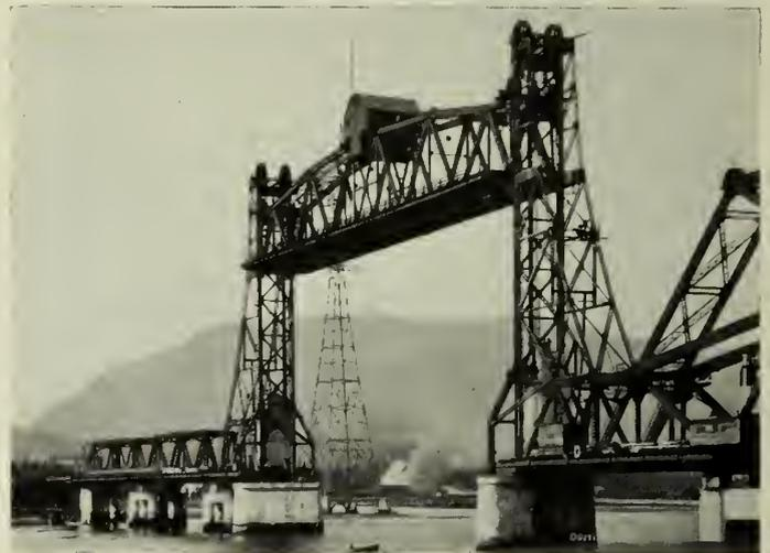
Fig. 24—Span Lifted for First Time.
