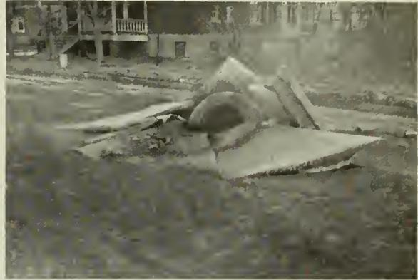
Fig. 9—Manhole Frame and Cover torn from Pavement.
