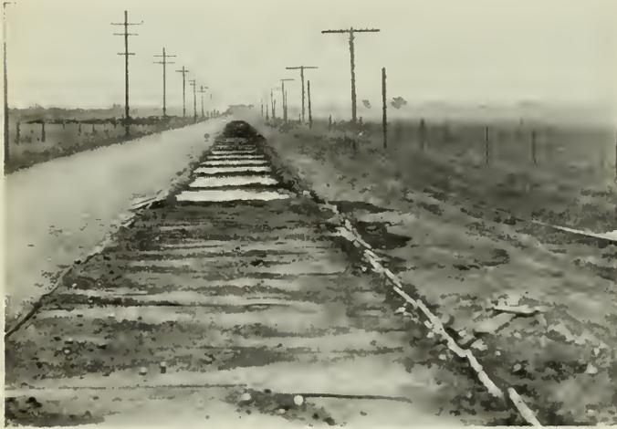
Fig. 6—Curing by Ponding.
