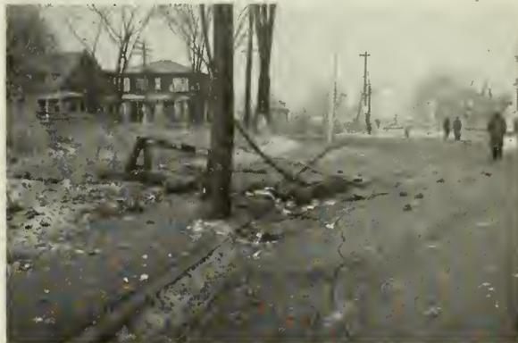
Fig. 5—Telephone Cable Torn from Pole by Manhole Cover.
