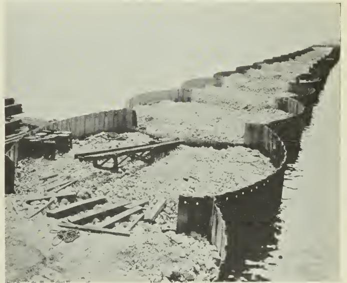
Fig. 6—Cellular Sheet Pile Breakwater, Calumet Harbour.
