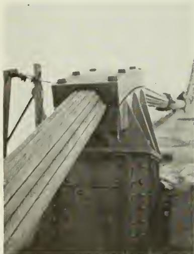
Fig. 10—Cable Bent Saddle.
