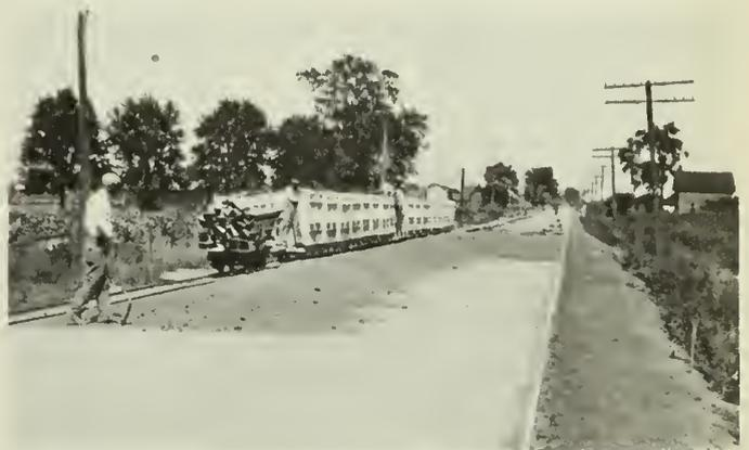
Fig. 2—Delivery of Material by an Industrial Railway.
