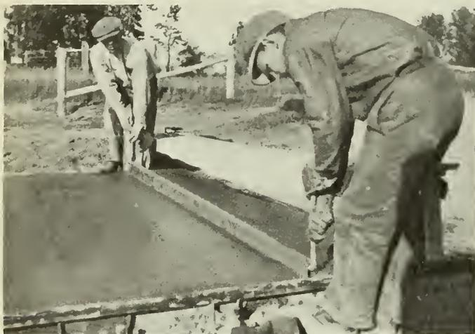
Fig. 4—Removing Joint Plate.
