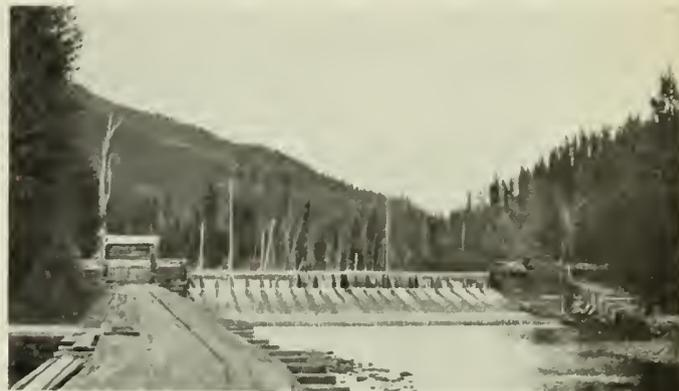
Fig. 2—Diversion Dam at the Head of the Barriere Flume.
