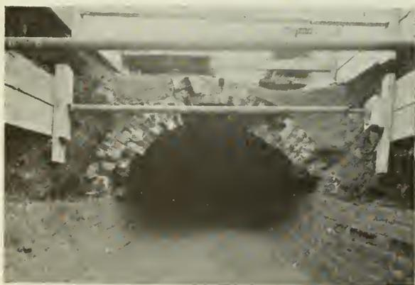
Fig. 6—Effect of Gasoline Explosion on 6-foot diameter Brick Sewer.
