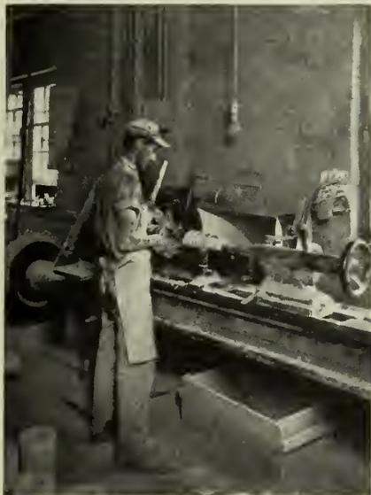
Fig. 9—Operator Turning Transformer Bushing.
