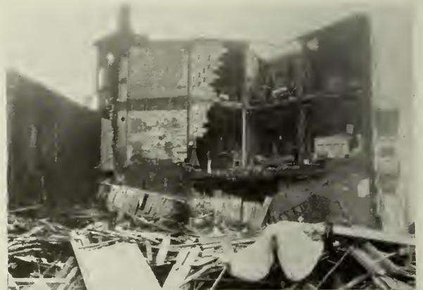
Fig. 3—Effect of Explosion in Basement of Dwelling of Block Construction.
