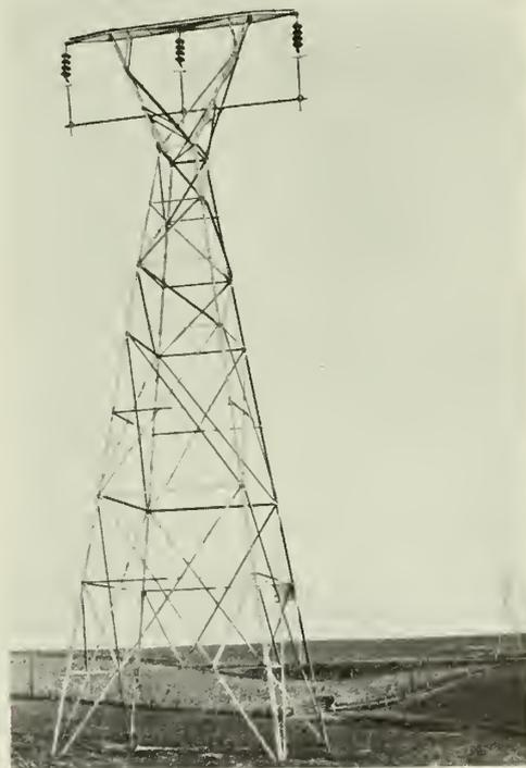
Fig. 5—Steel Tower on Clinton Dubuque 66-kv. Line.
