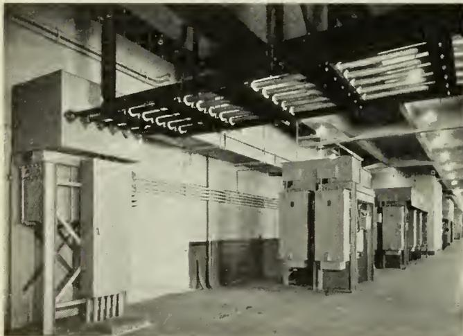
Fig. 11—Metal Clad Switching Equipment for the Frequency Changer Set and Generators Nos. 2 and 3.
