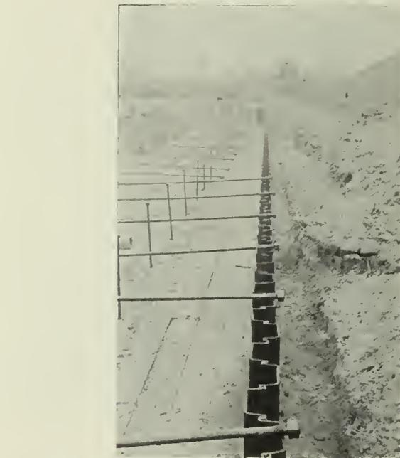
Fig. 9—Relieving Platform Type of Wharf Wall under Construction.
