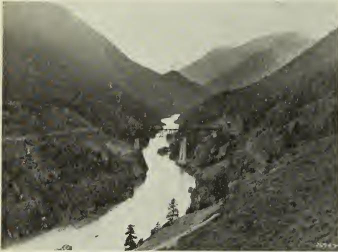
Fig. 4—Crossing the Fraser River North of Lillooet. Steel Truss and Concrete Bridge, Length 821 feet, Height 265 feet.
