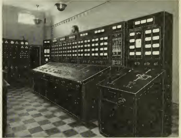
Fig. 13—Control Desk and Metering Board in the Control Room.
