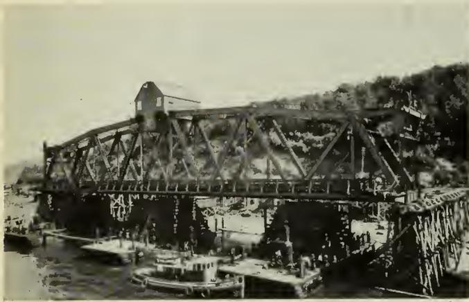
Fig. 22—Scows in Place under Lifting Span.
