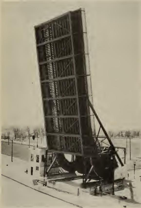
Fig. 31—Rolling Lift Bascule, Welland Ship Canal. Simple modern type for moderate spans. 1929.
