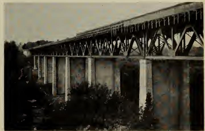
Fig. 11—Yonge Boulevard Bridge, near Toronto. Heavy Warren truss structure on reinforced concrete H-piers. 1928.
