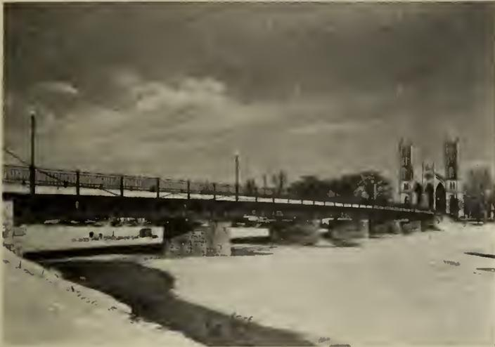
Fig. 31—Arc Welded Continuous Deck Plate Girder Bridge at Ste. Anne de la Perade, P.Q.
