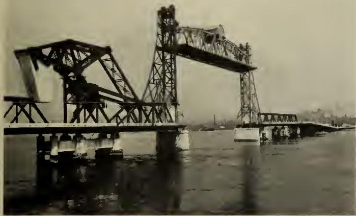
Fig. 34—Reconstructed Second Narrows Bridge, Vancouver, B.C. Prestressed counterweight ropes used without equalizers. Chromador steel extensively employed. 1935.
