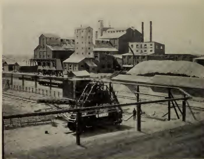
Fig. 2—Rear of factory, in foreground edge of pulp silo with pipe supply line and beet piler.
