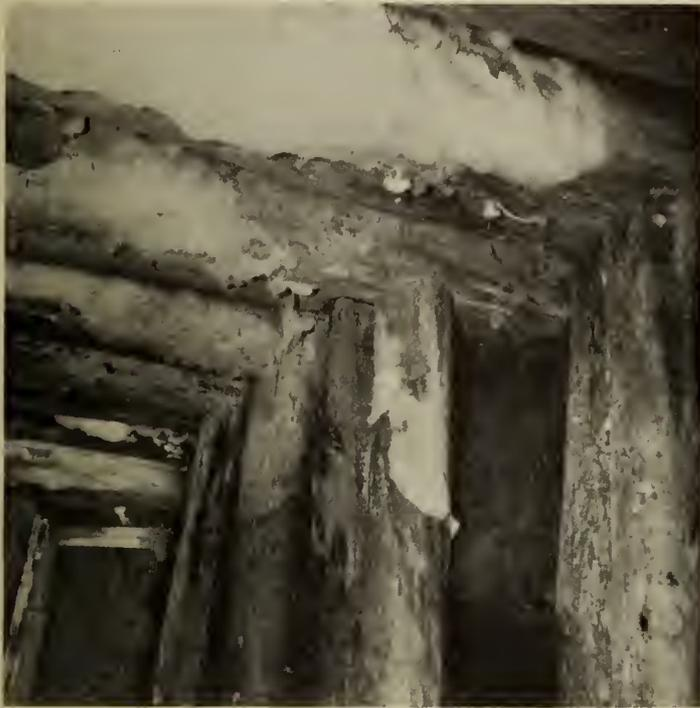
Fig. 4—Untreated drift timbers in a mine.
