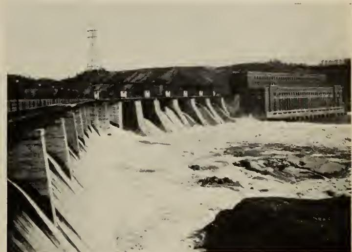
Fig. 20—La Gabelle, St. Maurice River, Que. S.W. and P. Co. Installed 1924. Present Capacity 152,000 hp.
