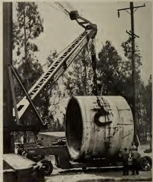
Fig. 10—Unloading 43-Ton Section of Pipe, Colorado River Aqueduct.
