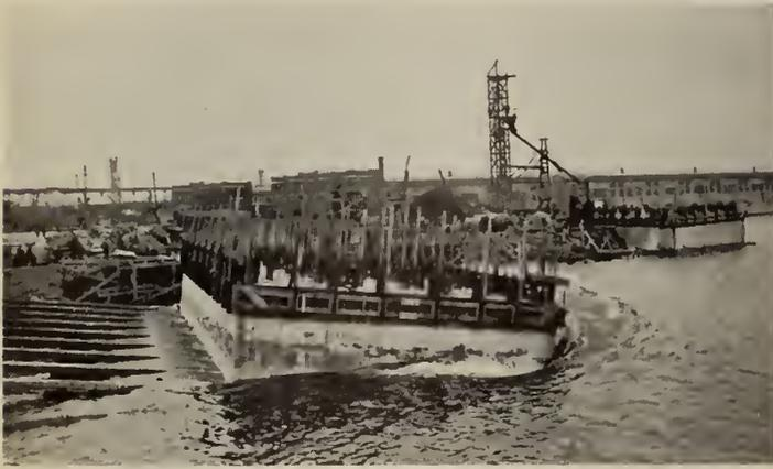
Fig. 10—Launching Crib, Imperial Oil Company Pier.
