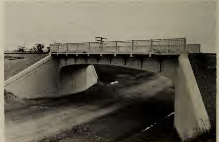
Fig. 50—C.N.R. Rigid Frame, Vaudreuil, Que. Heavy long-span grade separation structure. 1933.
