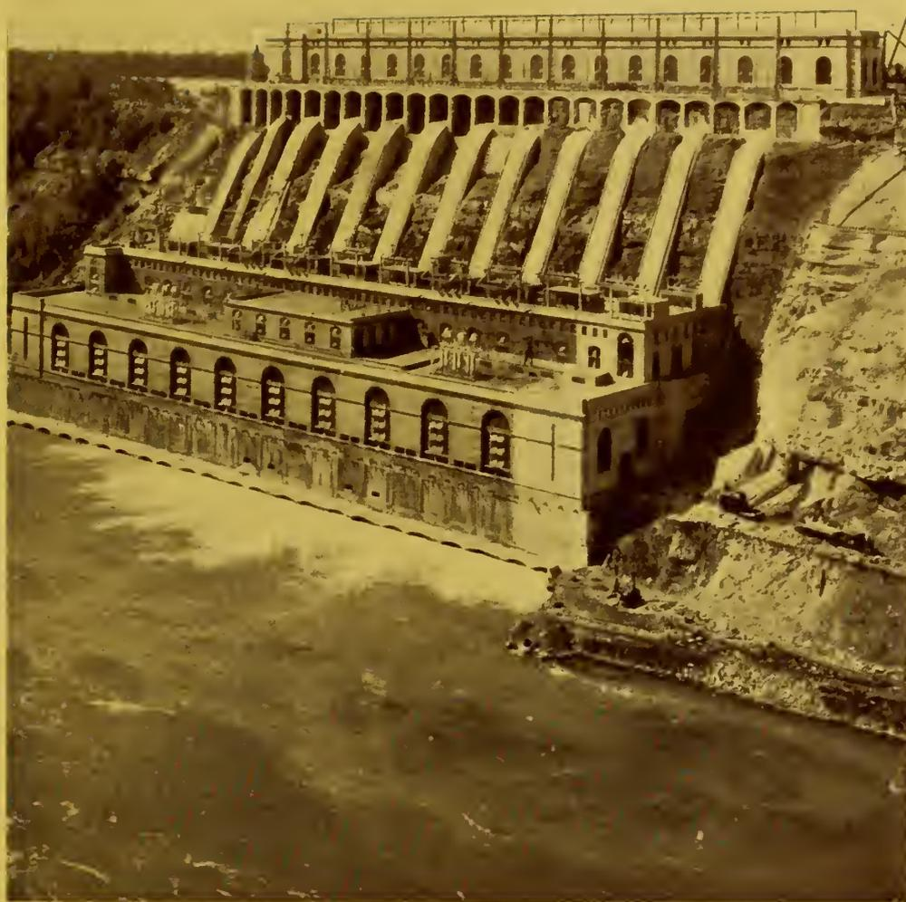
**T**HE QUEENSTON Power House of the Queenston-Chippawa Development. Its completed length, to house the ten main units and two service units which it now contains, exceeds 590 feet and operates under a head of 294 feet. If the building were placed in front of the American Falls it would nearly hide them. The total capacity of the development is 550,000 horse power.
