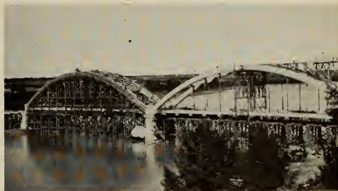
Fig. 12—Arch Ring with Hinge in Place.
