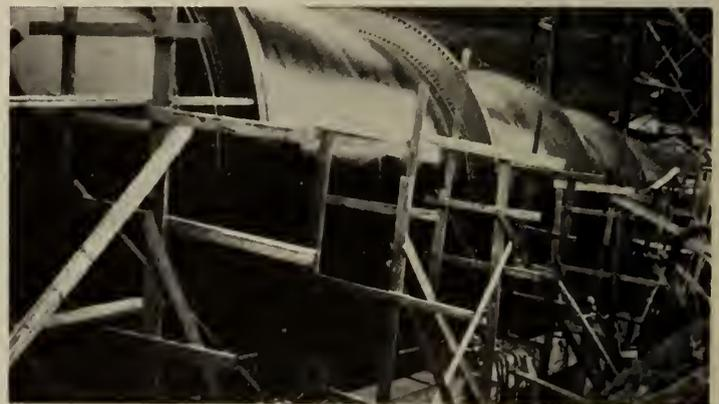
Fig. 8—18 ft. dia. Steel Pipe Showing Ring Girders and Struts.
