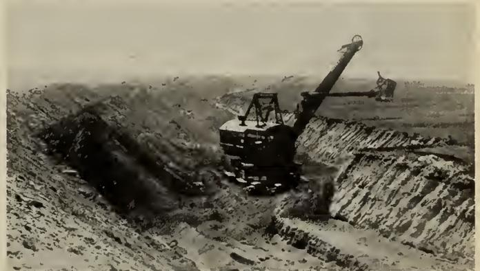
Fig. 1—Ten-ton Electric Stripping Shovel Removing Clay Overburden up to 65 Feet in Depth.
