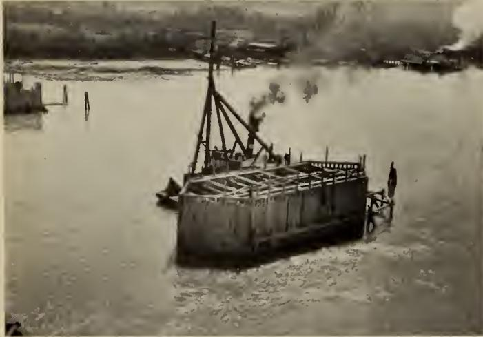
Fig. 6—No. 4 Caisson Before Grounding.
