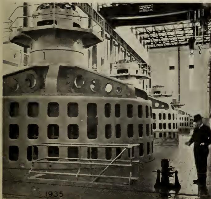
Fig. 2—1.6 hp. Dynamo, Installed 1885, Compared with Modern 34,000-hp. Generators, Chelsea Plant, Gatineau Power Company.
