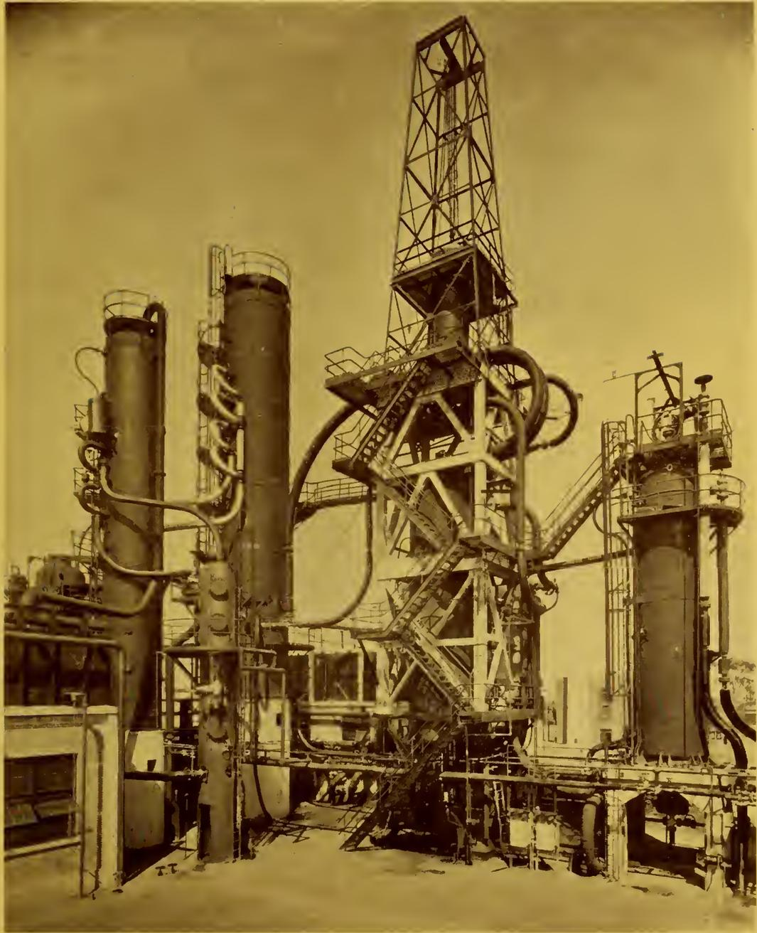
VESSELS and fractionating equipment of the combined topping and cracking plant at Shell Oil Company of Canada Limited refinery at Montreal East. This refinery was built in 1933.
