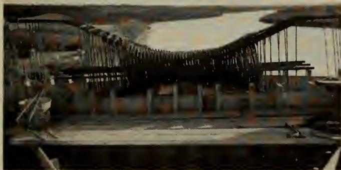
Fig. 10—Hinge Reinforcement.
