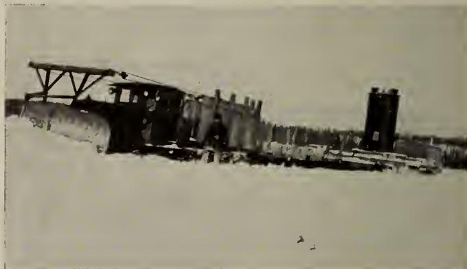
Fig. 4—Tractor-Train plowing out the Road and Transporting a Transformer.
