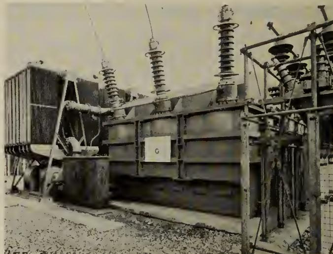
Fig. 6—75 mva. Three-Phase Transformer compared with Faraday's Induction Ring.
