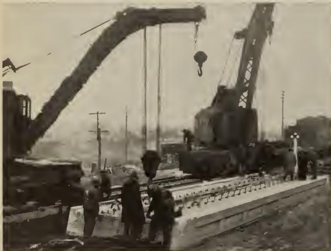
Fig. 2—Preparing to place Pre-Cast Bridge Slab.
