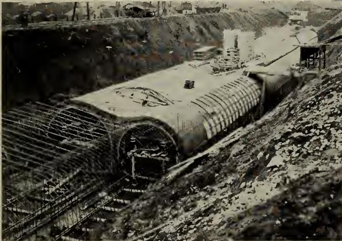
Fig. 3—St. Pierre River Collector, Montreal. Inside dimensions of Twin Section 14 ft. by 14 ft. 6 in. and 16 ft. by 17 ft. 6 in.
