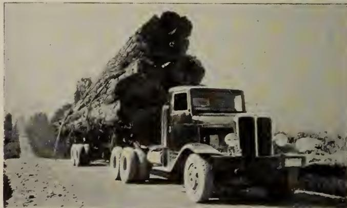
Fig. 9—Logging in British Columbia. Heavy Diesel Truck and Trailer—Load 9,000 f.b.m. (approximately 36 tons). These Trucks handle up to 50 Tons.
