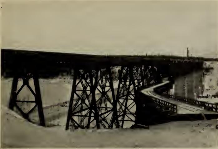
Fig. 9—C.P.R. Bridge, Saskatchewan River, Nipawin, Sask. Highway deck enters on a Y carried by brackets from railway bents. 1932.
