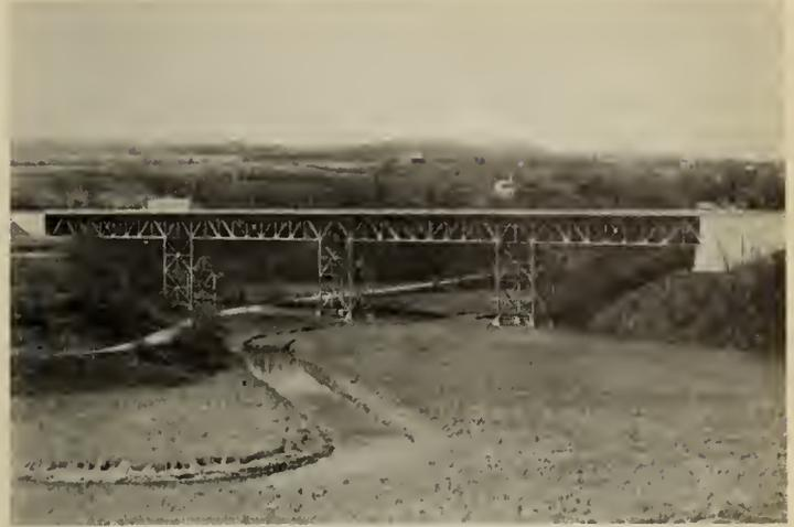
Fig. 10—Highway Viaduct at Eastern Entrance to Hamilton, Ont. Typical steel truss and tower viaduct on Ontario provincial highway. 1921.
