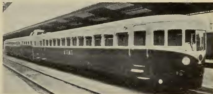
Fig. 14—Michelin-Triple-Car Pneumatically-Tired Train.
