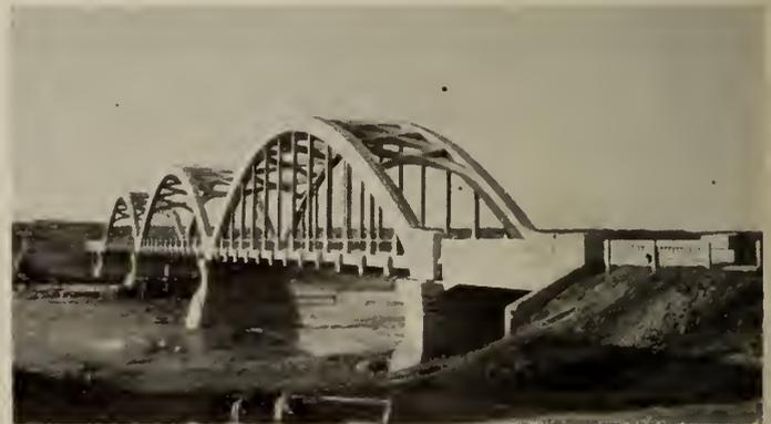
Fig. 3—Sway Bracing and Other Details.
