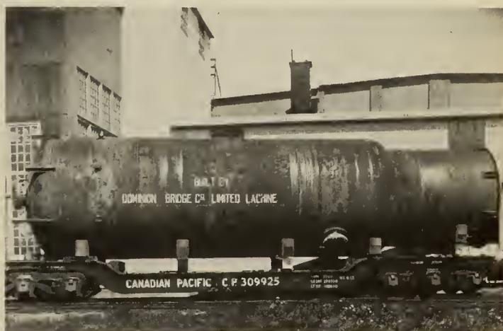
Fig. 4—Arc Welded Refinery Vessel 12 ft. dia. by 1½ in. Shell.
