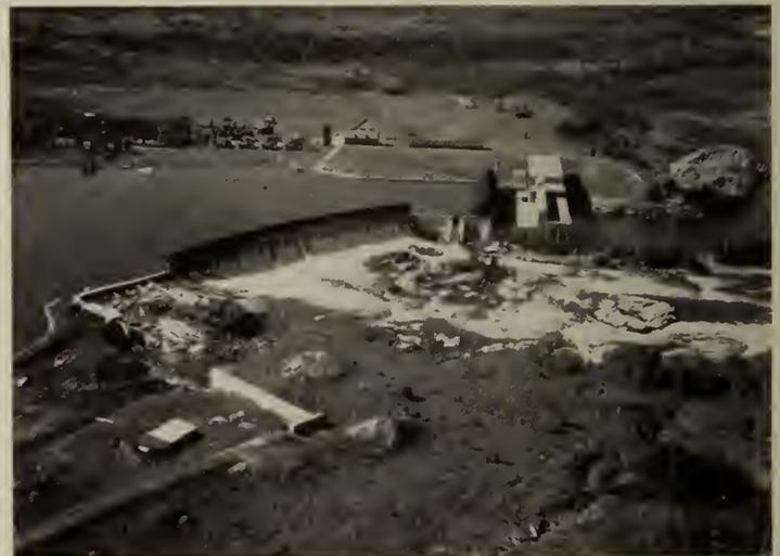
Fig. 8—Pinawa Channel Plant, Winnipeg River, Man. In operation 1906, with 37,800 hp. Winnipeg Electric Co.
