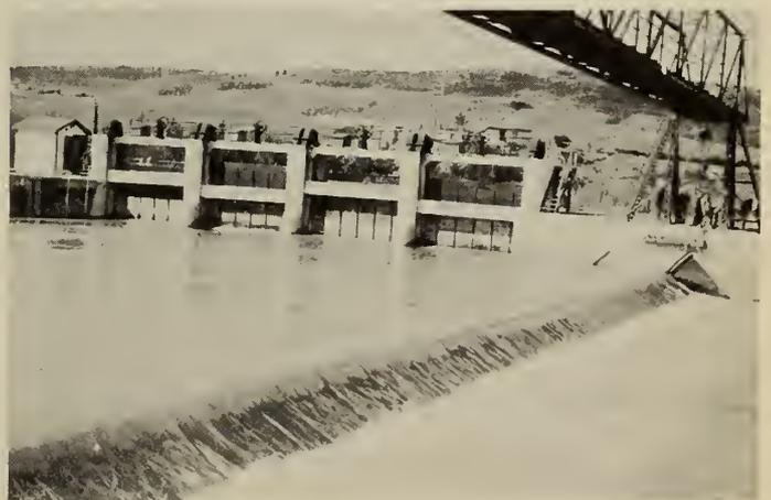
Fig. 7—Headgates of Main Canal and Movable Sector Weir, Bow River Canal.
