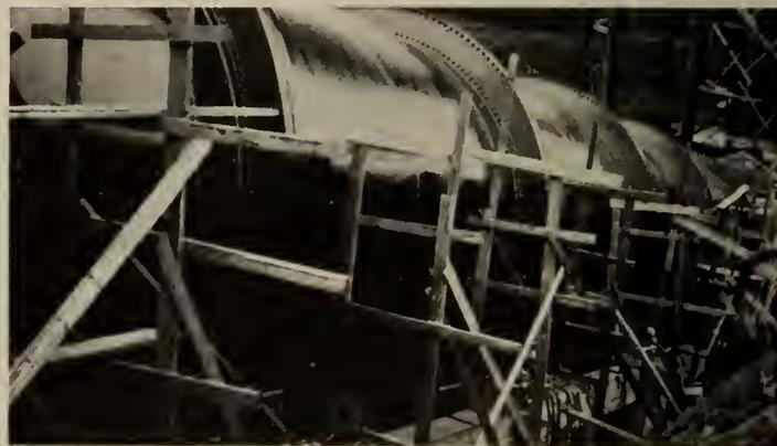
Fig. 8—18 ft. dia. Steel Pipe Showing Ring Girders and Struts.
