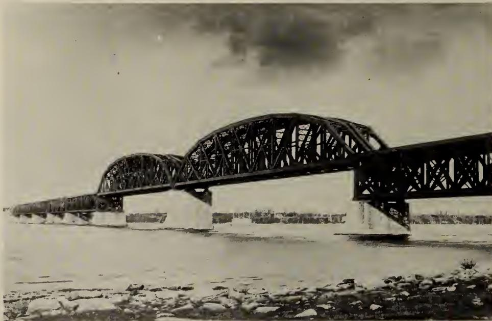
Fig. 8—C.P.R. Bridge over the St. Lawrence, Lachine, Que. The two through spans were end-launched over the previously constructed deck structure. 1913.
