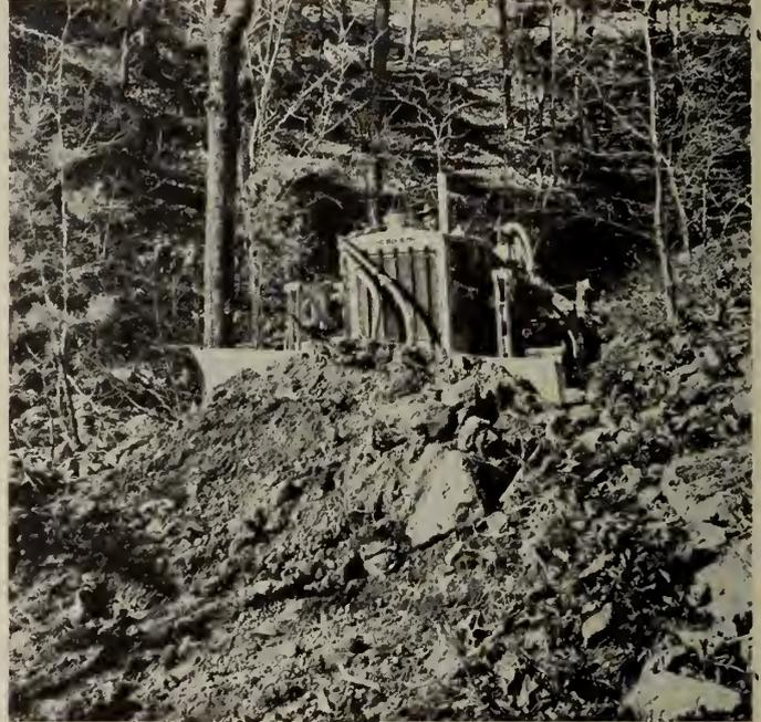
Fig. 1—Caterpillar tractor equipped with Trail-Builder building a Logging Truck Road.
