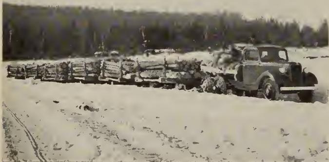
Fig. 8—A Ford-Warford Truck hauling a Train of six Sleighs.
