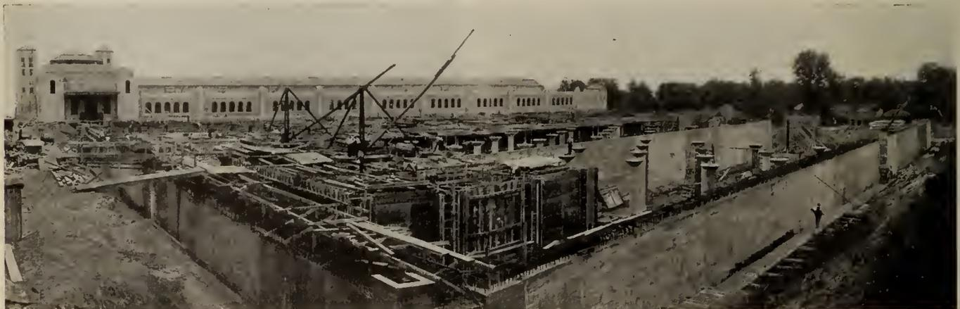
Fig. 6—Northerly Elevation of Victoria Park Filter House, Toronto. Mixing and Settling Tanks in Foreground.
