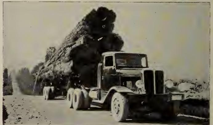
Fig. 9—Logging in British Columbia. Heavy Diesel Truck and Trailer—Load 9,000 f.b.m. (approximately 36 tons). These Trucks handle up to 50 Tons.
