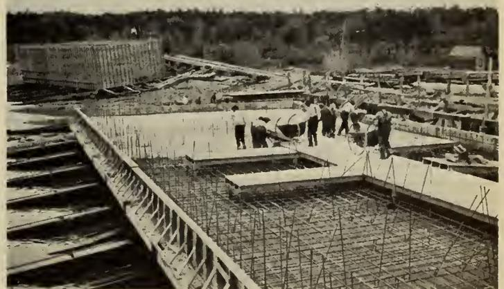
Fig. 9—Building Cribs, Imperial Oil Company Pier.
