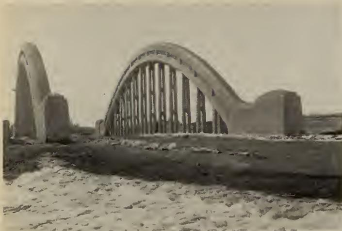
Fig. 47—Dubois St. Bridge over Montreal Aqueduct. Dumb-bell type of spirally-reinforced compression chord. Piers rock on sand cushions. 1930.
