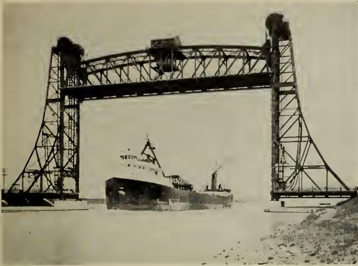
Fig. 33—Vertical Lift Bridge, Welland Ship Canal, Allanburg. Typical of the eleven vertical lift bridges over the canal. 1929.
