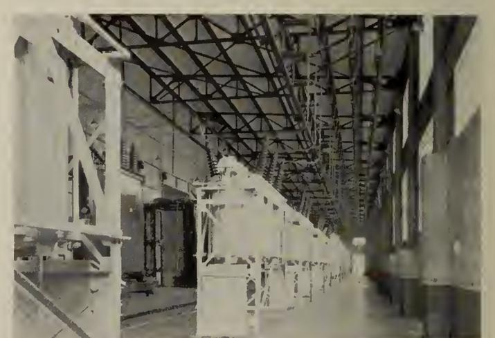
Fig. 4—No. 3, H.T. Step-down Station, Zinc Plant.
