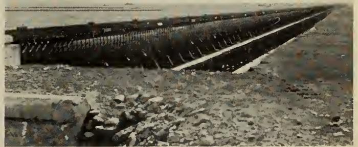
Fig. 11—Lathom, Semi-circular Wood Stave Flume 15 ft. diameter, 2,593 ft. long.
