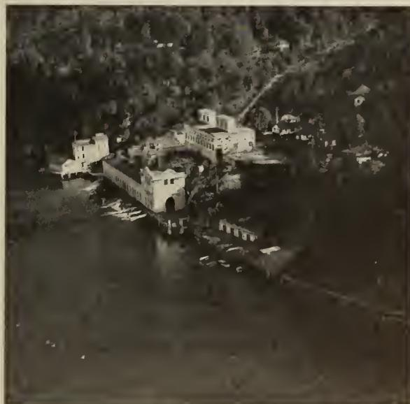
Fig. 5—Coquitlam-Buntzen Development No. 1 of British Columbia Power Corp. first operated 1904, Present capacity 43,500 hp., Head 395 ft.
