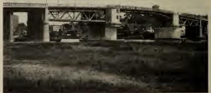
Fig. 32—Double-Leaf, Simple Trunnion Bascule, Sorel, Que. Characteristic example of modern simple trunnion design. 1932.
