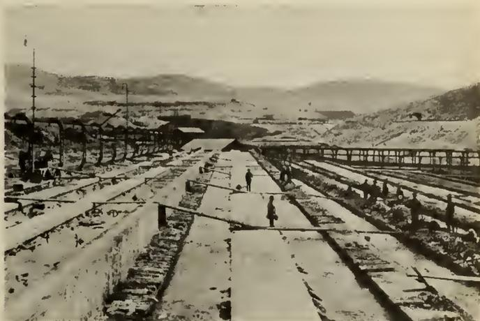
Fig. 6—Cementation Launders where Copper Liquors pass over Scrap Iron.
