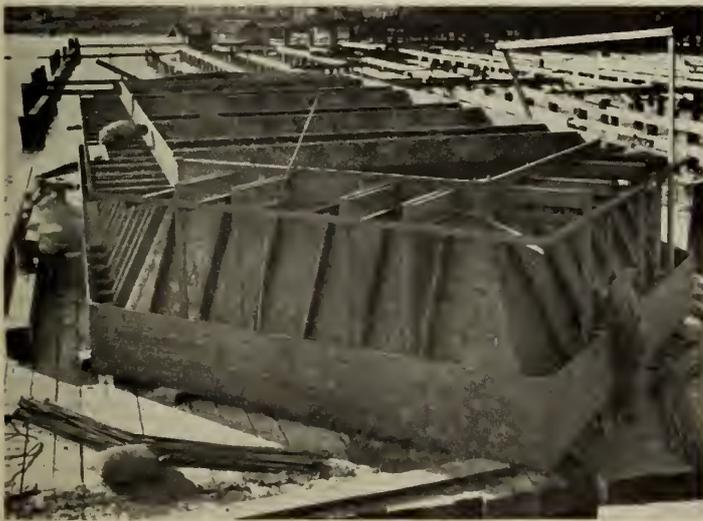
Fig. 4—Cutting Edge for No. 1 Caisson.
