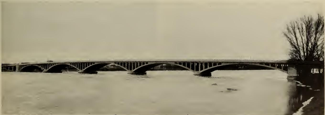
Fig. 41—Ahuntsic Bridge, Back River, near Montreal. Important instance of 3-hinged reinforced concrete arch construction. 1930.
