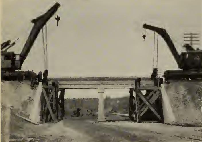
Fig. 53—C.N.R. Precast Slab Bridge, St. George, Ont.
