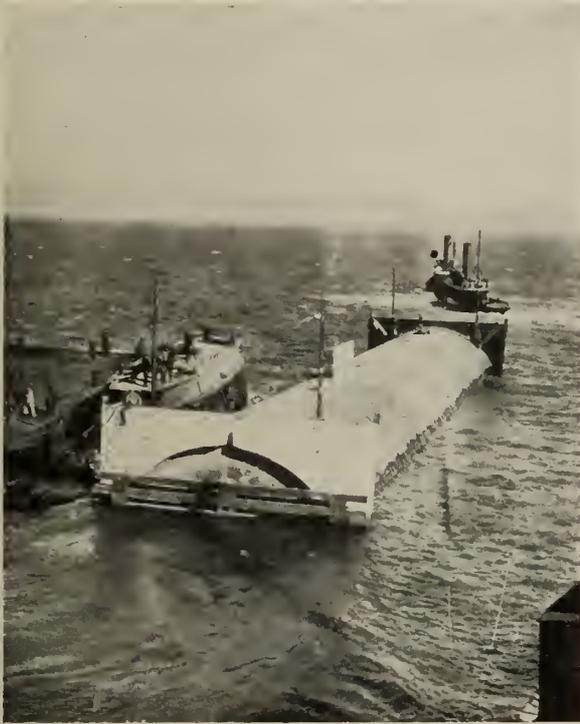
Fig. 11—Towing Pre-Cast Tunnel Section to Site, Alameda Tunnel.
