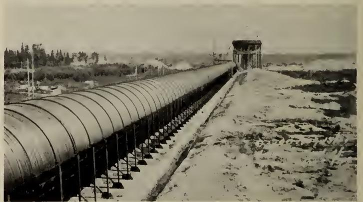
Fig. 11—Completed Wood Stave Pipe.
