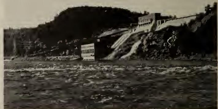
Fig. 28—High Falls, Lievre River, Que. In Operation 1930, Capacity now 120,000 hp. McLaren-Quebec Power Co.
