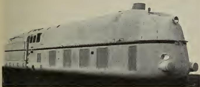
Fig. 10—Streamlined 4-6-4 German Reichsbahn Locomotive Class 05.
