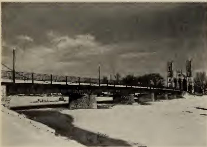
Fig. 27—Welded Continuous Plate Girder Bridge, La Perade, Que. Most important all-welded bridge in Canada. 1936.
