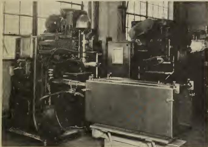
Fig. 9—Modern Spot Welders used in the Production of All-Steel Refrigerator Cabinets.
