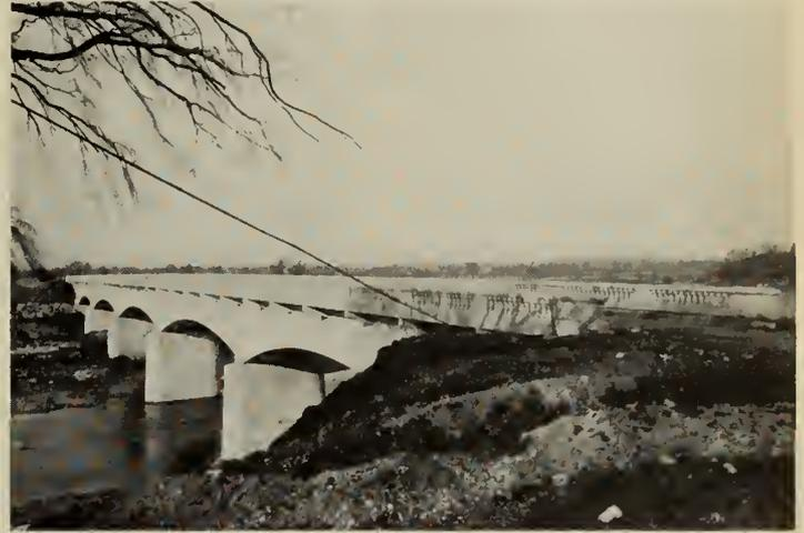
Fig. 51—Cockshutt Cantilever Bridge near Brantford, Ont. Expansion by reinforced concrete rockers in pier recesses. 1933.
