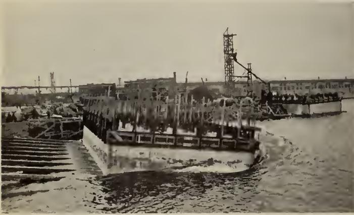
Fig. 10—Launching Crib, Imperial Oil Company Pier.
