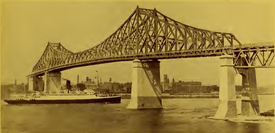
**I**SLE OF ORLEANS Bridge, (*top*) over St. Lawrence River, six miles below Quebec City. Total length including approaches,  $1\frac{1}{2}$  miles. Suspension span, longest of its type in Canada, 1,059 feet centre to centre of main piers. Two side spans 419½ feet each.
