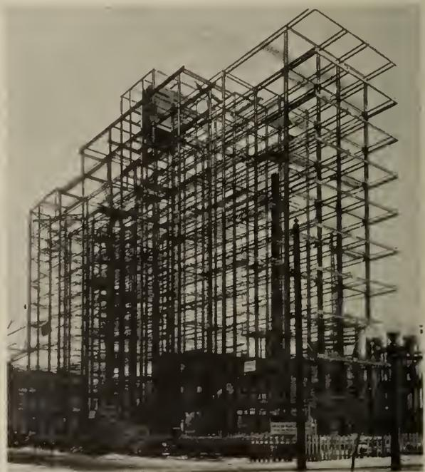
Fig. 30—All Welded Steel Addition to Western Hospital, Montreal, Designed for Composite Construction.
