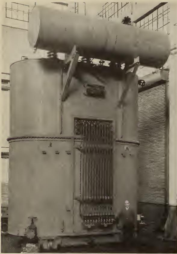
Fig. 1—Arc Welded Transformer Tank, Canadian Westinghouse.
