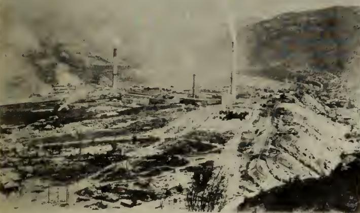
The works of Shawinigan Chemicals Limited, producing calcium carbide and glacial acetic acid, is one of the largest in the world and the greatest of its kind in the Empire. Carbide is made from limestone and coke in electric furnaces. The acetylene gas therefrom is the base for acetic acid. Products are shipped to all parts of the world. The company employs about 1000 people and uses 75,000 h.p. of electricity.
