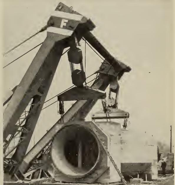
Fig. 5—Three-Way Pre-Cast Distributor, Toronto Waterworks Intake.
