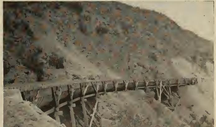
Fig. 3—Metal Flume, South Okanagan Project, B.C.
