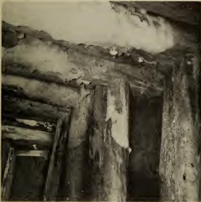
Fig. 4—Untreated drift timbers in a mine.
