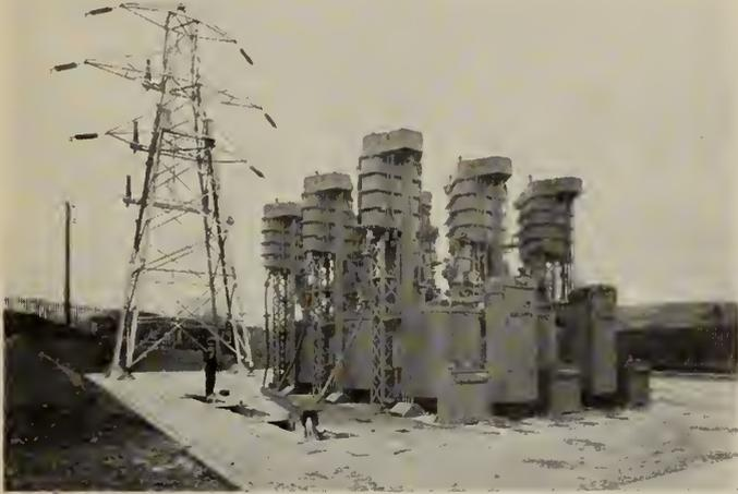
Fig. 9—Metal Clad 132-kv. Switchgear at Tongland.
