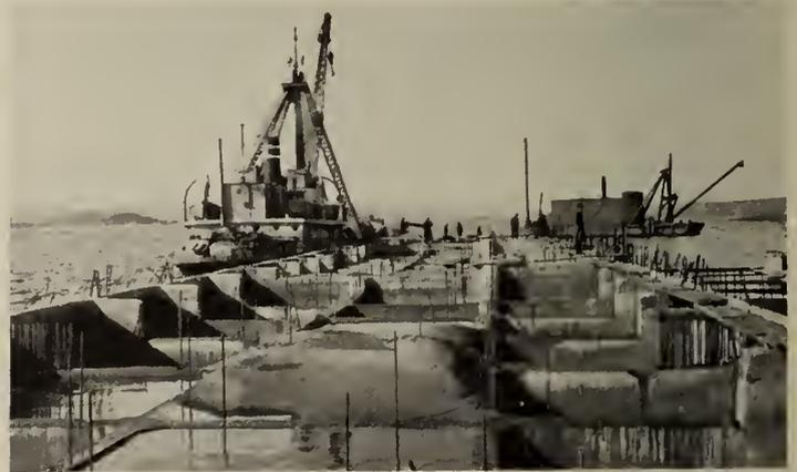
Fig. 11—Filling Cribs, Imperial Oil Company Pier.
