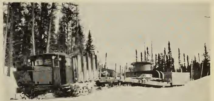
Fig. 7—Tractor Train transporting Generator Spider and other Equipment.
