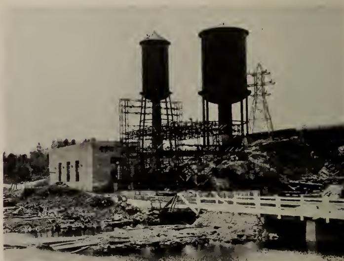
Fig. 18—Musquash Development of N.B. Electric Power Comm. Completed 1922. 11,100 hp.
