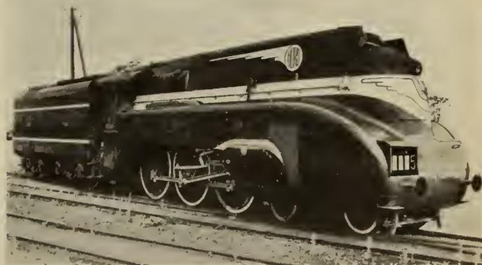
Fig. 7—Super-Pacific Streamlined Locomotive of the Northern Railway of France.
