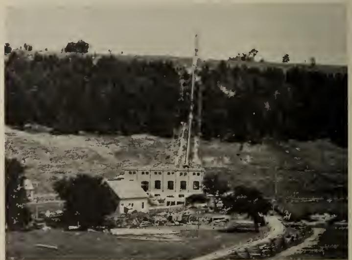
Fig. 13—Eugenia Falls, Beaver River, Ont., H.E.P.C. of Ont. Installed 1915. Present Capacity 8,500 hp. Head 549 ft.
