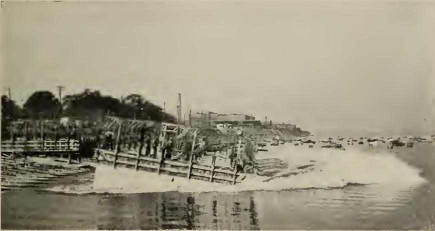
Fig. 4—Method of Launching Caisson at Halifax.
