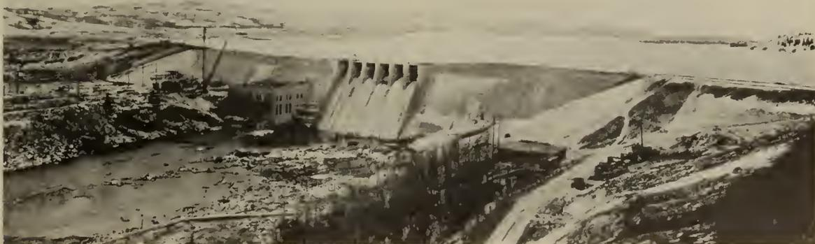
Fig. 25—Ghost Development, Bow River, Alta. Installed 1929 with 36,000 hp. Calgary Power Co.
