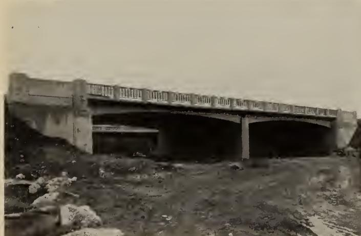
Fig. 48—Two-Span Rigid Frame, Etobicoke River. First use of multiple-rib type in Canada. 1935.
