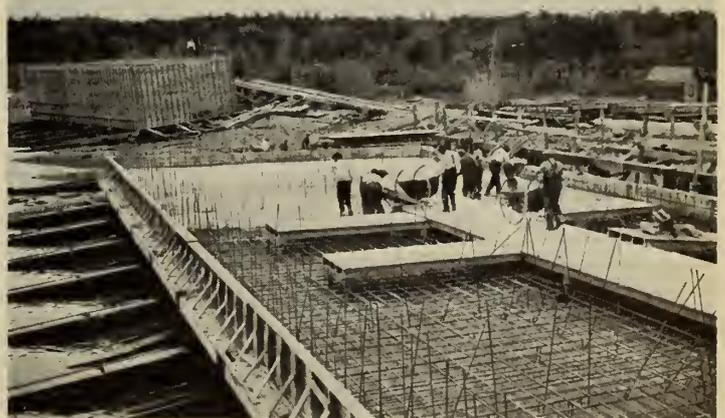
Fig. 9—Building Cribs, Imperial Oil Company Pier.
