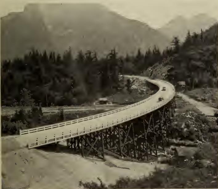
Fig. 3—Highway overhead crossing at Haig, B.C. Composite concrete creosoted timber deck on creosoted timber bents.
