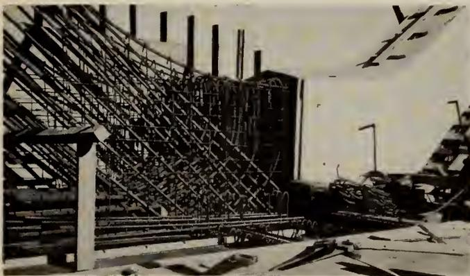
Fig. 8—Terminal Block Reinforcement.
