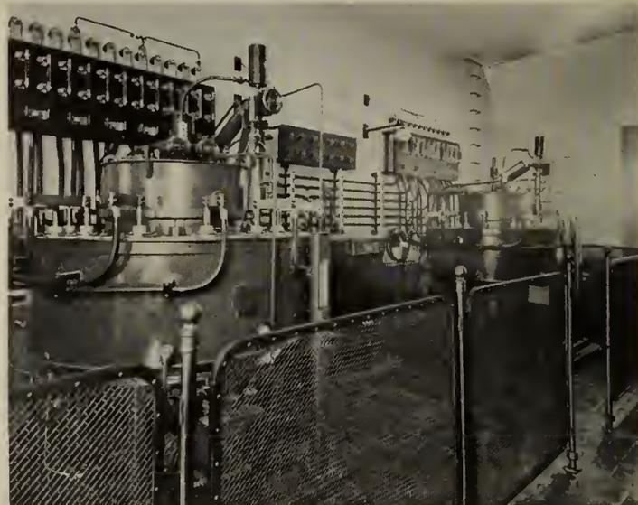
Fig. 19—Queen Mary Road Substation, Montreal. Two 1,500-kw. Mercury Arc Rectifiers. Operation Fully Automatic and Supervisory Controlled.
