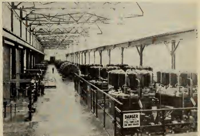
Fig. 6—Rotary Converters, and Mercury Arc Rectifiers, Zinc Plant.
