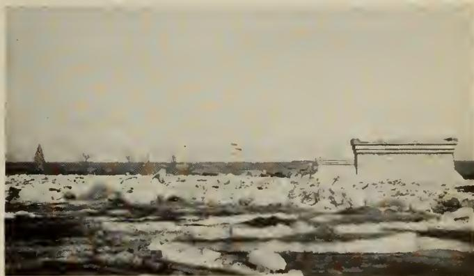
Fig. 17—Pier 3 and Ice "break up."
