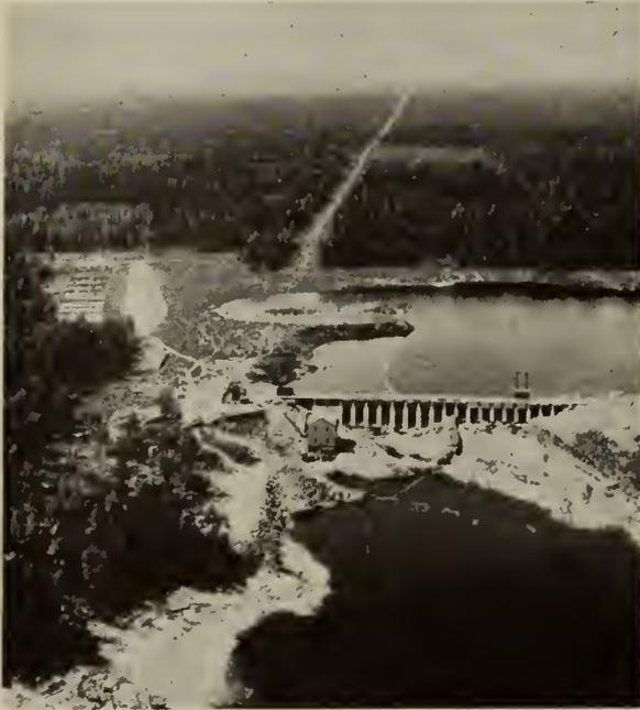
Fig. 5—Ear Falls Development. Showing Lac Seul Conservation Dam, Power House and Transmission Line to Red Lake.
