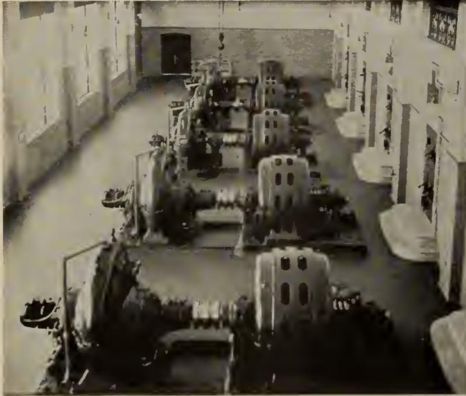
Fig. 5—Main Pumping Station, Montreal. Highlift Pumps.
