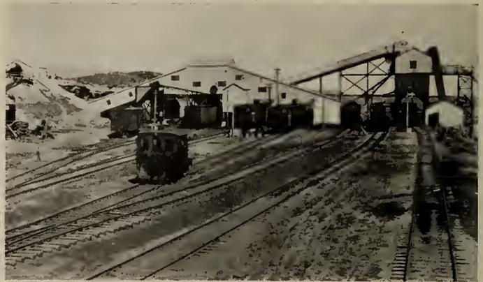
Fig. 7—Tipple at Truax-Traer Opencast Mine, showing Rotary Pump (left) and Pneumatic Cleaning Plant (right).
