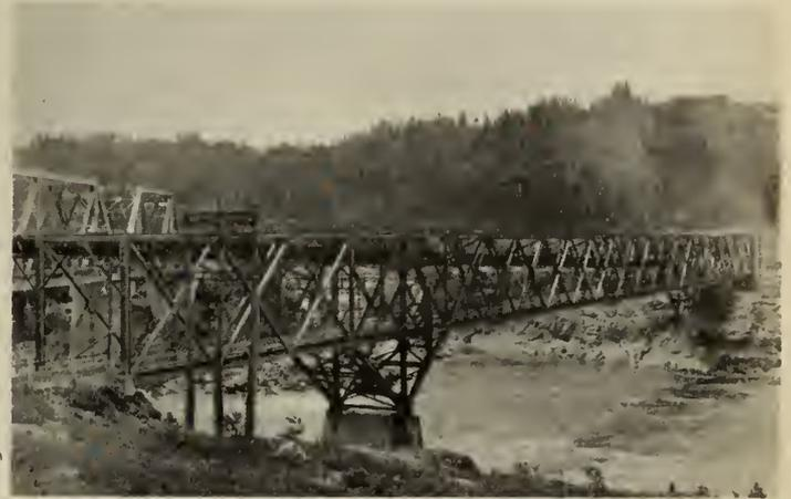
Fig. 25—Saguenay River Continuous Bridge at Kenogami. Economical structure with low piers. 1922.
