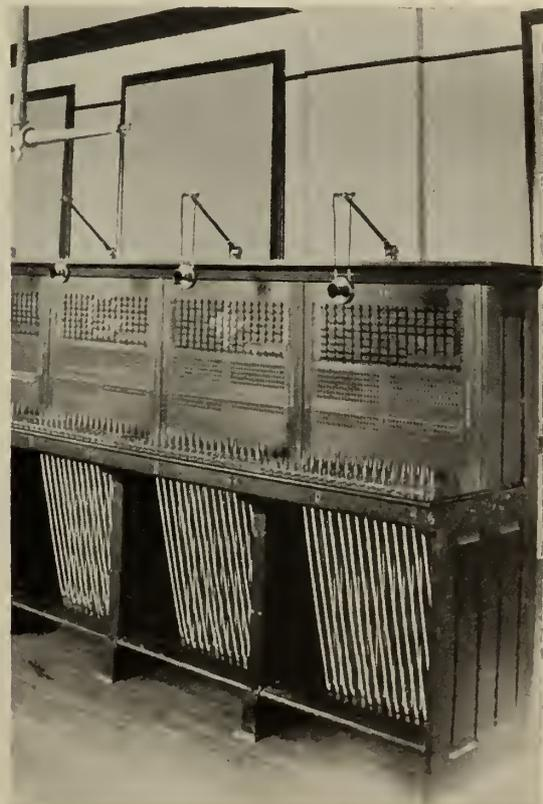
Fig. 7—Three Sections of Winnipeg's Switchboard in 1896, with one hundred Subscribers' Lines per Section.
