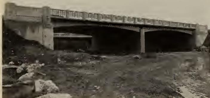
Fig. 48—Two-Span Rigid Frame, Etobicoke River. First use of multiple-rib type in Canada. 1935.
