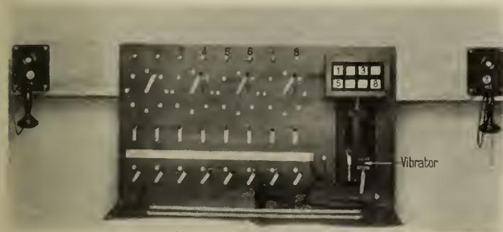
Fig. 6—Typical 8-Line Telephone Switchboard of about 1880.
