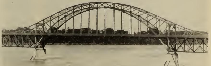
Fig. 26—Honoré Mercier Bridge, Lachine, Que. Contains a unique continuous tied arch span. 1934.
