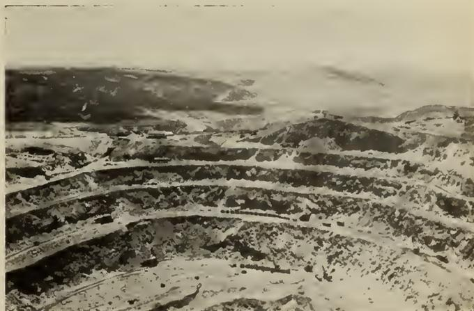
Fig. 1—Rio Tinto. Atalaya Opencast. Porphyry on the Right, Slate on the Left, with Ore Between.
