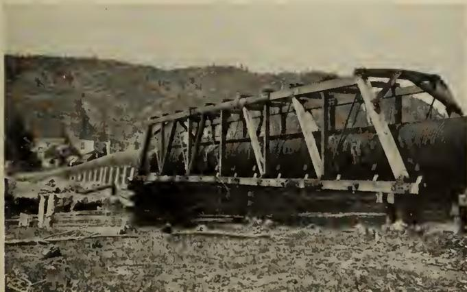
Fig. 1—Truss Bridge Carrying Inverted Siphon across Okanagan River.
