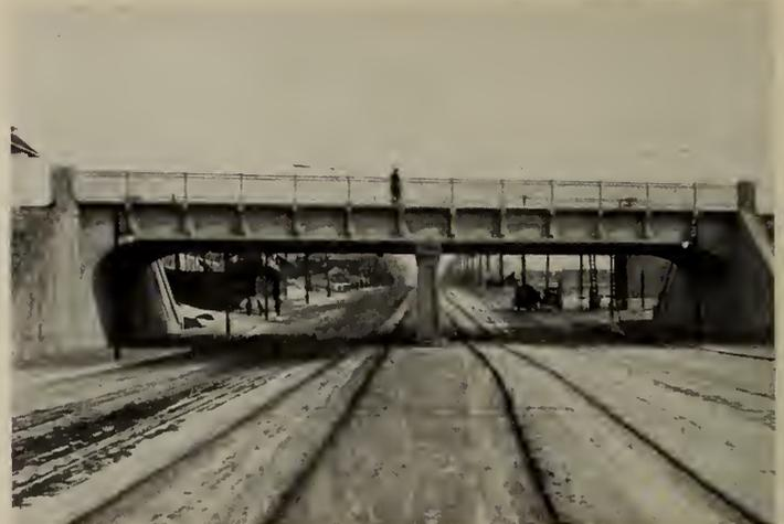
Fig. 49—C.N.R. Two-Span Rigid Frame, St. Clair Ave. West, Toronto. Rests freely on centre pier. Shallow concrete ties and no ballast used. 1931.
