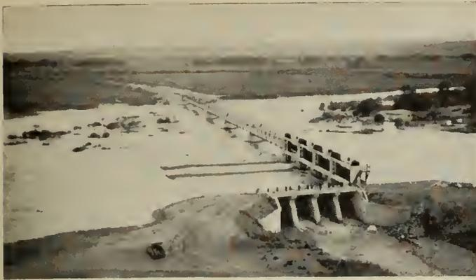
Fig. 13—Diversion Dam, Sluice Gates and Headgates on Oldman River.
