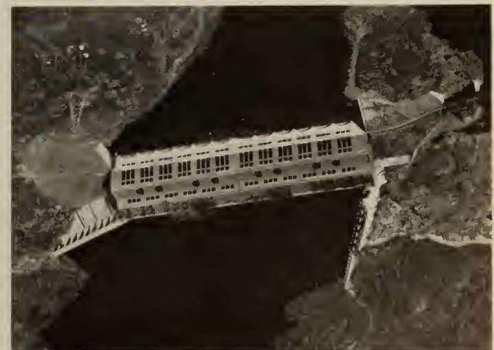
Fig. 21—Isle Maligne, Saguenay River, Que. Installed 1925 by Duke-Price Power Co. Capacity now 495,000 hp.
