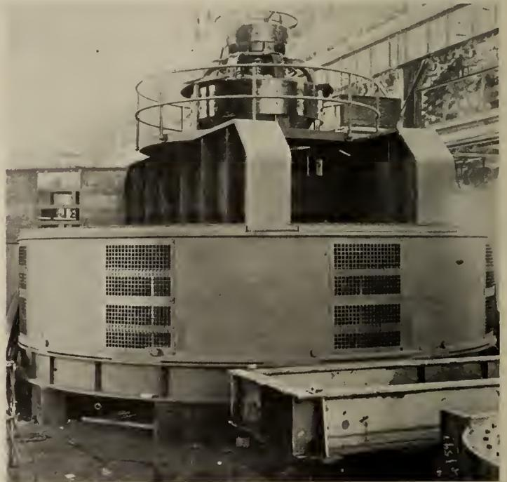
Fig. 2—Arc Welded A.C. Generator, Canadian General Electric.
