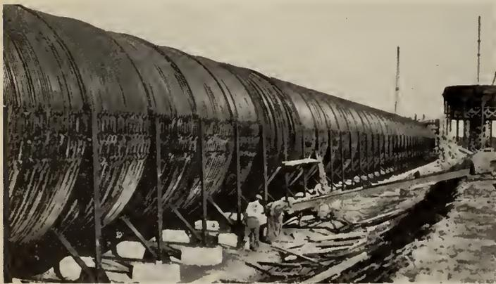
Fig. 10—Cinching and Spacing Bands on Wood Stave Pipe.
