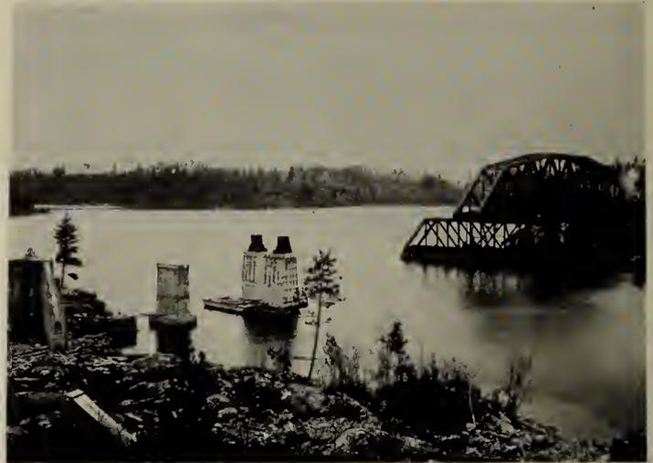
Fig. 7—Erection of the C.P.R. Bridge over the French River. Span end-launched across the river in three hours. 1907.
