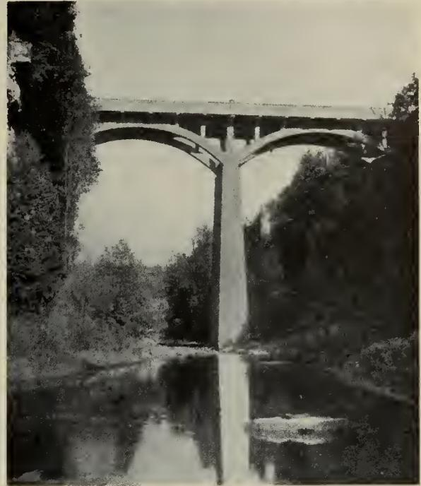
Fig. 40—Twin Arches on 80-ft. Masonry Pier, Elora, Ont. Trusses of old bridge supported forms which were built as a tied arch. 1921.
