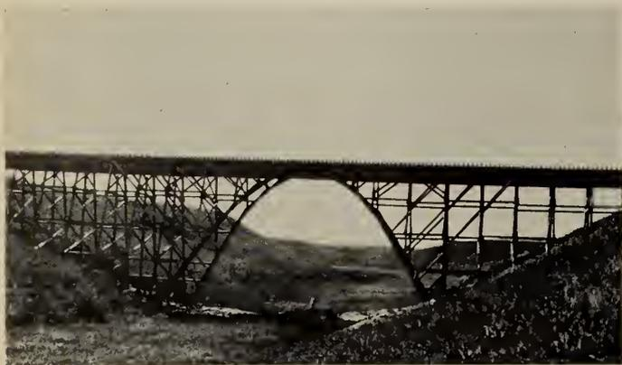
Fig. 8—Winona Semi-circular Metal Flume, 7 ft. 2 in. diameter, Arch Span 64 ft.
