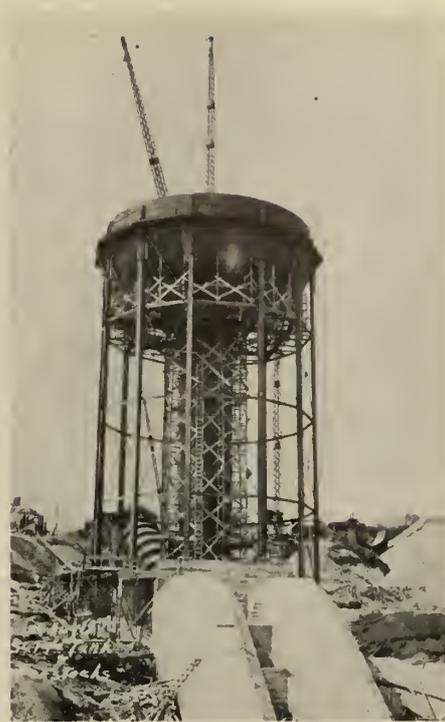
Fig. 9—Concrete Encased Penstocks, Surge-tank and Steel Pipe Line.
