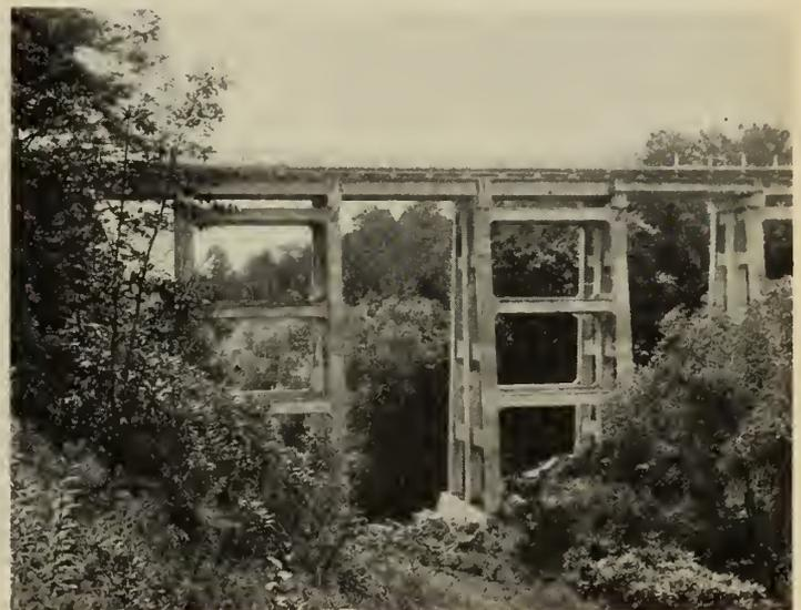
Fig. 35—C.P.R. Reinforced Concrete Viaduct, Toronto. Precast T-beam units weighing 55 tons placed by wrecking crane. 1918.
