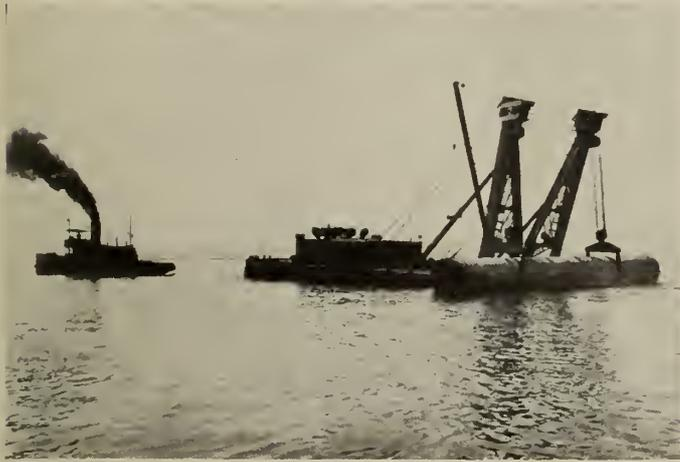
Fig. 1—Transporting 250-Ton Section of Pipe, Toronto Waterworks Intake.
