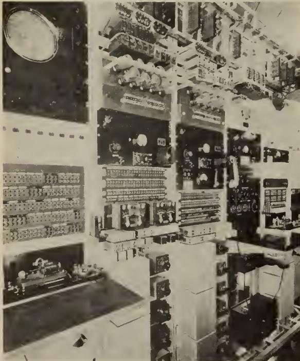
Fig. 8—Telephone Repeater Equipment used in Transmitting Radio Programmes for Network Broadcasting.
