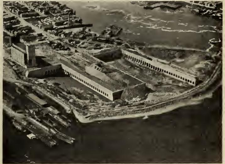
Fig. 4—Navy Island Development, Saint John, N.B., before Removal of Cofferdam.
