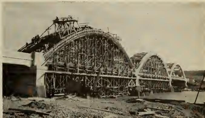
Fig. 19—Falsework and Forms during Concreting.
