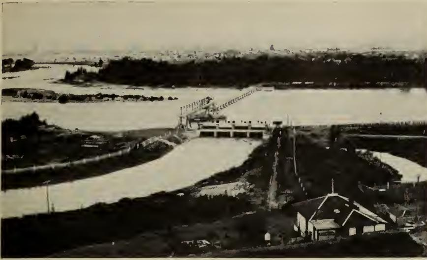
Fig. 6—Diversion Weir and Main Canal Headgates, Bow River, Calgary.
