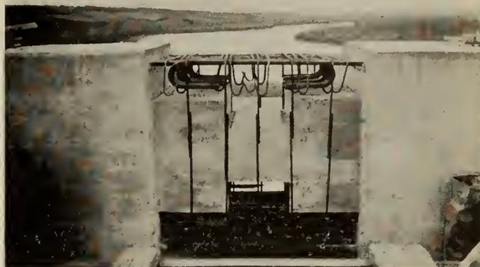
Fig. 11—Hinge, showing Main Rib Reinforcement.
