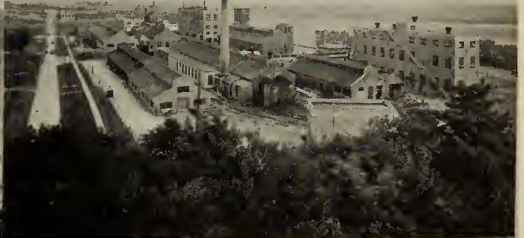
The plant of the North American Cyanamid Limited at Niagara Falls, Ont., is the largest cyanamid works in the world. The products manufactured are cyanamid, cyanide and silicate of soda. Cyanamid is used as a fertilizer and is made by absorbing nitrogen in powdered calcium carbide at white heat. The capacity of the plant is over 350,000 tons. Nearly 1000 people are employed.
