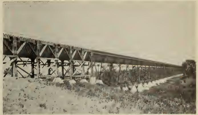
Fig. 14—Metal Flume on Timber Trestle at Oldman River Crossing.
