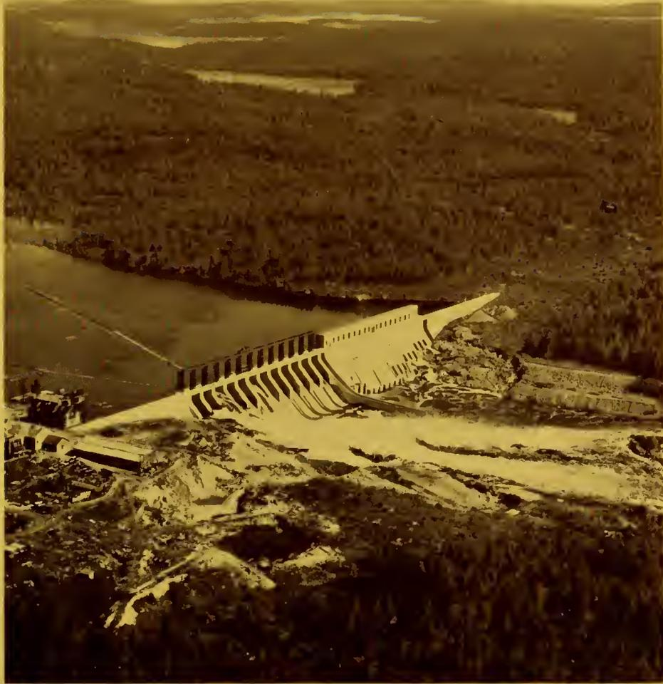
**A**ERIAL photograph of Mercier Storage Dam on the Gatineau River, Province of Quebec. This dam was constructed in 1926-27 by The Foundation Company of Canada Limited for the Quebec Streams Commission and the Gatineau Power Company. The building of this dam created one of the largest storage reservoirs in the world, its capacity being approximately one hundred billion cubic feet of water.
