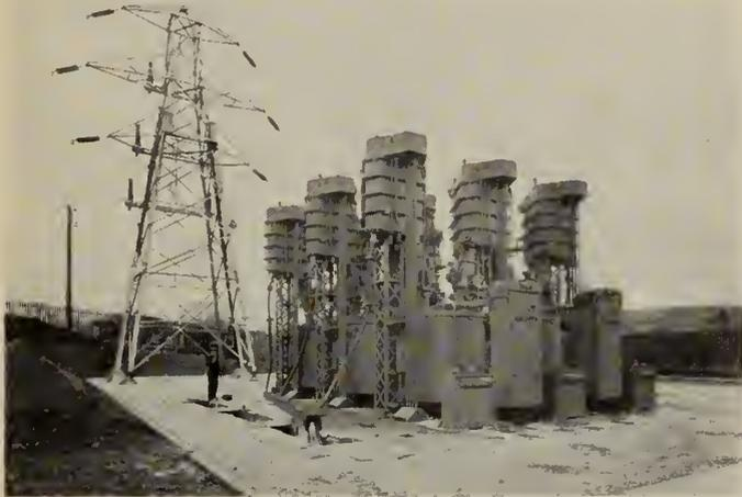
Fig. 9—Metal Clad 132-kv. Switchgear at Tongland.
