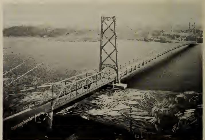
Fig. 28—St. Maurice River Suspension Bridge, Grand'Mère, Que. Twisted wire rope cables. Cables and stiffening trusses erected from the ice 1929.
