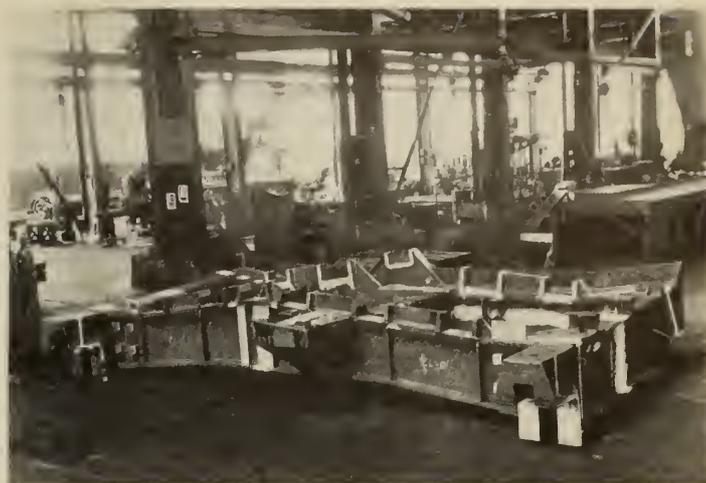
Fig. 3—Arc Welded 60-Ton Crane Trolley Frame.
