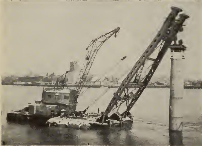
Fig. 9—Transporting Caisson from Drydock to Site, Saint John.
