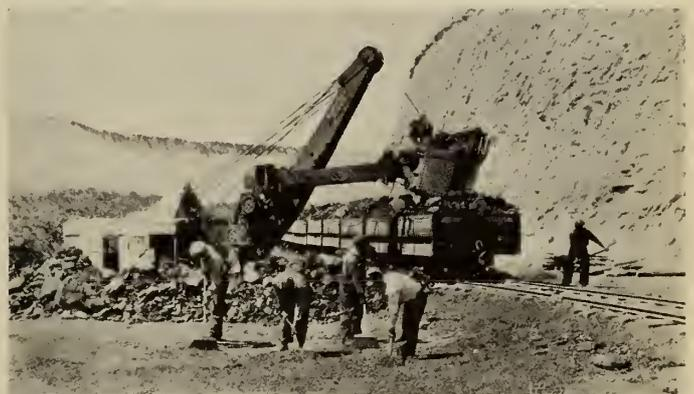
Fig. 5—Loading Lignite into 4-ton pit Cars at Opencast Mine.
