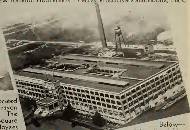
Buildings and grounds of Canadian Kodak Company, Ltd., Kodak Heights, Toronto. Floor space 500,000 square feet; employment 800. The power plant has latest equipment, automatically controlled; will develop 1800 h.p.; operates at steam pressure of 450 lbs. and steam temperature of 560° F. A 750 kw. turbo-generator, speed 8,000 r.p.m., supplies electrical power.
