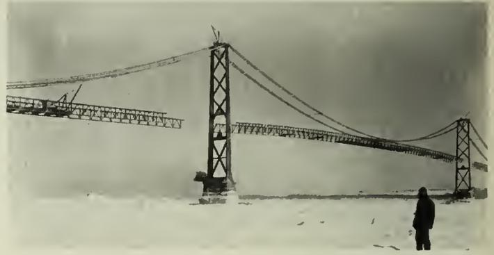
Fig. 7—Erection of Stiffening Trusses.
