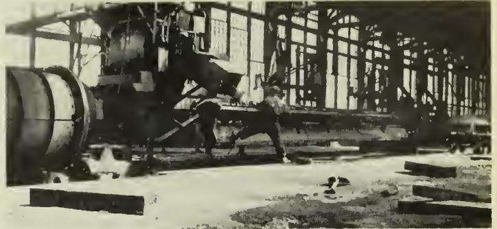
Fig. 17—Concrete Mixing, Loading and Spinning Equipment.
