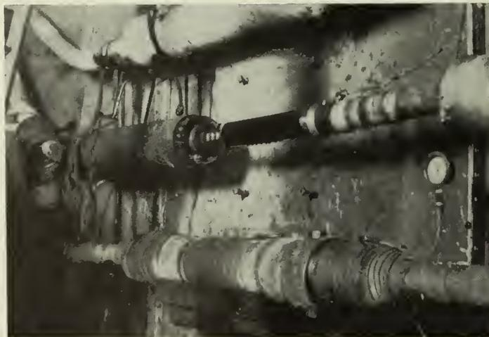
Fig. 5—Stop Joint Being Assembled.
