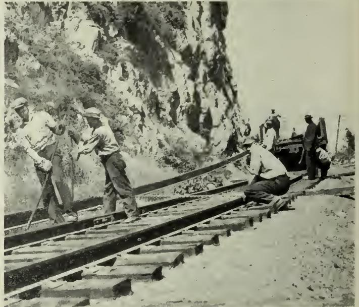
Fig. 3—Distributing Welded Rail Beside Curved Track.
