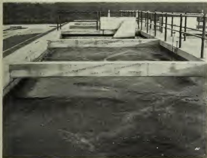
Fig. 3—Aeration Tank in Activated Sludge Plant.
