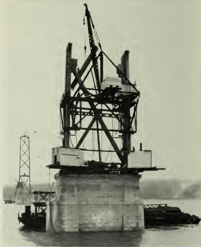
Fig. 5—Creeper Traveller Erecting Tower.
