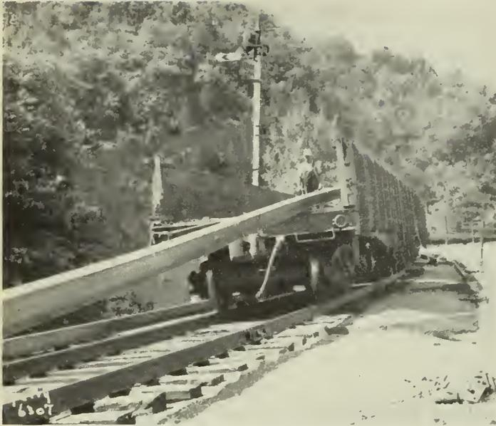
Fig. 1—Unloading Welded Rail.
