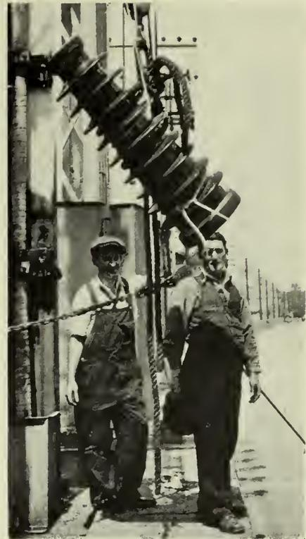
Fig. 8—Porcelain Bushing Being Hoisted into Place.
