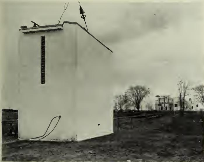
Fig. 3—Tuning House. Co-axial Feed Line, Rear of Transmitter Building and Substation.
