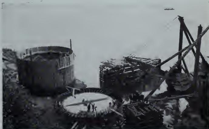
Fig. 5—South main pier: caisson-construction on shore.
