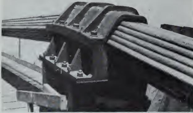
Fig. 66—Saddle at south cable-post.
