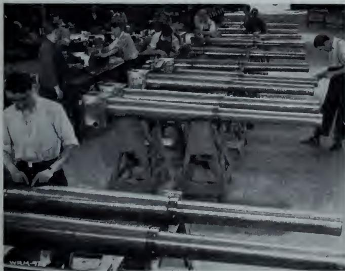
Fig. 5—Fitting breech mechanisms to gun barrels.
