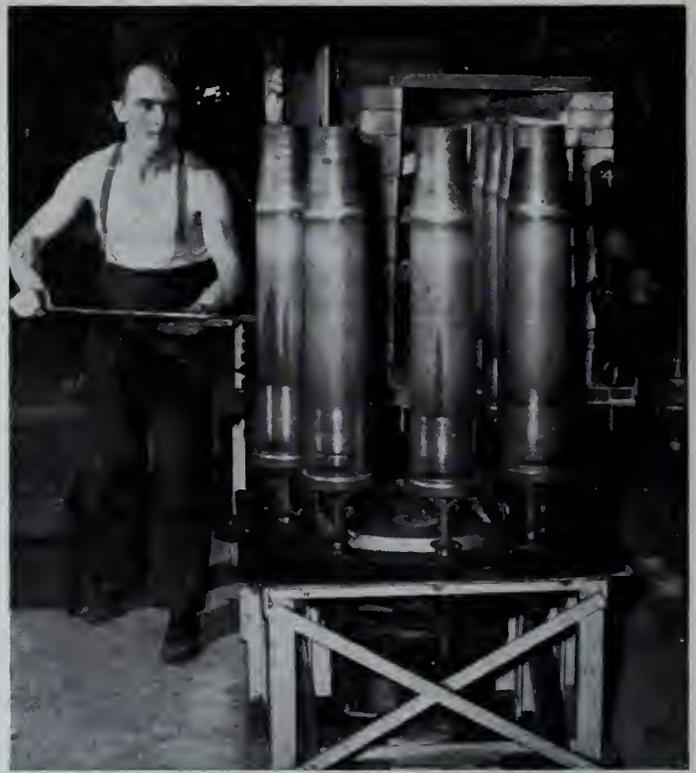
Fig. 11—Mouth annealing 4-inch cartridge case after necking.
