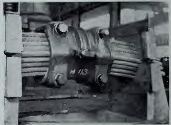
Fig. 45—Assembly of cable-band.
