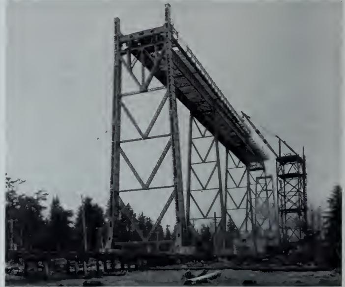
Fig. 55—Erection of north viaduct.
