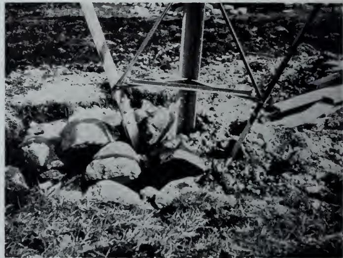
Fig. 2—Anchoring a grillage in soft ground by backfilling with rock.
