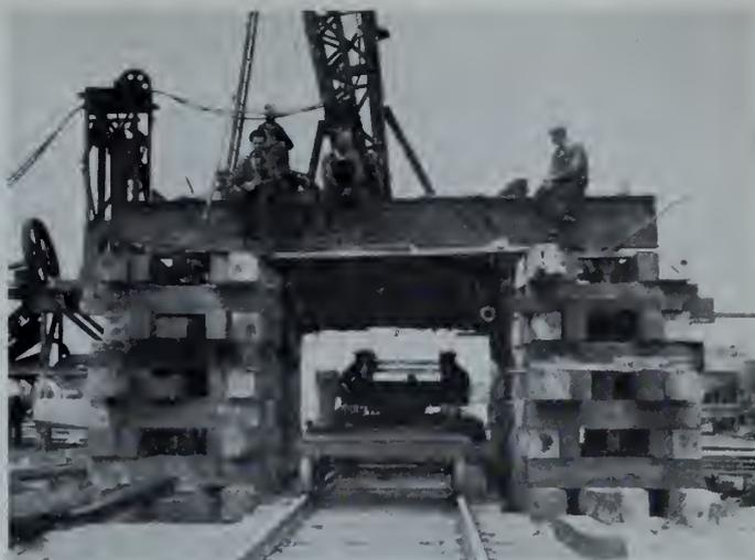
Fig. 5—Jacking crib at shear leg end showing 60-ton trucks being placed under leg.
