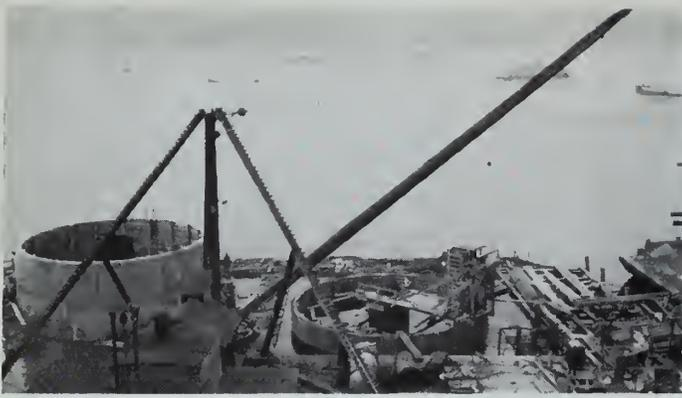
Fig. 6—South main pier: sinking of caissons.
