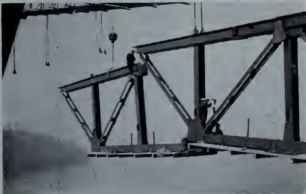
Fig. 64—Erection of truss-section, north side-span.
