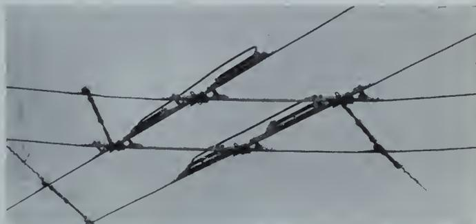
Fig. 6—Typical crossover using standard insulating unit tips and crossover pan.
