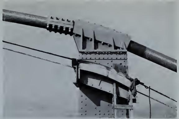
Fig. 65—Cable-saddle and keeper at cable-bent.
