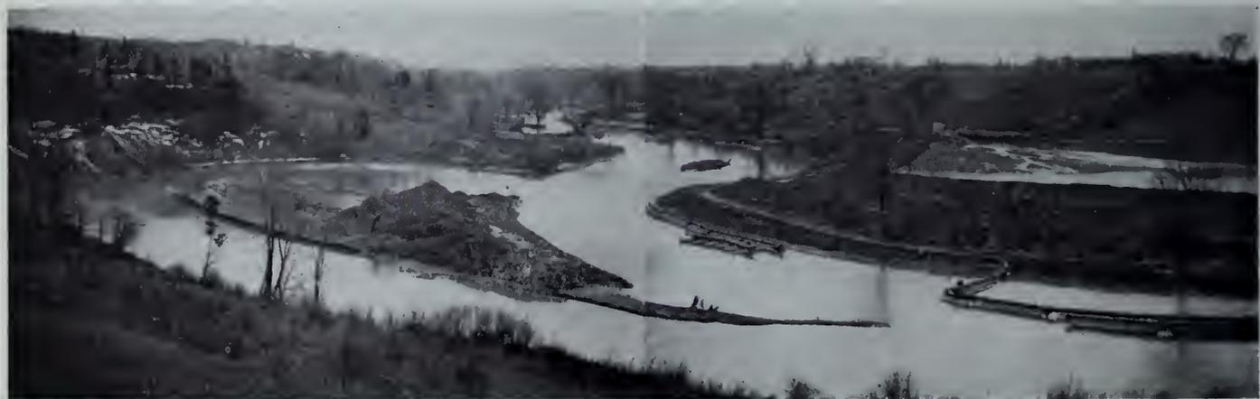
Fig. 10—Photographs of enlarged channel in Twelve Mile creek. Original channel at left, disposal area at right.
