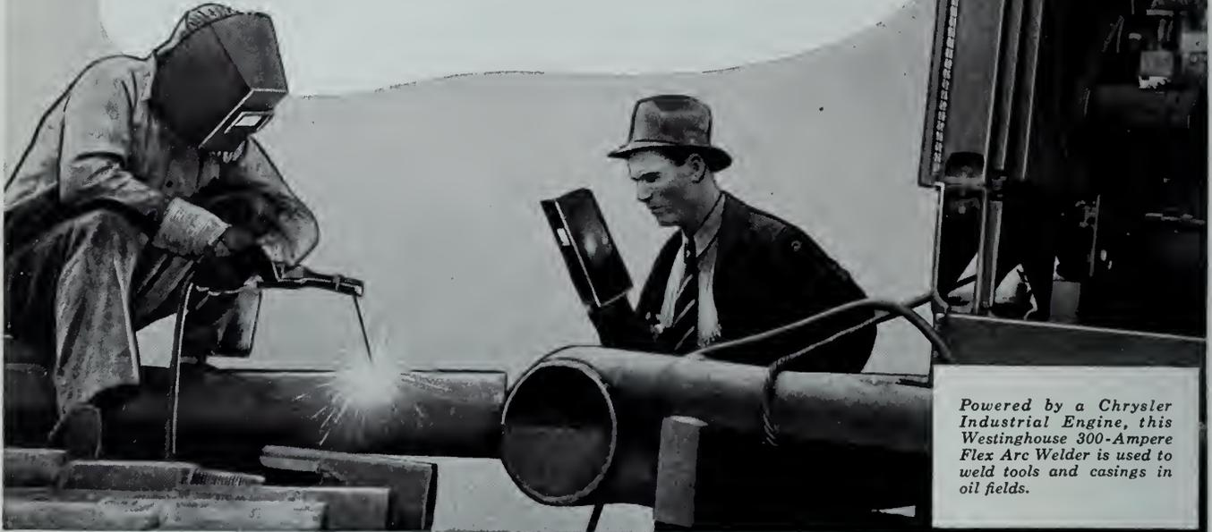
Powered by a Chrysler Industrial Engine, this Westinghouse 300-Ampere Flex Arc Welder is used to weld tools and casings in oil fields.
