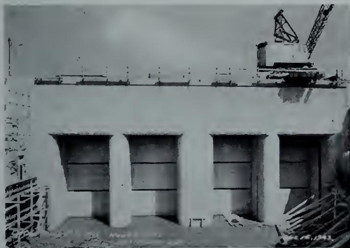
Fig. 6—Photograph of headworks nearing completion.
