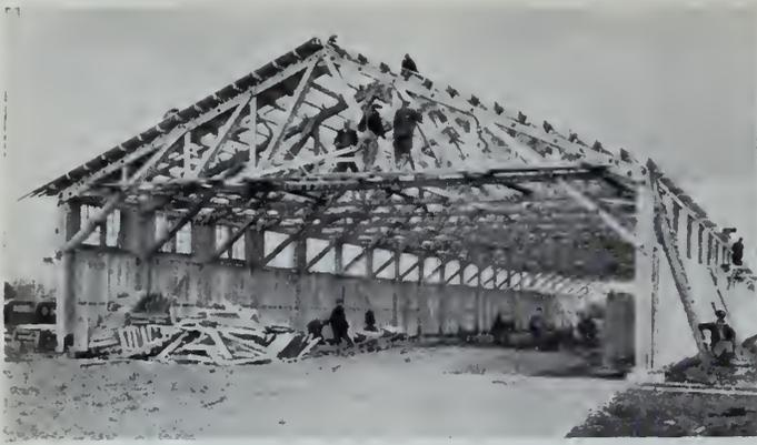
Fig. 16—51 ft. span triangular Pratt trusses which support a roof over a storage building for Fairchild Aircraft Ltd., near Montreal.
