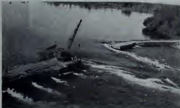
Closing the gap in the final stage of Coteau Dam No. 3 cofferdam.
