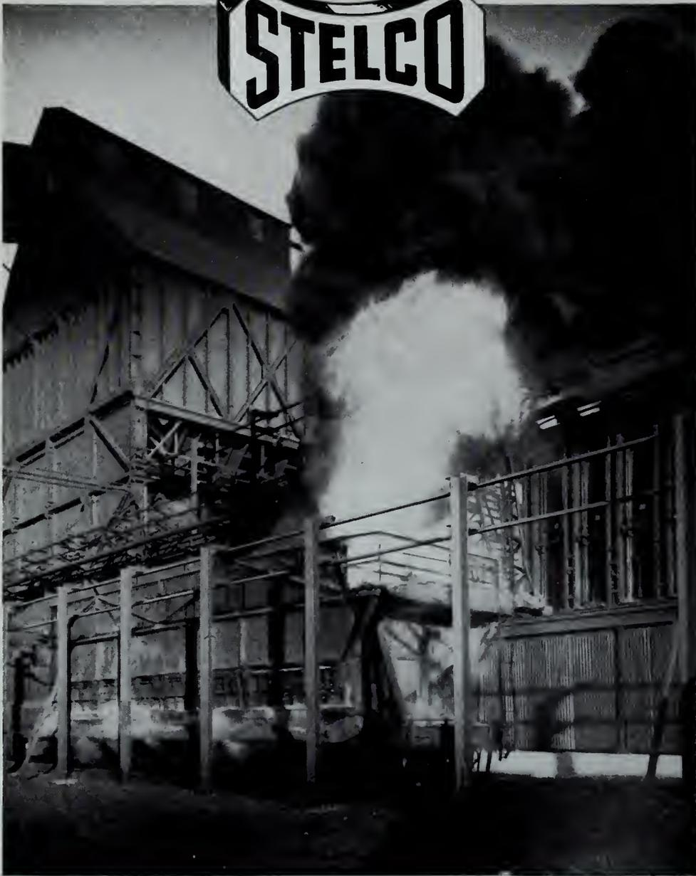
*Flame and smoke burst forth as another carload of Stelco Blast Furnace Coke leaves the oven.*
