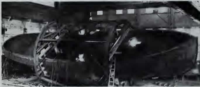
Fig. 2—Positioner for all-welded ship, allowing downhand welding.
