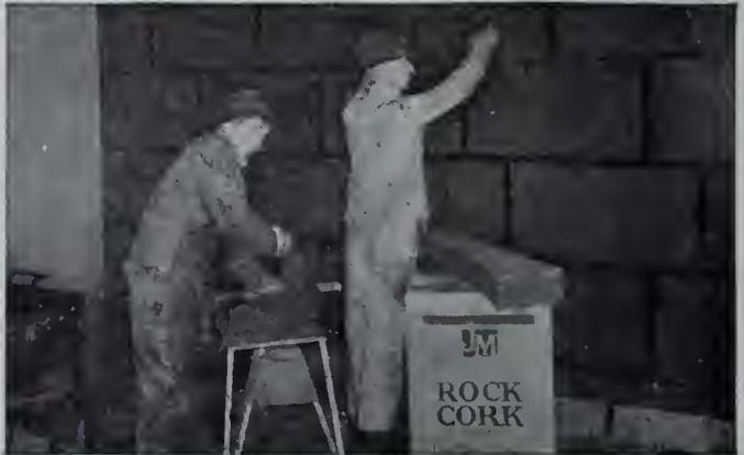
**LOW TEMPERATURES . . .** J-M Rock Cork Sheets and Pipe Insulation are recommended for cold storage construction and refrigerating equipment. J-M Rock Cork does not rot or decay. Unusually moisture-resistant, it assures permanently high insulating efficiency.
