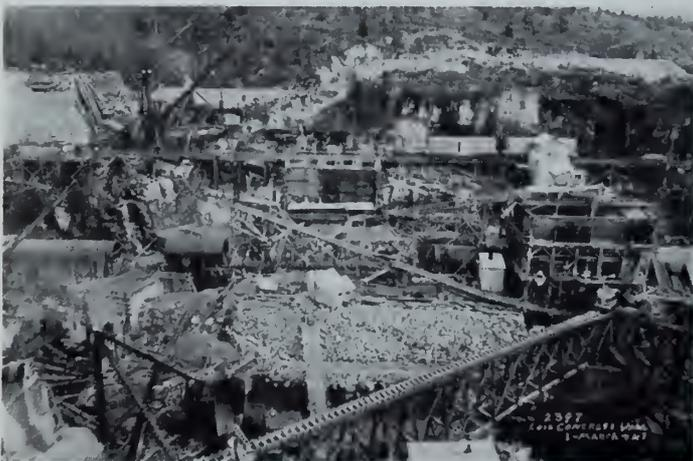
Fig. 5—General view of construction works showing mixing plant, narrow-gauge tracks, etc.
