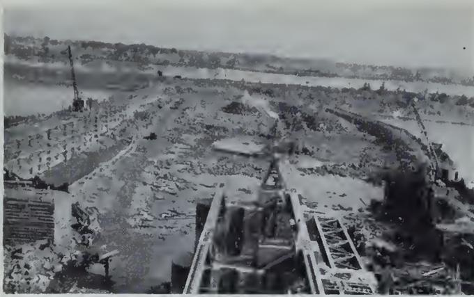
North channel at Ile Juillet unwatered in one large cofferdam.
