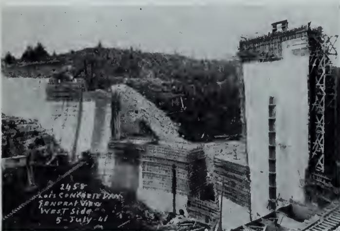
Fig. 3—General view of west side of dam showing entry gate section, culvert, and method of pouring successive sections.
