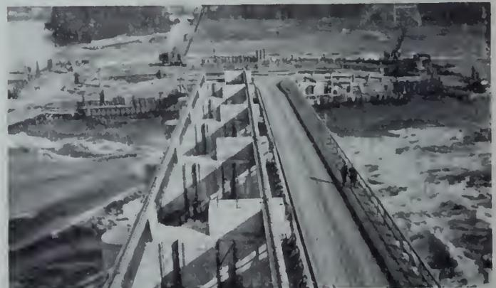
Construction of Dam No. 3 at Coteau (1943), showing first stage completed and opened, the second cofferdam unwatered, and the third section of the channel still flowing free.
