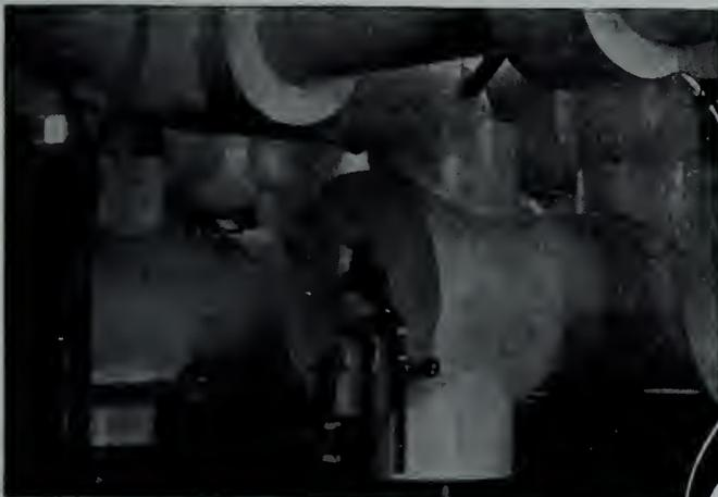
**IN BLOCK FORM . . .** J-M 85% Magnesia Blocks are furnished 3"x 18", 6"x 36", 12"x 36", in thicknesses of 1" to 4". Weight, about 1.4 lb. per sq. ft., per 1" thick.
