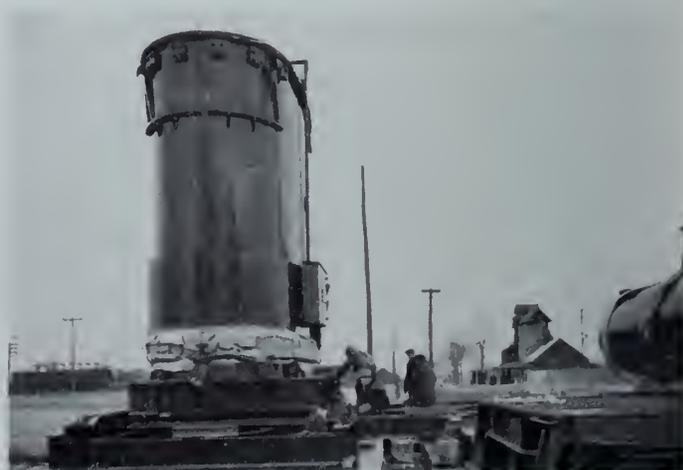
Fig. 3—Transformer on transfer truck.
