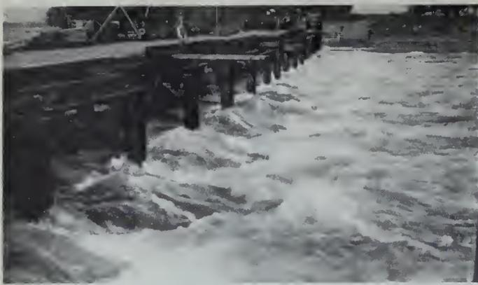
Steel cribs all placed across south channel at Ile Juillet with 20,000 cu. ft. per sec. flowing through open cribs prior to filling with rock.
