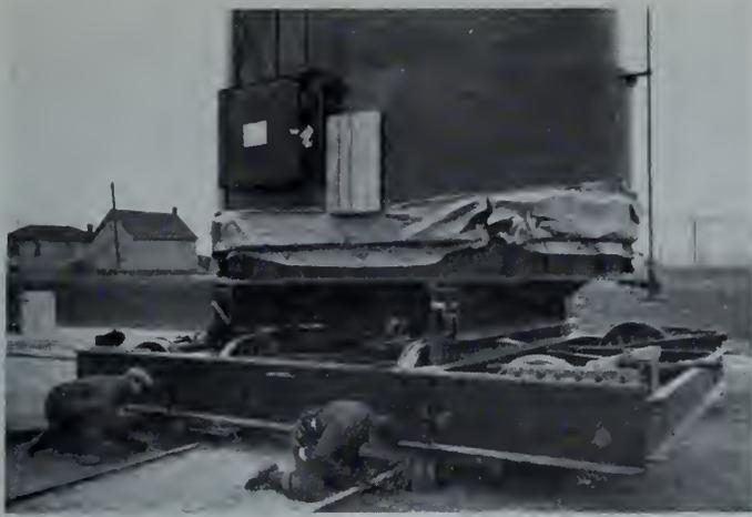
Fig. 4—Changing wheels on transformer truck.
