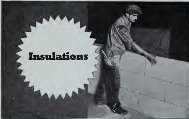
**BOILER FURNACES . . .** Johns-Manville Superex is the most widely used block insulation for temperatures between 600° and 1900° Fahrenheit. Low thermal conductivity means less thickness required than with any other material of equal heat resistance.
