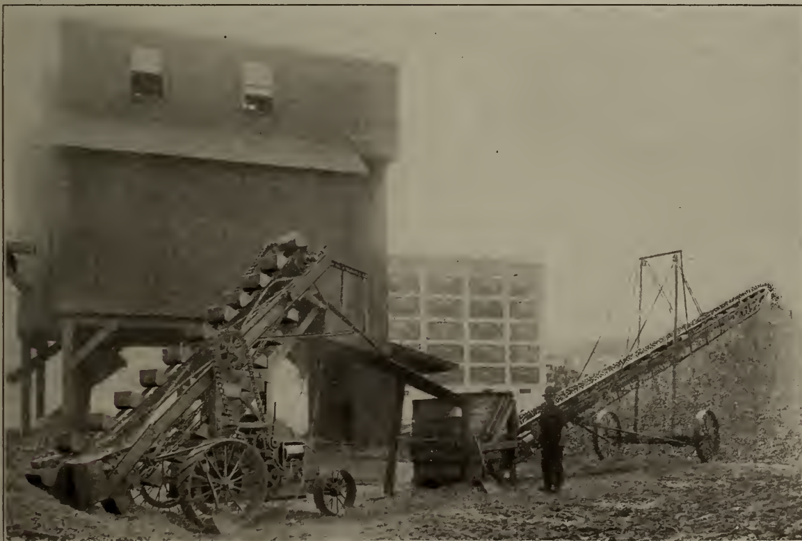
Old Type B. G. Bucket Loader handling Coal from Stock Pile and delivering to B. G. Portable Belt Conveyor.
