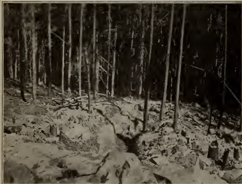
Trench across norite 'orebody' on the 'Hititrite' claim. The 'orebody' is here a mineralized zone 150 feet wide, along the norite-greenstone contact. Muskeg in the background.
