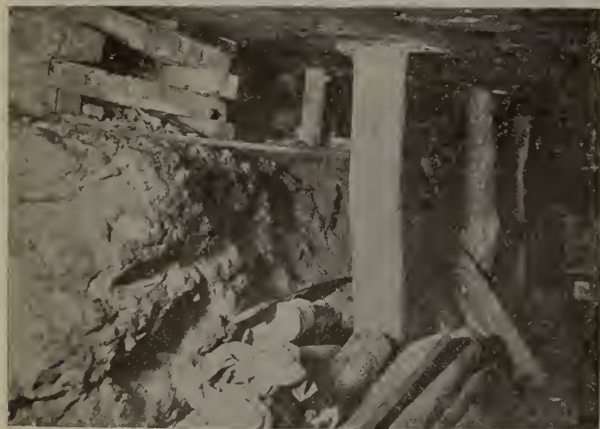
WOODEN CRIBS USED IN LONGWALL MINING IN THIN SEAM OF ANTHRACITE.
