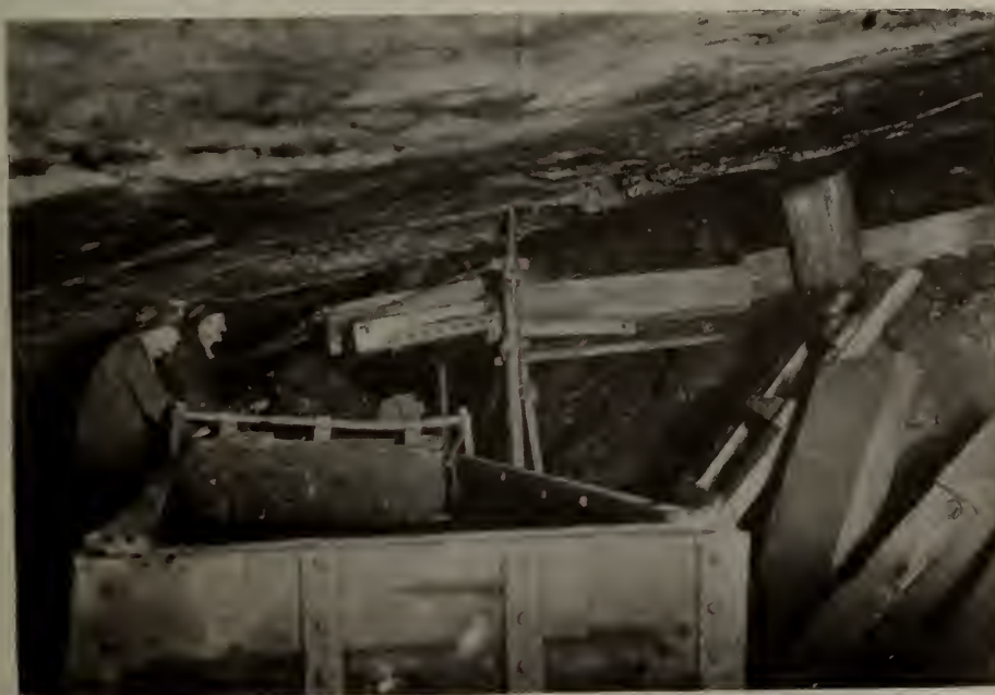
LOADING FROM A LONGWALL FACE. NOTE AGAIN THE THINNESS OF THE SEAM.
