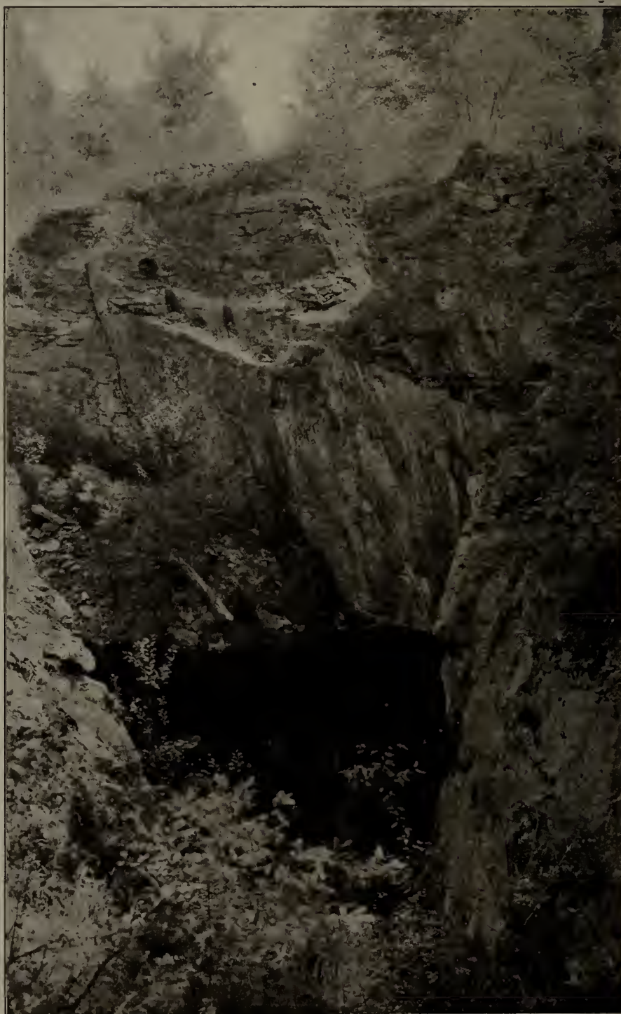
Main pit of Miller mine, range V, lot 10, township of Grenville, Que. The ore-body is stated to have followed the well defined slip face on the far side of the pit
