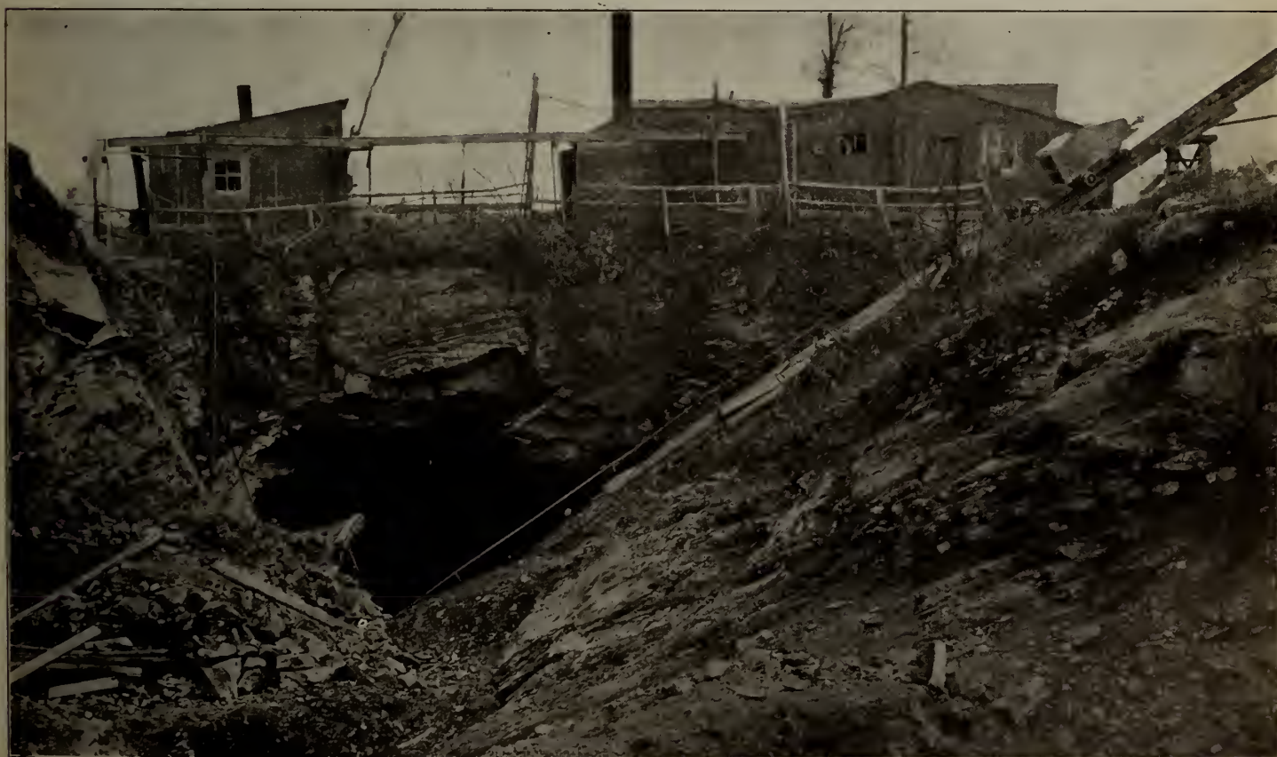
Open cut above workings of Globe Graphite Mining and Refining Company, concession V1, lot 21, township of North Elmsley, Ont. The banding in the limestone is well shown, and a well defined fold is exhibited in the cap rock above the shaft. Graphite bodies tend to occur at the crest of such folds.
