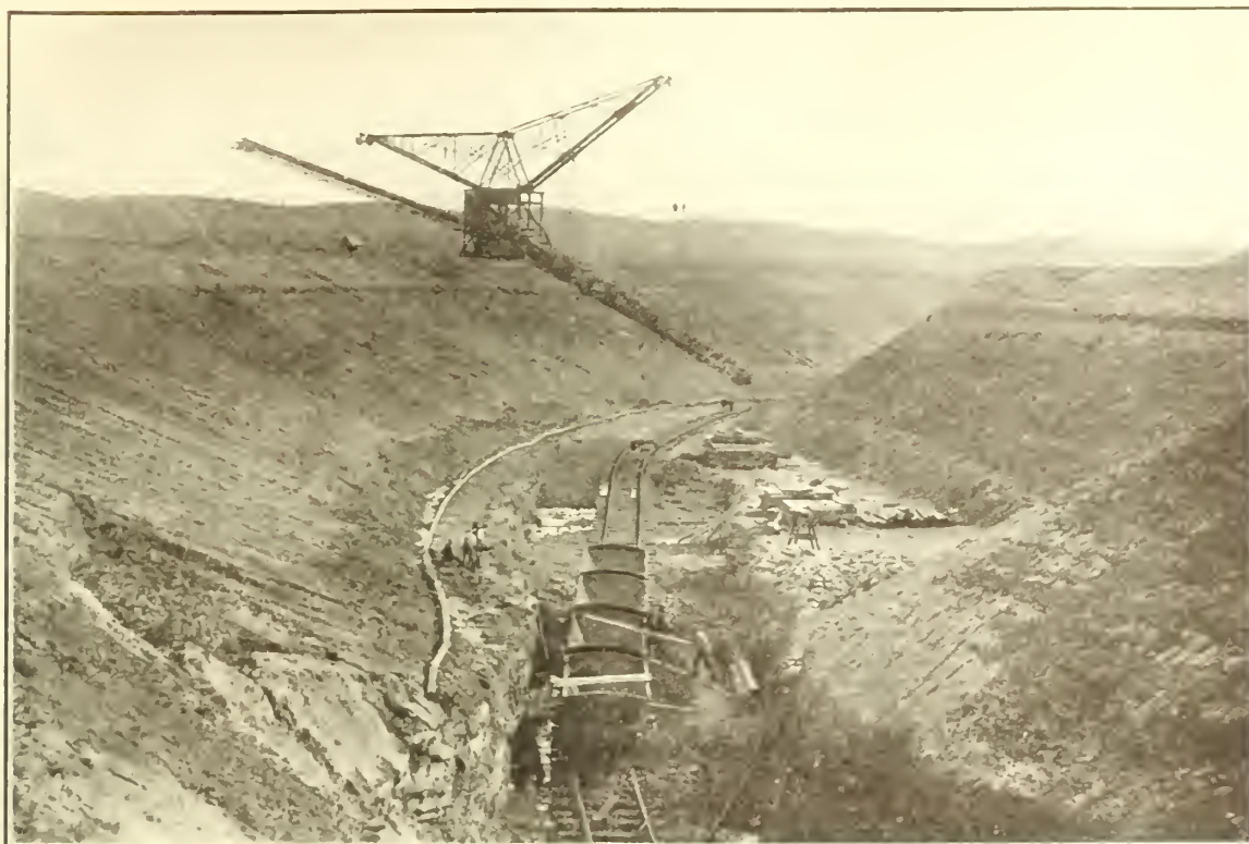
Stripping Operations—Frodingham Iron-Ore Bed.
