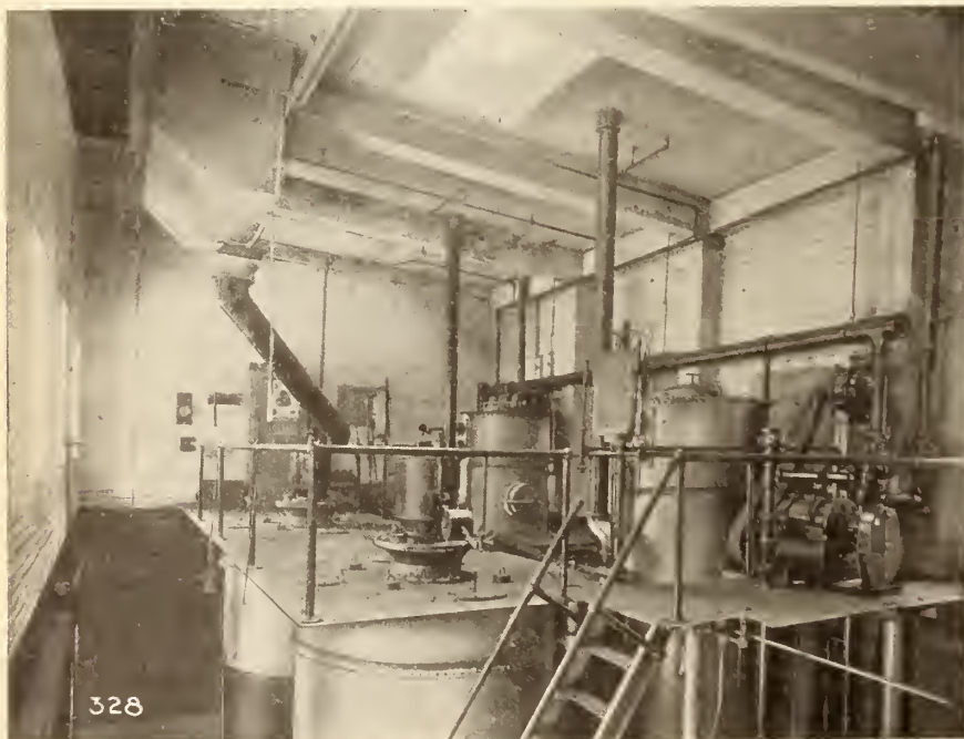
Operating platform of two 100 h.p. type "A" Akerlund Gas-Producers in use for several years at the plant of the Simonds Saw Company Montreal.
