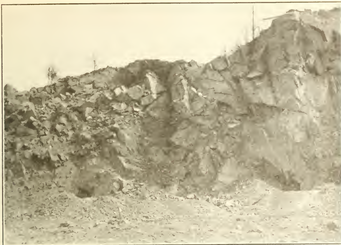
Ontario Rock Company's Preveaux Quarry, showing 60 foot face and entrances of Blasting Adits.
