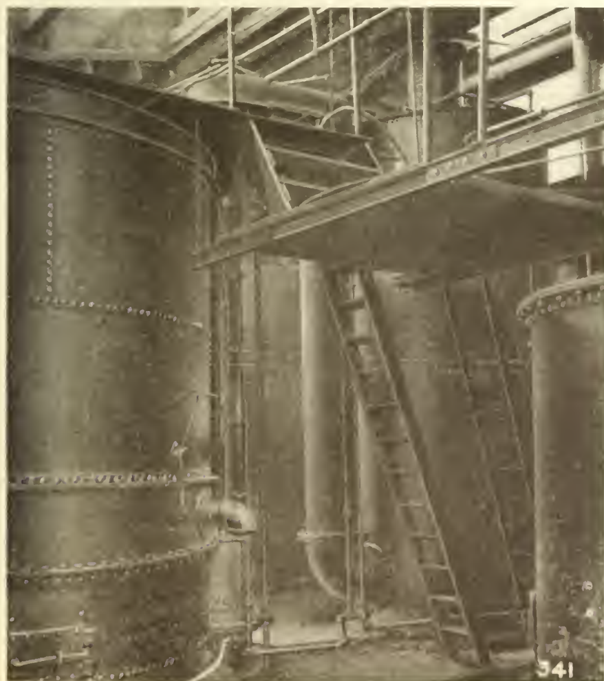
500 h.p. type "B" producer-gas plant for municipal electric-lighting and power. Suitable for utilization of lignite.
