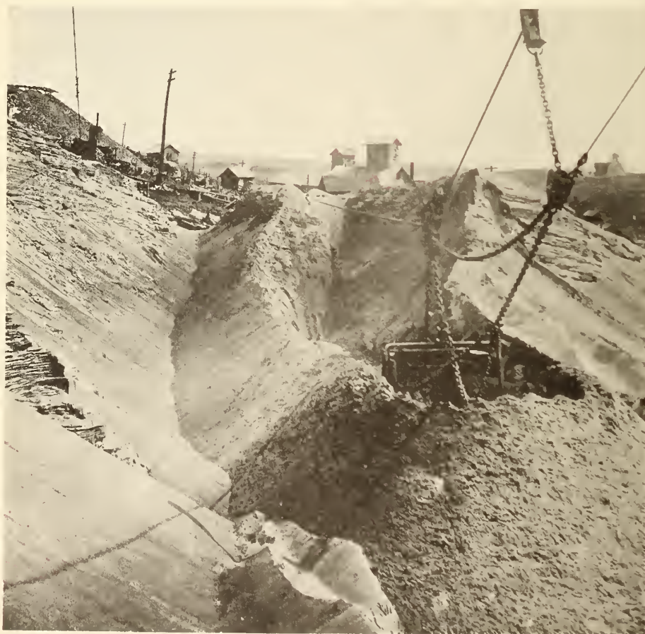
Sauerman drag-line excavator at Coniagas Mine reclaiming sands carrying 3 to 3½ ozs. of silver per ton. The sand is re-ground in tube mills to 100-mesh and treated by the flotation process.
