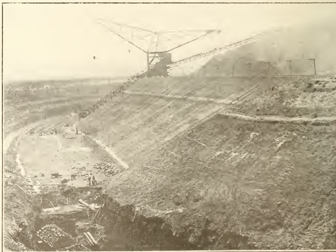
Stripping the Frodingham Iron-Ore Bed.
