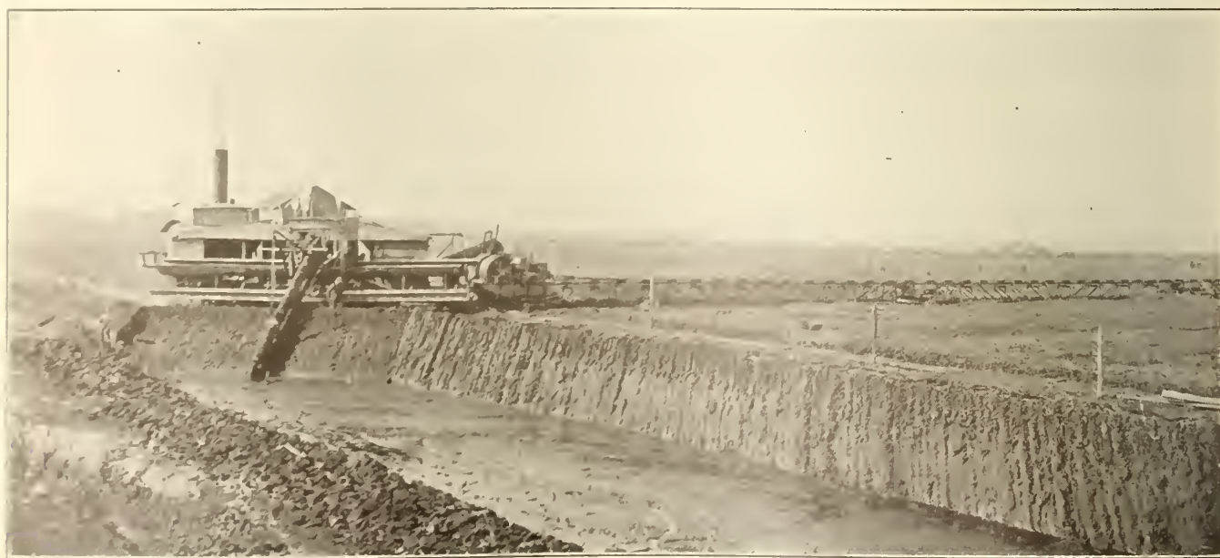
Anrep-Moore Peat Machine, showing Excavator, with Digger working on diagonal face, and part of Belt Conveyor.
