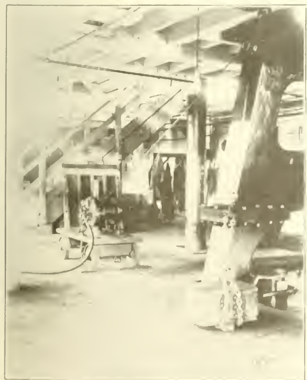
Fig. 7. — Changing stamp mill shoes with a column hoist mounted on a small truck.
