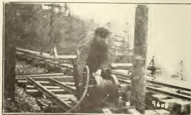
Fig. 6. — Hauling Rails through a rail bender with a Little Tugger Hoist.
