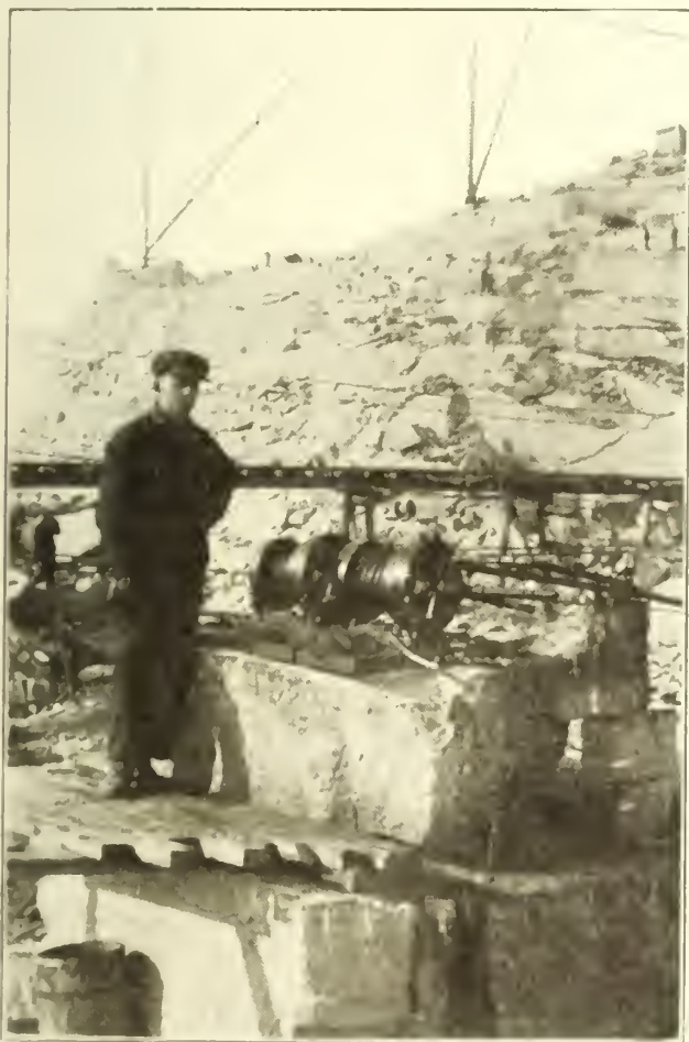
Fig. 9. — Two Hoists of the Little Tugger Type used for swinging a large derrick.
