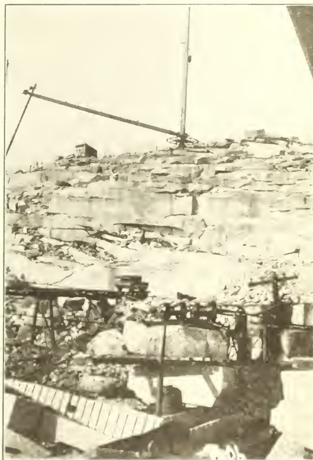
Fig. 10. — Tugger Hoists used for hoisting supplies and carrying derrick cable across quarry.
