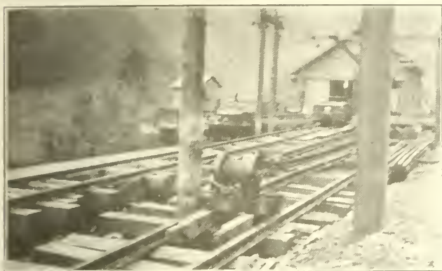
Fig. 6a. — Hoist arranged for hauling rails through bender.
