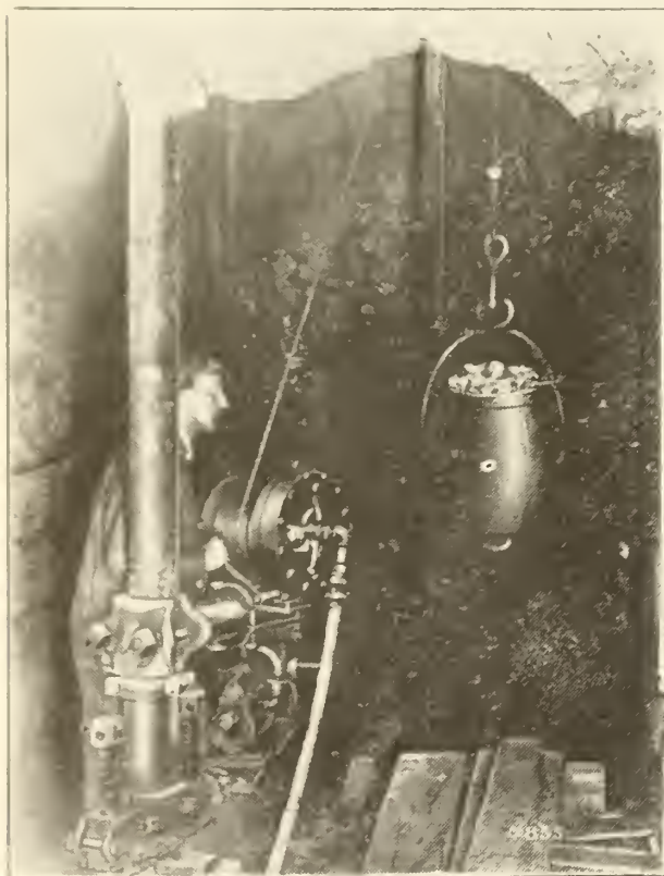
Fig. 4. — Hoisting muck in a winze with hoist clamped to stretcher bar.
