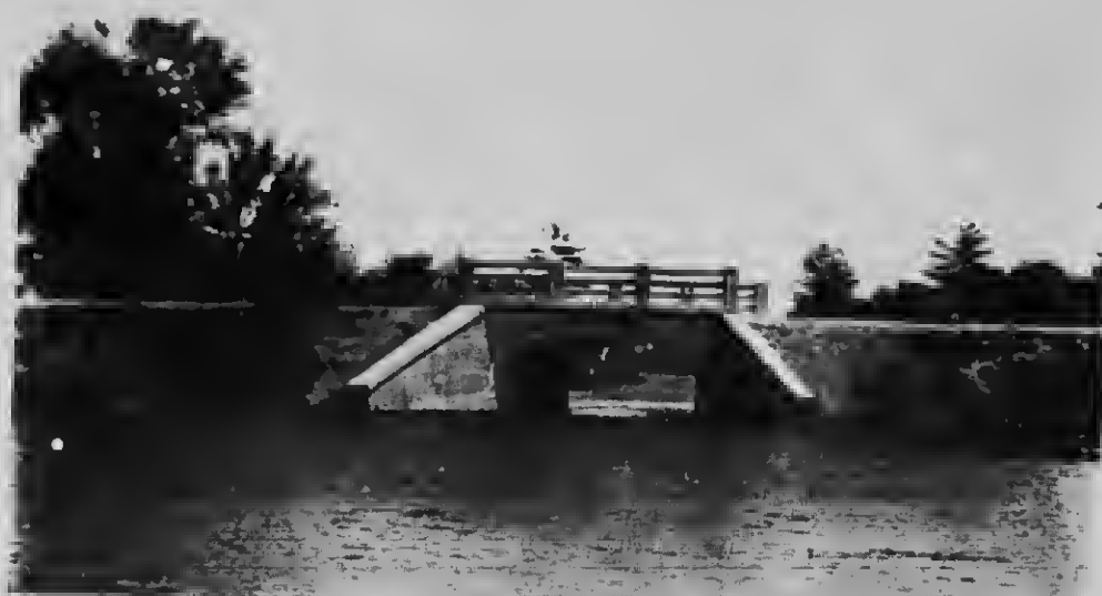
Patterson Creek Bridge, Ottawa.
