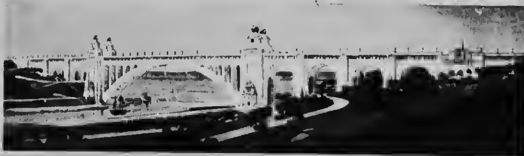
Perspective view of proposed Henry Hudson Memorial Concrete Arch Bridge, as it will appear when completed. It will have a single arch span 703 feet in the clear and a rise of 177 feet centre to centre, or approximately three times as long as the longest Concrete Arch Bridge now in existence.
