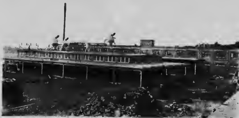
Partial View W. C. Edwards' Mill, Ottawa.
