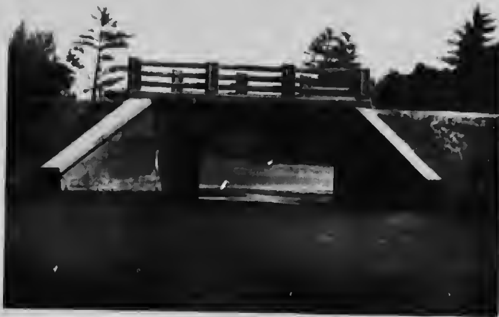
Peterson Creek Bridge, Ottawa.
