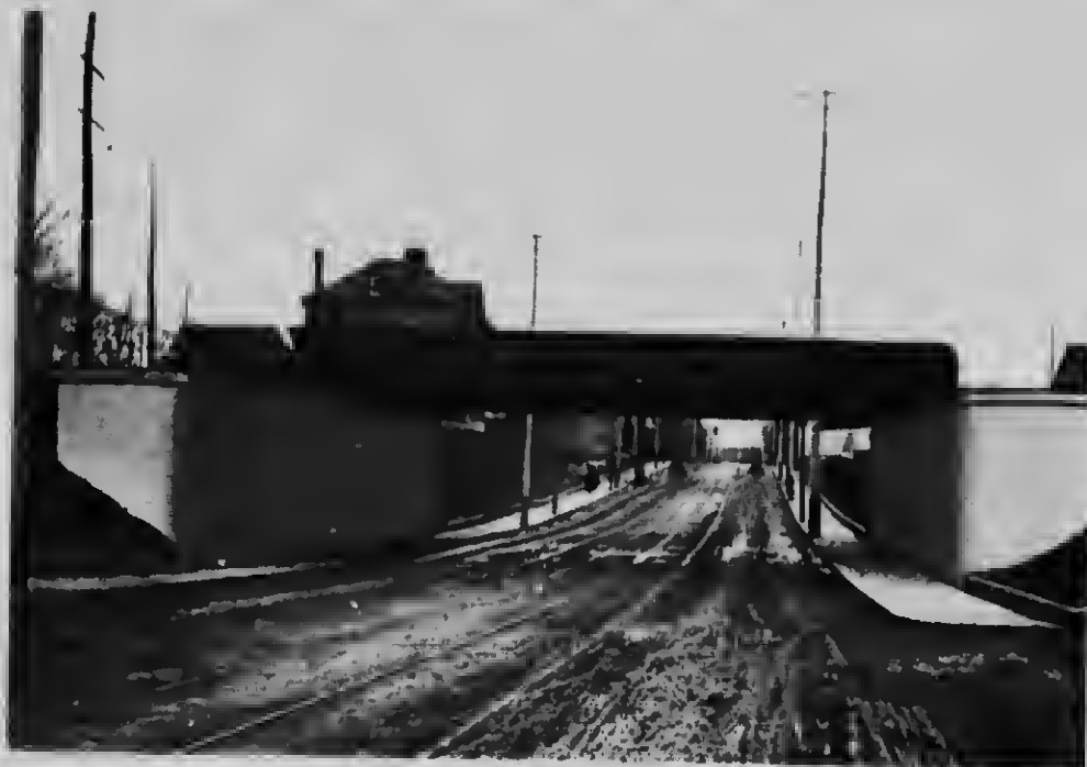
Grand Trunk Bank St. Subway Ottawa.
